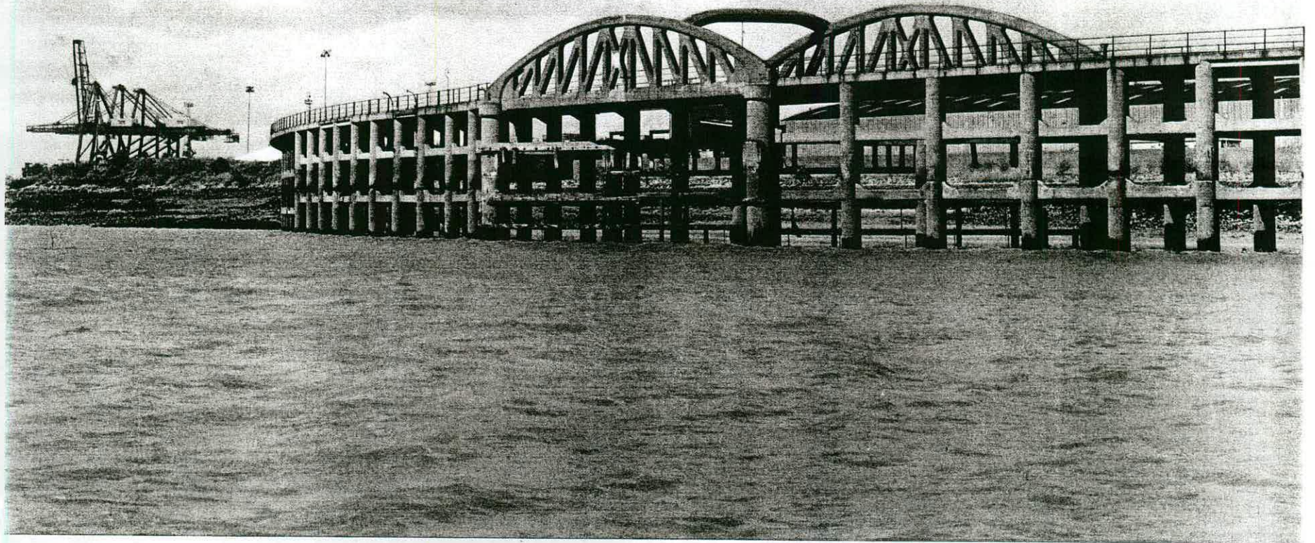
28 - RIVER CARGO JETTY, PORT OF TILBURY, ESSEX - Construction of this 1000ft long cargo jetty for the PLA was started in 1913, although it wasn't completed until 1921 due to the war. It is built of reinforced concrete, a notable and early use of the material, with the deck supported on cylindrical columns. The purpose of its construction was to allow larger ships to save time by not having to lock in and out of the main dock. Railway tracks were built on the deck of the jetty to facilitate the distribution of goods. Unfortunately, due to the large tidal rise and fall, the jetty has never proved popular. (AA94/3489)
