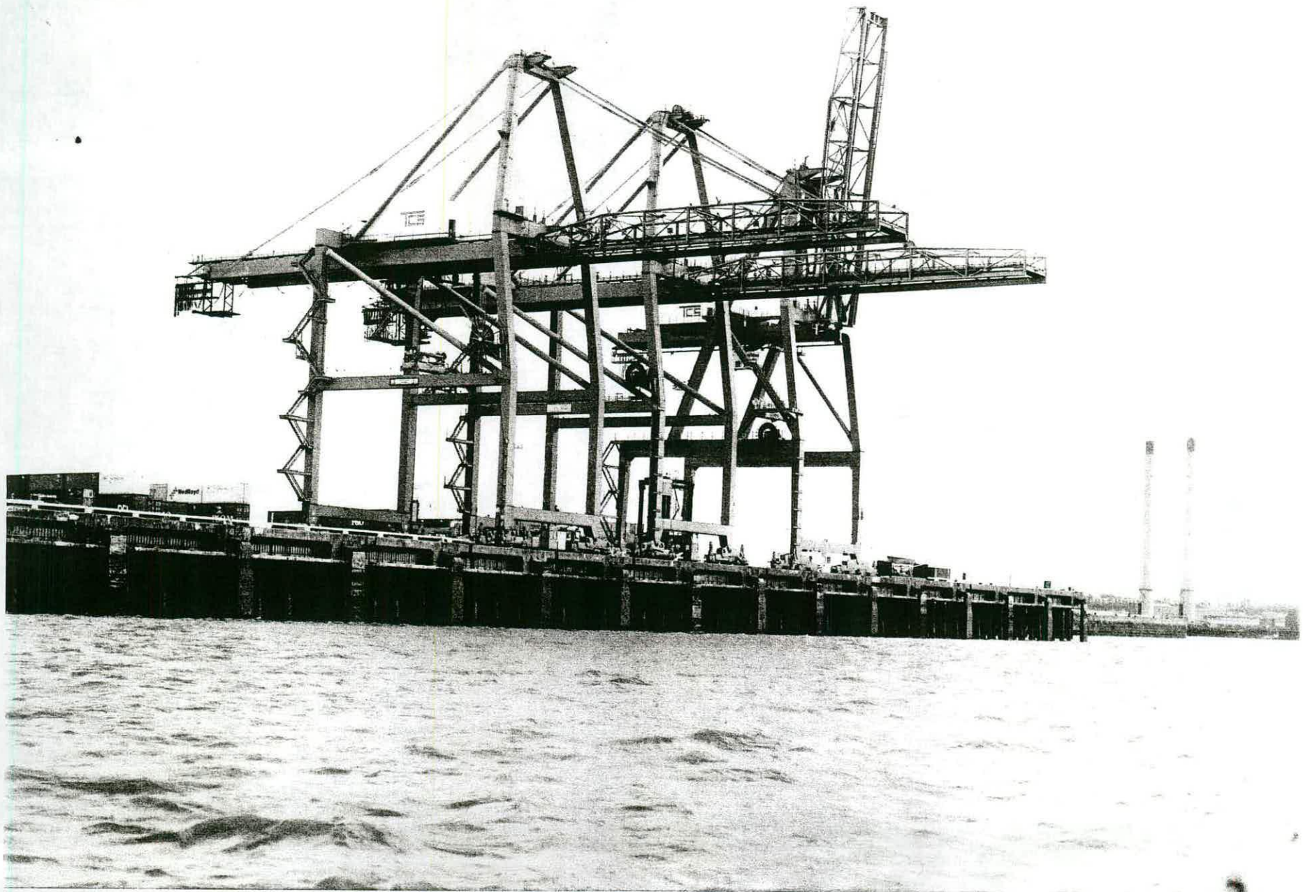
26 - NORTHFLEET HOPE TERMINAL, PORT OF TILBURY, ESSEX - This container handling berth was built 1976-8 when 25 acres of river front at Northfleet Hope was reclaimed for its construction. The container terminal it serves was established c.1965 and covers some 64 acres, stretching back from the river front to the west side of the branch dock extension of Tilbury Docks. The three riverside single lift cranes shown here can each carry 35 tonne containers. The chimneys of Northfleet Power station can be seen in the distance. (AA94/3496)
