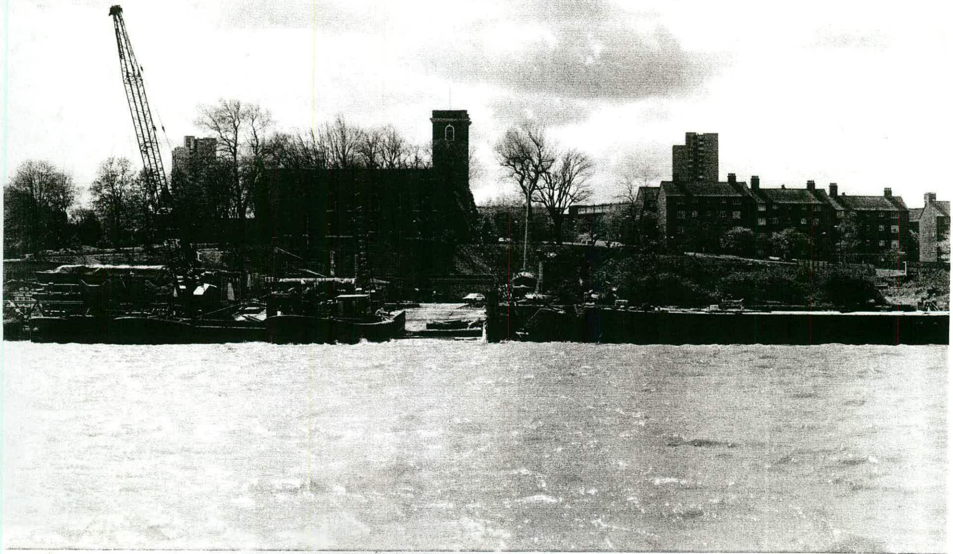
48 - SHIP BUILDING SLIPS AND THE CHURCH OF ST MARY, WOOLWICH, L.B. GREENWICH - Two slipways at the east end of the former Woolwich Royal Naval Dockyard continued in use for shipbuilding into the 1980s as Cubow's Shipyard. They remain a repair facility. Downstream is the site known as Mast Pond Wharf, reflecting its use when the site was part of the Royal Dockyard. The simple brick Church of St Mary Magdalene on the hill to the south was built in 1727-39 by Matthew Spray. (AA94/3353)
