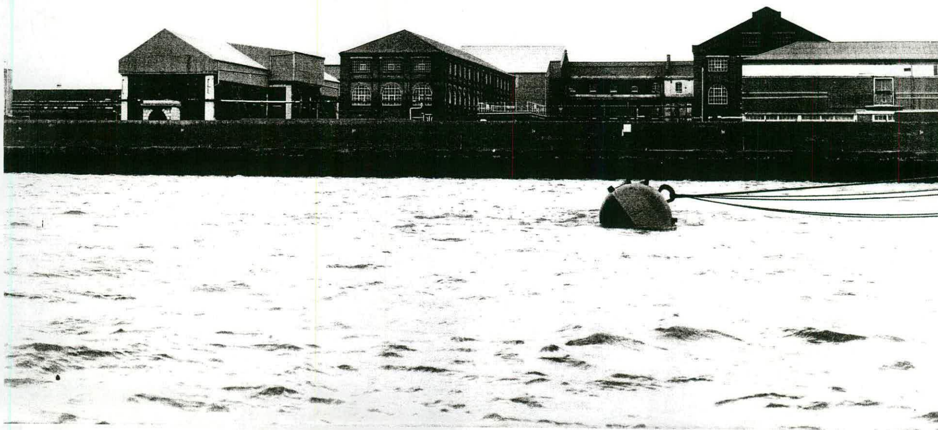
51 - THE GRAND STORE, WOOLWICH ARSENAL, L.B. GREENWICH - This imposing complex of storehouses was built by the Board of Ordnance for the Royal Arsenal from 1806 to 1813. It is one of the most important and least altered of the few surviving groups of warehouse buildings from a period notable in England for its ambitious commercial and military architecture. An open yard towards the river for the storage of shot was partially infilled in 1889-90 with more warehouse buildings. Much of the early complex has been out of use for many years and survives in poor condition. (AA94/3363)
