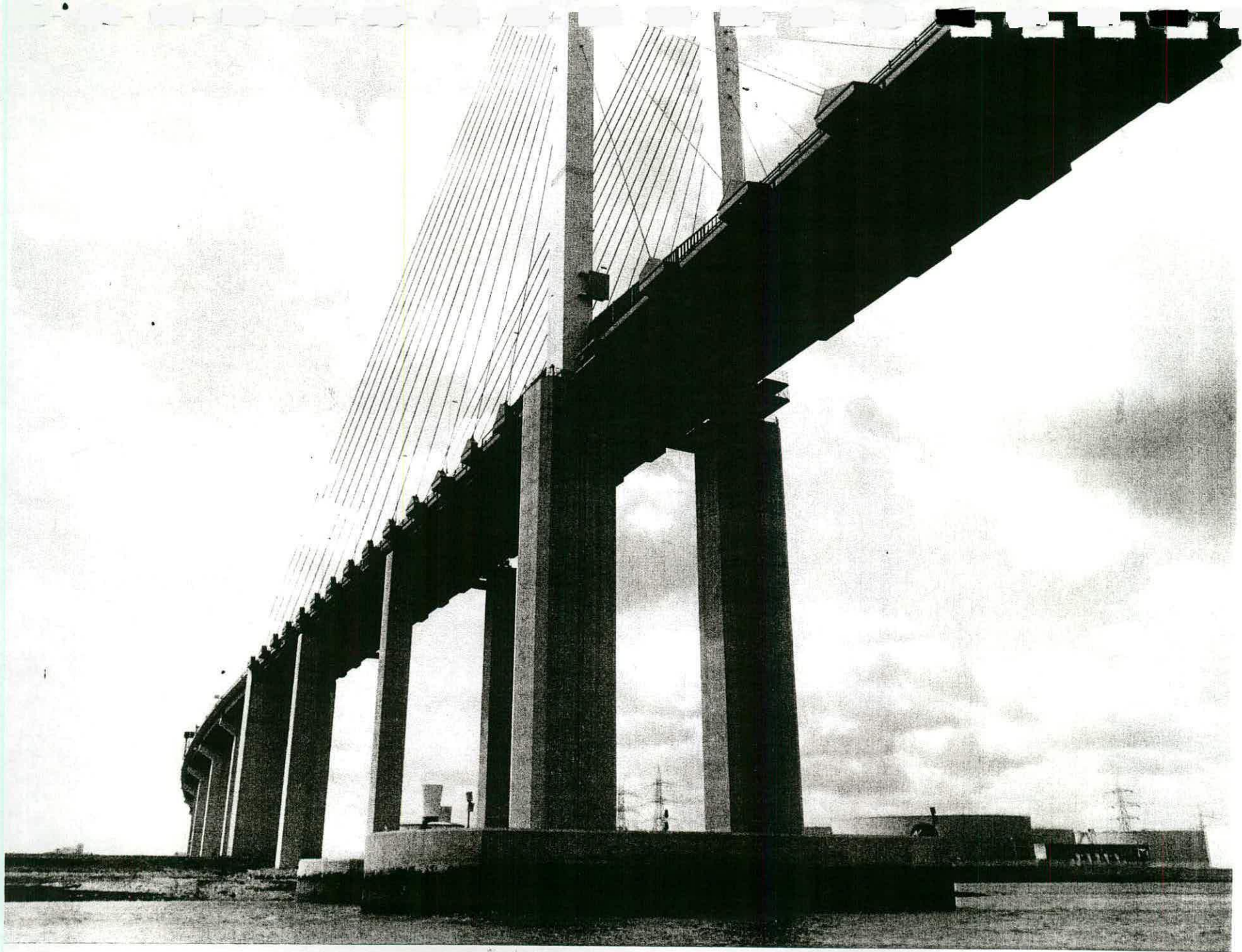
59 - QUEEN ELIZABETH II BRIDGE, DARTFORD, KENT - Opened in 1991 this impressive suspension bridge is the first bridge over the Thames to be put up downstream of London Bridge since Tower Bridge in 1894. It was built to relieve congestion at the Dartford Tunnel and carries southbound traffic on the A282 link in the M25 London orbital motorway. The masts rise 137m above the deck and its 450m river span was briefly the longest cable-stayed span in Europe. The bridge was designed by Trafalgar House Technology and constructed by the Cleveland Bridge Company. On the bank the oil tanks to Littlebrook Power Station are visible. (AA94/3409)
