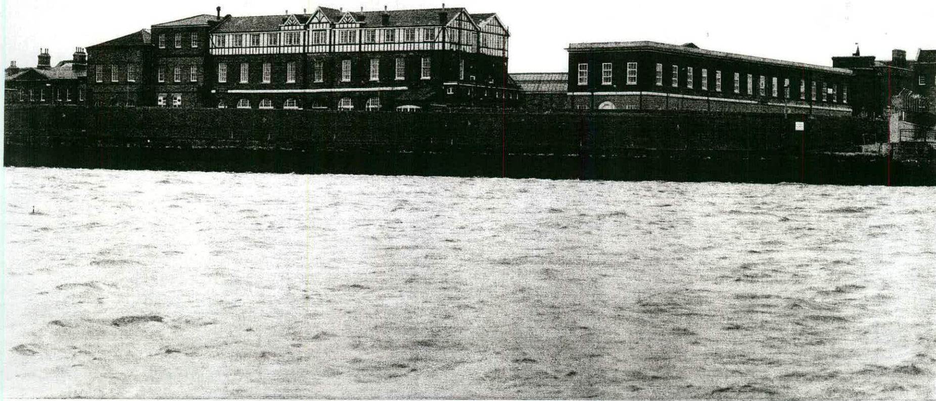
50 - THE ROYAL ARSENAL, WOOLWICH, L.B. GREENWICH - An ordnance depôt was formed at Woolwich in 1518, moving downriver onto what was then known as Woolwich Warren in 1671. The depôt was also used as a munitions factory from 1696 with the formation of the Royal Laboratory. In 1805 the growing establishment was named the Royal Arsenal and as such remained in use as a defence facility until 1994. Here, at the west end towards the river, is a view of part of New Laboratory Square, laid out during the Napoleonic Wars as an extension of the ammunition-making facilities of the Royal Laboratory. The mock-Tudor attic is a bafflingly whimsical early-20th-century addition. (AA94/3358)
