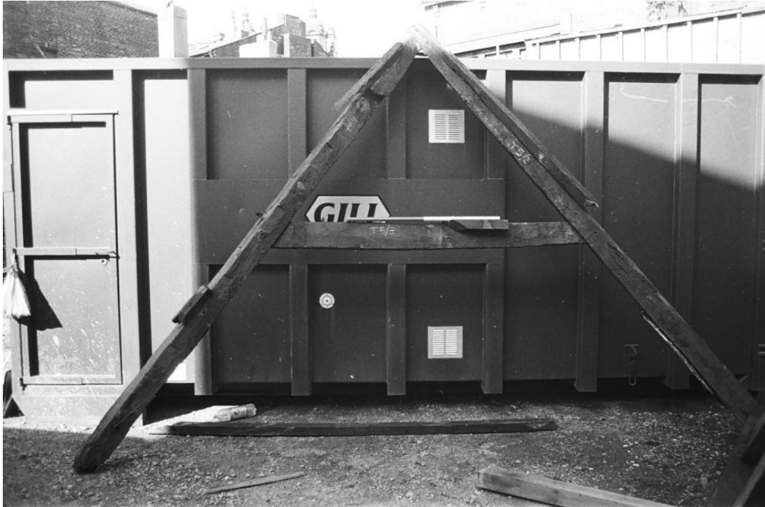
Figure 7: Truss 5 following salvage during demolition (photograph CFA Archaeology Ltd)
