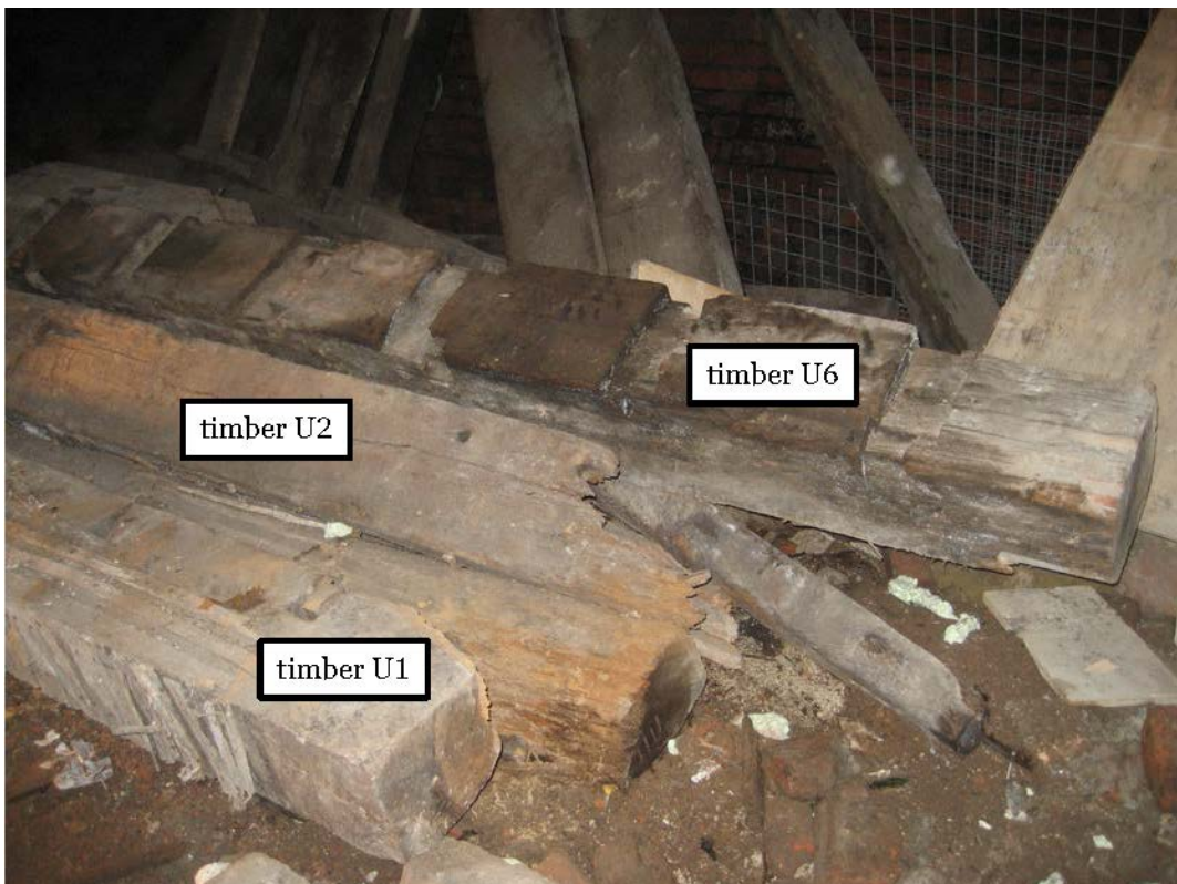
Figure 15: Annotated photograph showing some of the sampled loose timbers (photograph Robert Howard)
