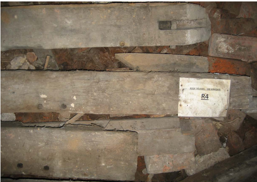
Figure 19: Timber R4 (group 1), centre (photograph Cathy Tyers, Historic England)
