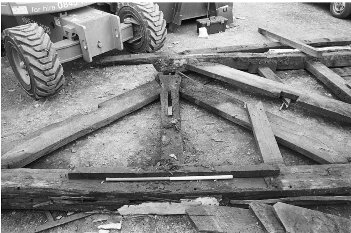
Figure 6: Truss 3 following salvage during demolition (photograph CFA Archaeology Ltd)
