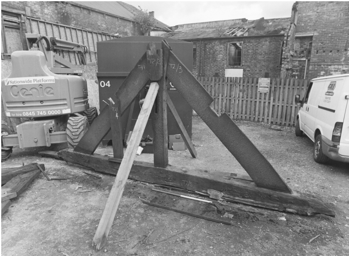
Figure 5: Truss 2 following salvage during demolition (photograph CFA Archaeology Ltd)
