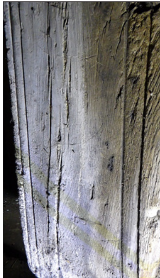
Fig 7 (left): bressumer re-used as support for tie-beam, replacing post e: mortices in upper face for stud wall above and in east face for bearer beams for firehood (© Diane Charlton)
