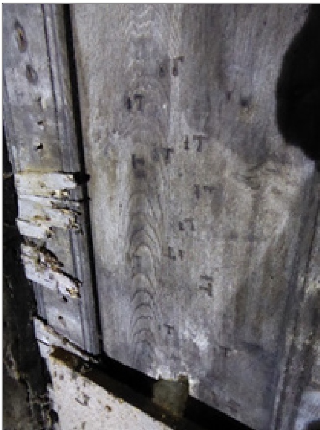
Fig 29: carved initials 'IT' on plank of heck screen, with shallow roll mouldings to studs (©Historic England. Colum Giles)
