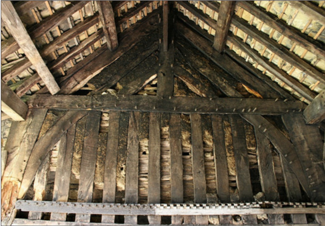
Fig 15: truss IIII, upper walling showing projecting pegs (© Diane Charlton)
