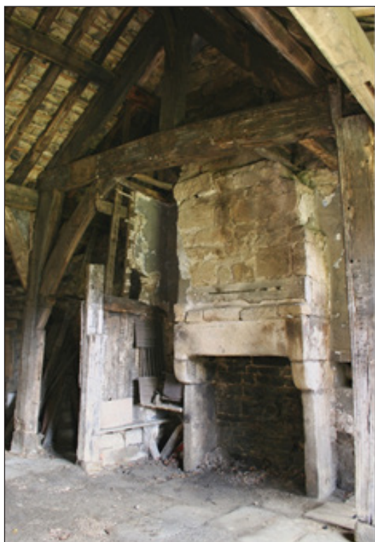
Fig 27 (left): housebody fire area, showing short post f 1 , heck screen and bench and fireplace (© Diane Charlton)
