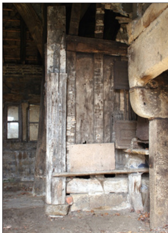
Fig 27 (left): housebody fire area, showing short post f 1 , heck screen and bench and fireplace (© Diane Charlton)
