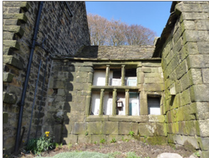
Fig 21 (left): porch, with deep-coursed masonry (©Historic England. Colum Giles)
