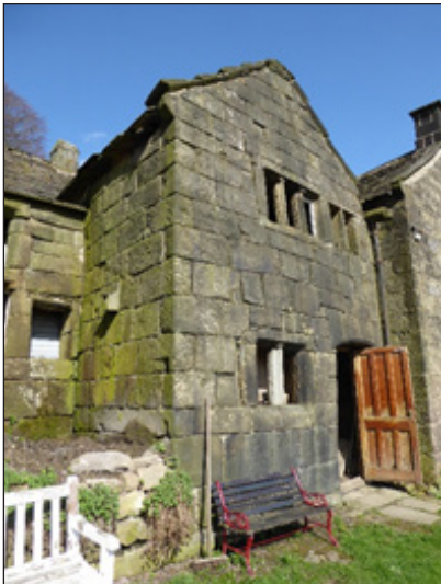
Fig 21 (left): porch, with deep-coursed masonry (©Historic England. Colum Giles)
