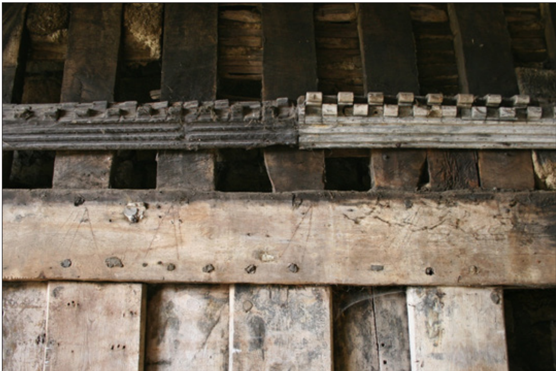
Fig 14: brattished rail, junction of timber: note the carpenters' numbering of the joints (© Diane Charlton)
