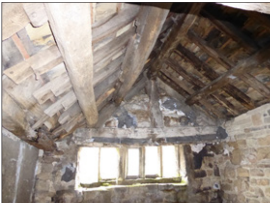
Fig 23 (left): porch first floor, view to south showing king-post truss in south wall: note tie beam shorter than width of porch (©Historic England. Colum Giles)
