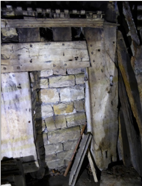
Fig 11: Truss III, post h, showing upper and lower mortices for screen at end of dais (©Historic England. Colum Giles)
