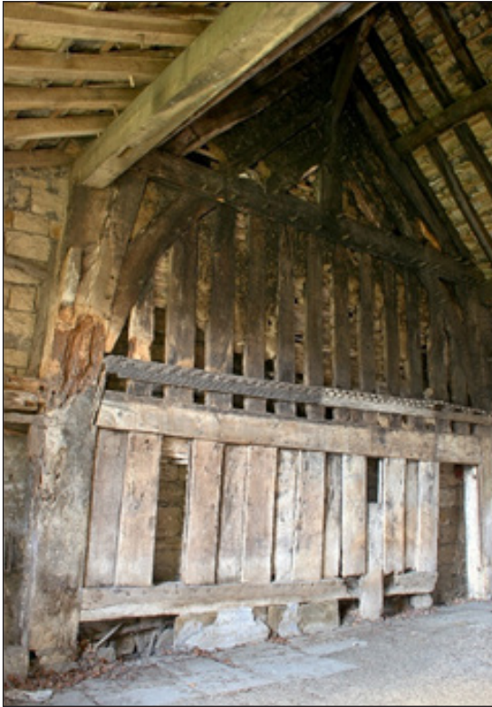
Fig 3 (left): the housebody, view to north west showing truss IIII with plank and muntin screen (© Diane Charlton)
