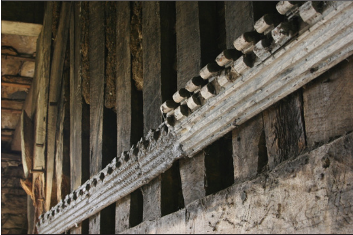
Fig 13: brattished rail fixed to truss IIII above mid rail (© Diane Charlton)
