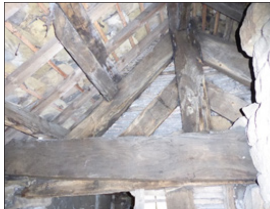
Fig 23 (left): porch first floor, view to south showing king-post truss in south wall: note tie beam shorter than width of porch (©Historic England. Colum Giles)
