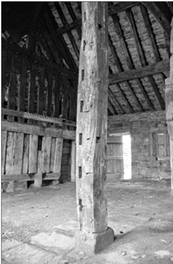
Fig 7 (left): bressumer re-used as support for tie-beam, replacing post e: mortices in upper face for stud wall above and in east face for bearer beams for firehood (© Diane Charlton)
