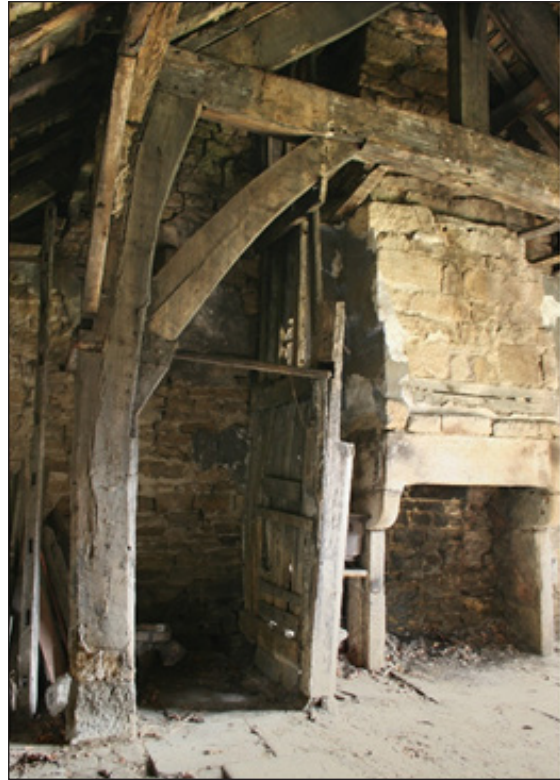
Fig 3 (left): the housebody, view to north west showing truss IIII with plank and muntin screen (© Diane Charlton)
