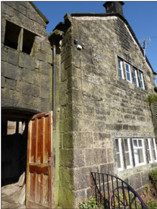
Fig 18 (left): east wing at junction with porch, showing first phase of deep-coursed masonry (©Historic England. Colum Giles)
