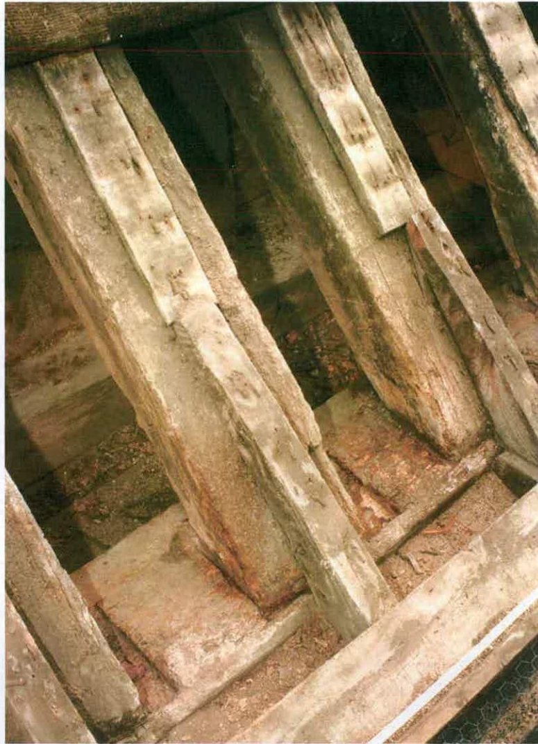
Fig. 41, the rafter ends above the north wall of the Guard Room, set in their housings in the outer wall plate. Photograph: October 1995.
