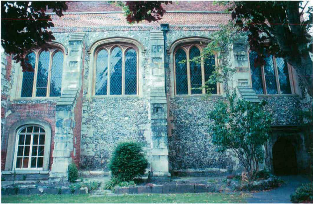
Fig. 21, the south wall of the Great Hall. Photograph: August 1993.
