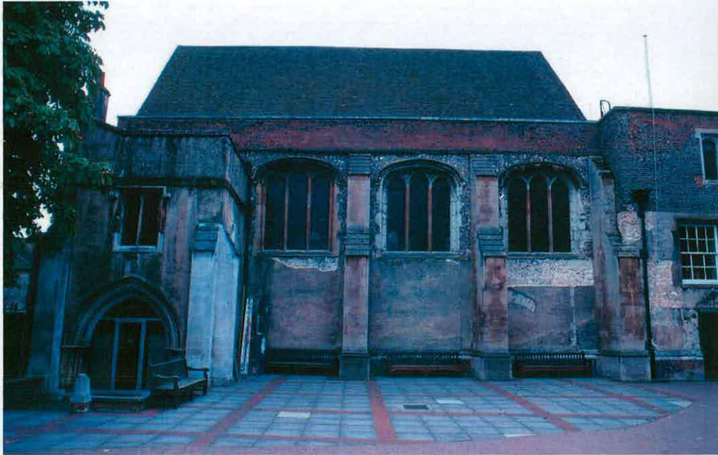
Fig. 20, the north wall of the Great Hall. Photograph: August 1991.
