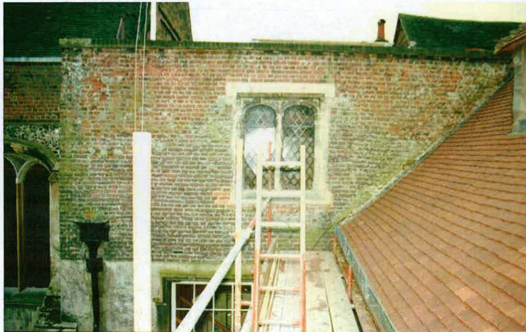
Fig. 10, the north wall of the south-east range. Photograph: November 1987.
