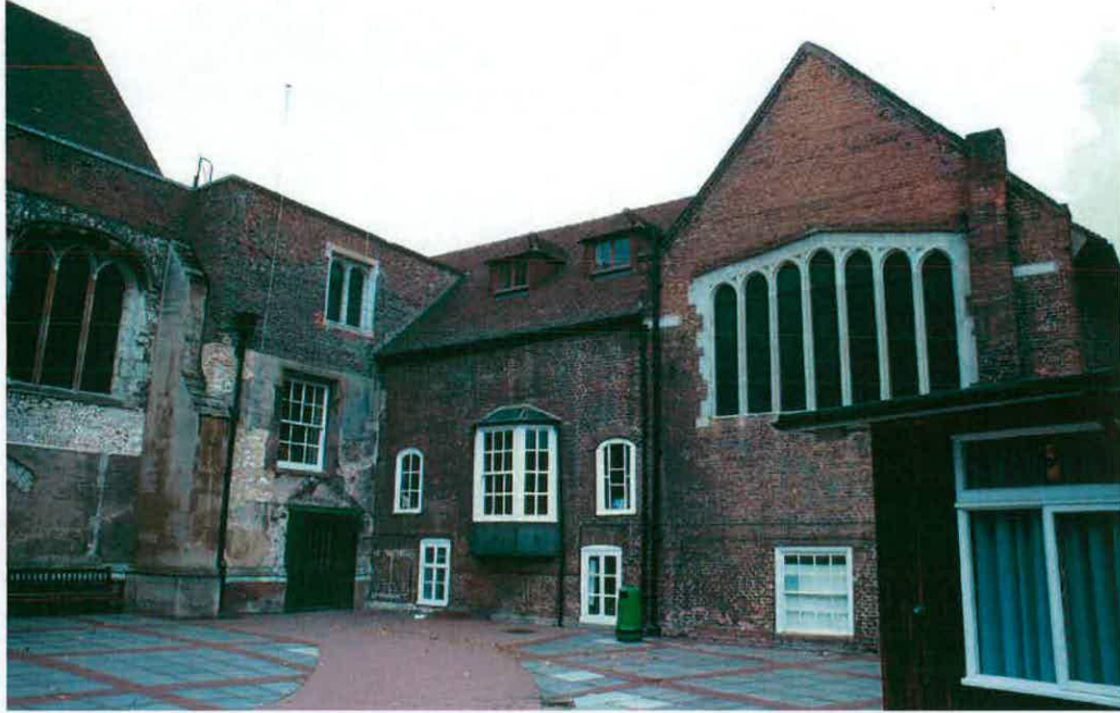
Fig. 9, the junction between the north-east and south-east ranges, viewed from the north-east. Photograph: August 1991
