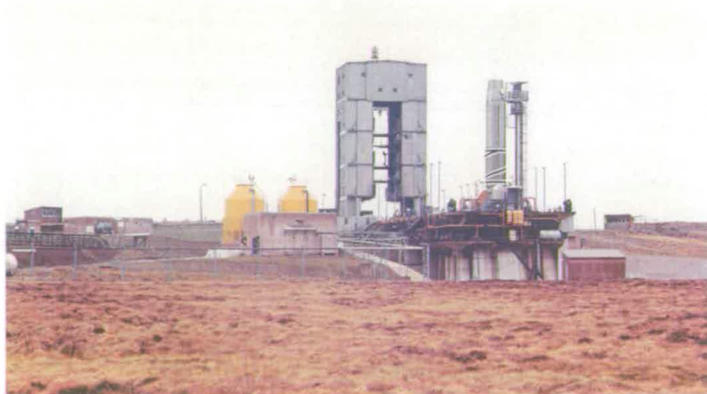
Figure 230 Contemporary photograph of Missile Test Stand C3 showing two large yellow LOX storage tanks to the west of the causeway © Rolls-Royce plc
