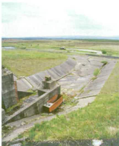
Figure 155 On the west side of Engine Test Stand A2 is a metal tank of unknown function. This is located adjacent to one of the concrete supports which held the steel framework tower © English Heritage NMR (DP003894)
