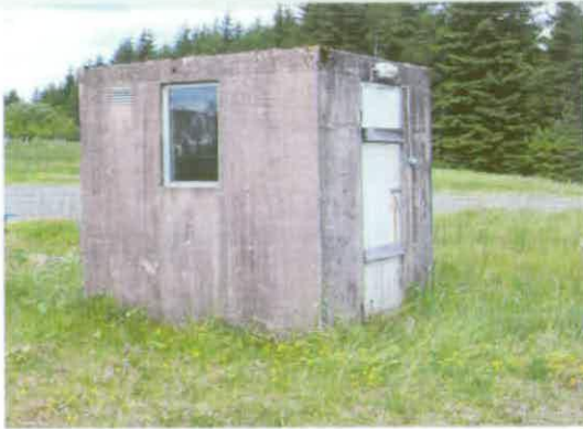
Figure 294 Reinforced concrete Police Post at the junction of roads leading to Greymare Hill and Berry Hill © English Heritage (AF00134/greypolice)
