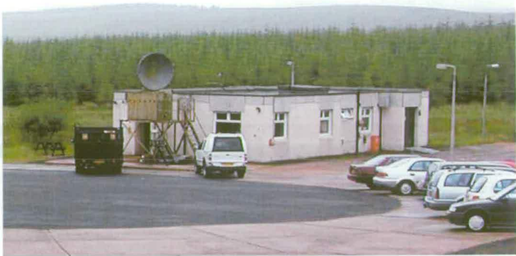
Figure 306 Office Q110 in the Meteorological Station © English Heritage (AF00134/Q110)
