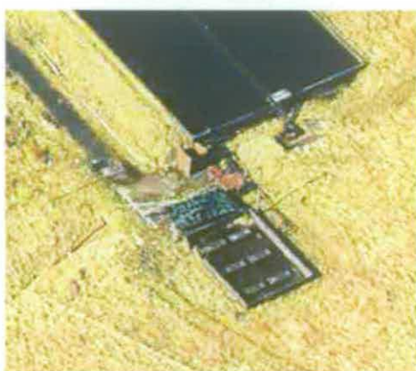
Figure 202 Immediately east of the Effluent Lagoon is the Waste Kerosene System A14.1 © English Heritage NMR (17819/01)
