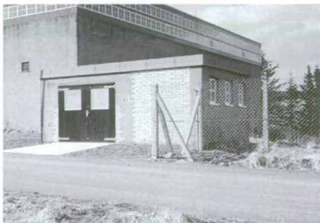
Figure 98 Police Control Post B5 © Crown copyright NMR (AA94/2936)
