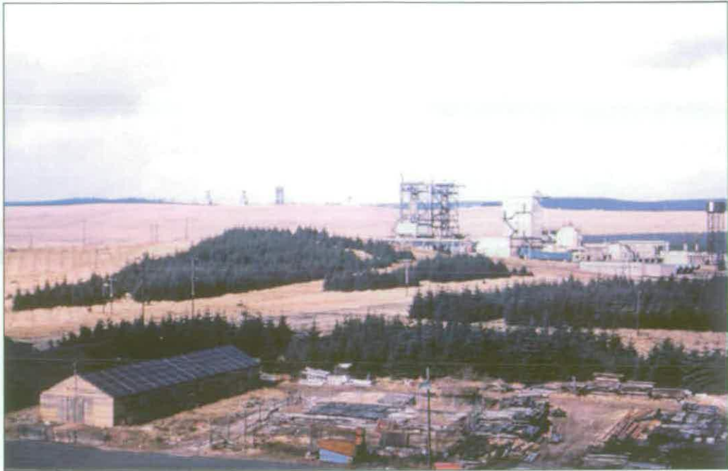
Figure 93 Contemporary photograph of the Equipment Yard taken from the BOC Compound looking north. The partially constructed Component Test and Engine Test Areas are visible in the background © Rolls-Royce plc
