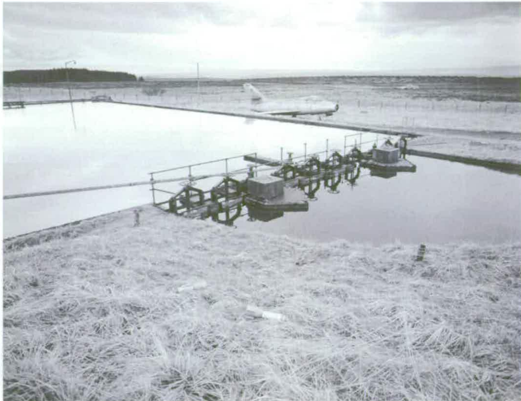
Figure 201 Storm water, cooling water and unspent fuel were collected in an Effluent Lagoon A14 to the south-east of the test stands © Crown copyright NMR (AA94/1971)
