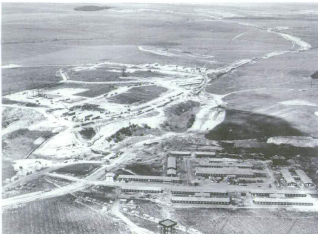
Figure 28 An aerial photograph taken in 1957 shows the arrangement of temporary labourers' huts at Paddy's Camp © Rolls-Royce plc
