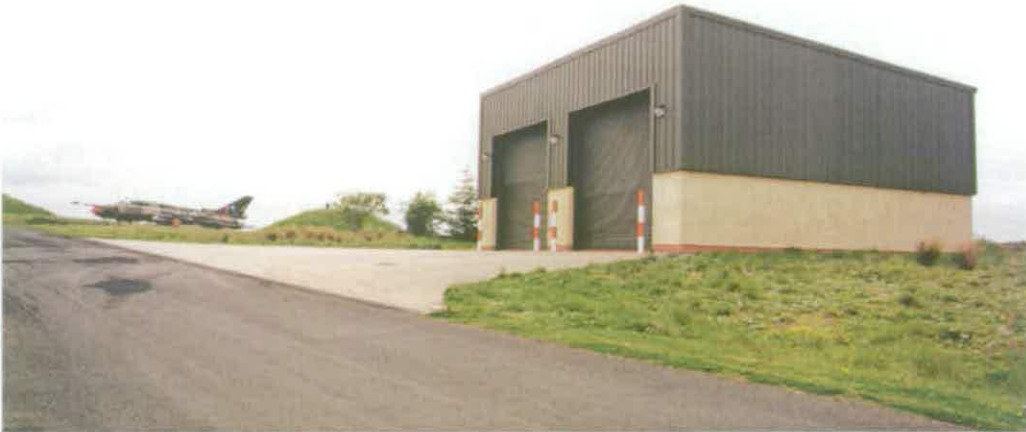
Figure 207 Modern Garage A13. In the background is a Fitter SU22-M, one of the derelict aircraft positioned on the site for training purposes © English Heritage NMR (DP003881)
