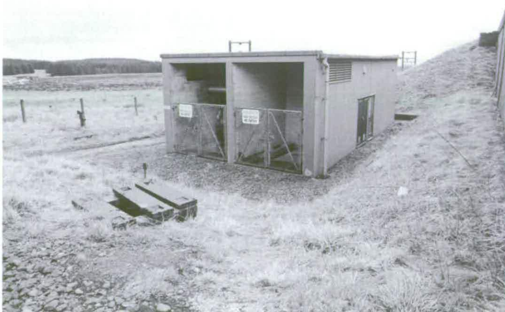
Figure 175 Electricity Sub-station A10.1 © Crown copyright NMR (AA94/1945)
