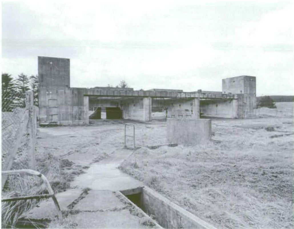
Figure 110 The floors of the test cells sloped to the east draining unspent fuel into the effluent system © Crown copyright NMR (AA94/1931)
