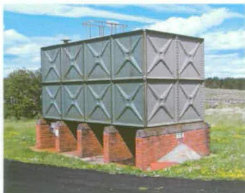
Figure 186 Steel Braithwaite water tank A29 © English Heritage (AF00134/A29)
