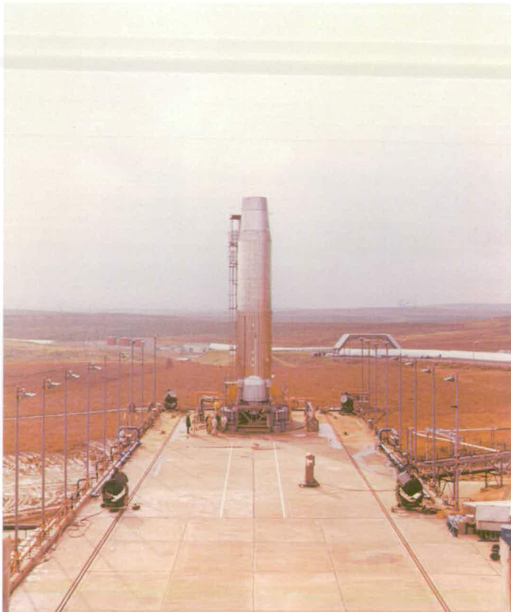
Figure 215 Contemporary photograph of the causeway of Missile Test Stand C3 showing a vehicle in place on the thrust pad © Rolls-Royce plc
