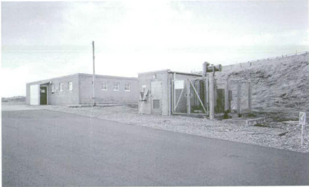
Figure 262 High voltage electrical Sub-Station C5.2 © Crown copyright NMR (AA94/2886)
