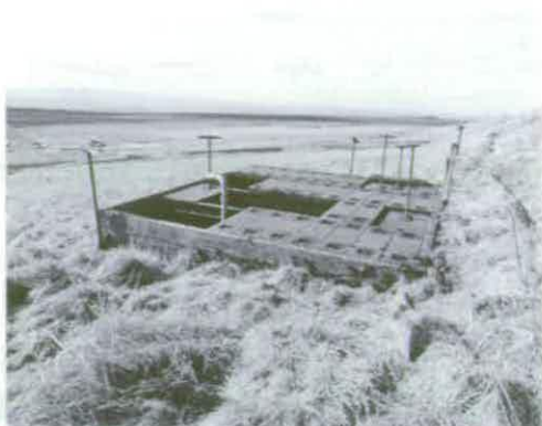
Figure 184 Valve Pit to the west of Engine Test Stand A1 (left) © Crown copyright NMR (AA94/1962)
