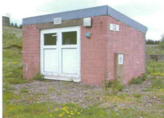
Figure 275 Water Booster Pump House C18 © English Heritage (AF00134/C18)
