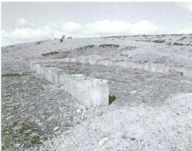
Figure 234 High Pressure Nitrogen Booster Storage Tanks C16 © Crown copyright NMR (AA94/2041)
