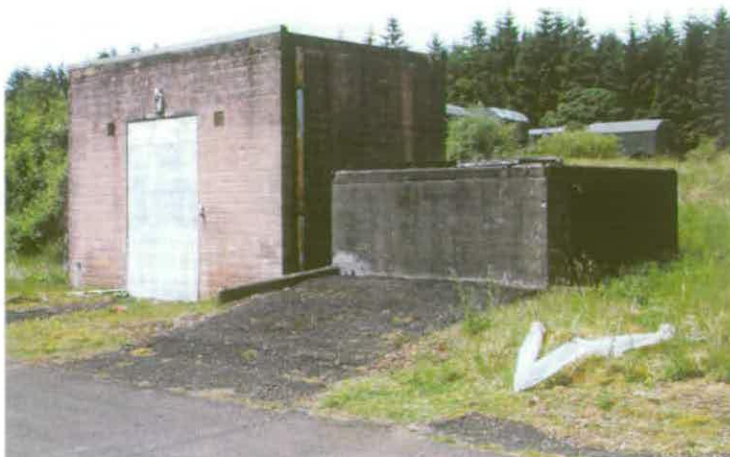
Figure 86 Cooling Water Treatment Plant D16.1 © English Heritage NMR (AF00134/ D16.1)
