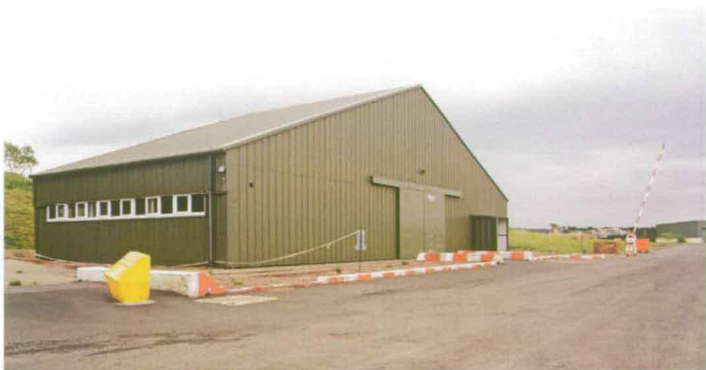
Figure 204 The Engine Preparation Building A6 has been re-clad in pressed steel © English Heritage NMR (DP003902)
