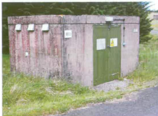
Figure 296 Sub-Station H1.1 at the entrance to H Site © English Heritage (AF00134/H1.1)
