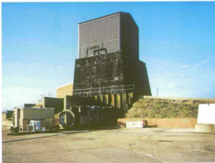
Figure 12 Blue Streak vertical firing point at the Rocket Propulsion Establishment, Westcott, Buckinghamshire. Octagonal section in foreground is part of a one-sixth scale silo model © Crown copyright NMR (BB94/4874)
