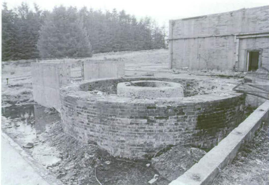
Figure 108 Liquid Oxygen Storage Facility B8 looking south-west © Crown copyright NMR (AA94/1939)
