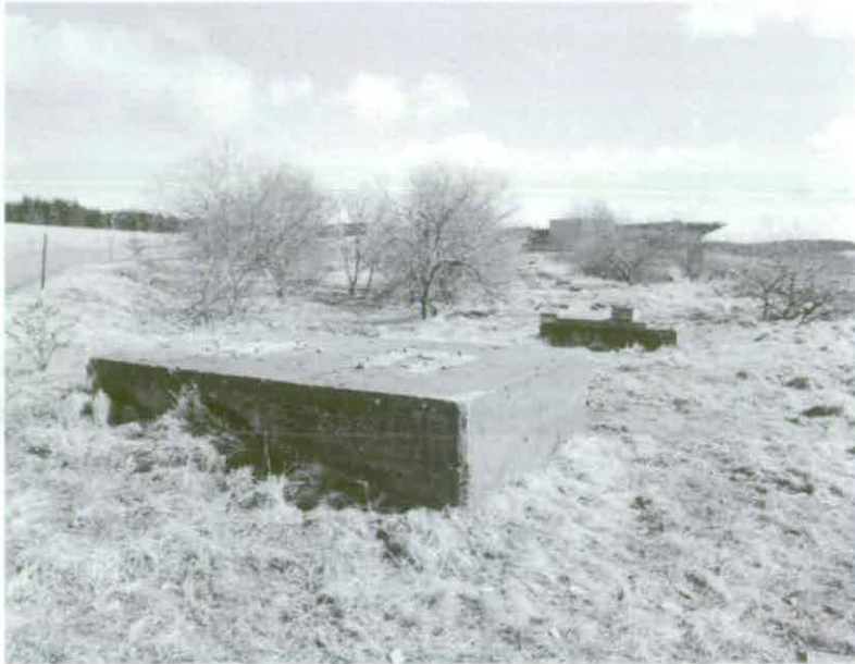
Figure 250 Two concrete blocks to the east of the access road supported the Instrumentation Duct gantry. Missile Test Stand C3 is in the background © Crown copyright NMR (AA94/2001)
