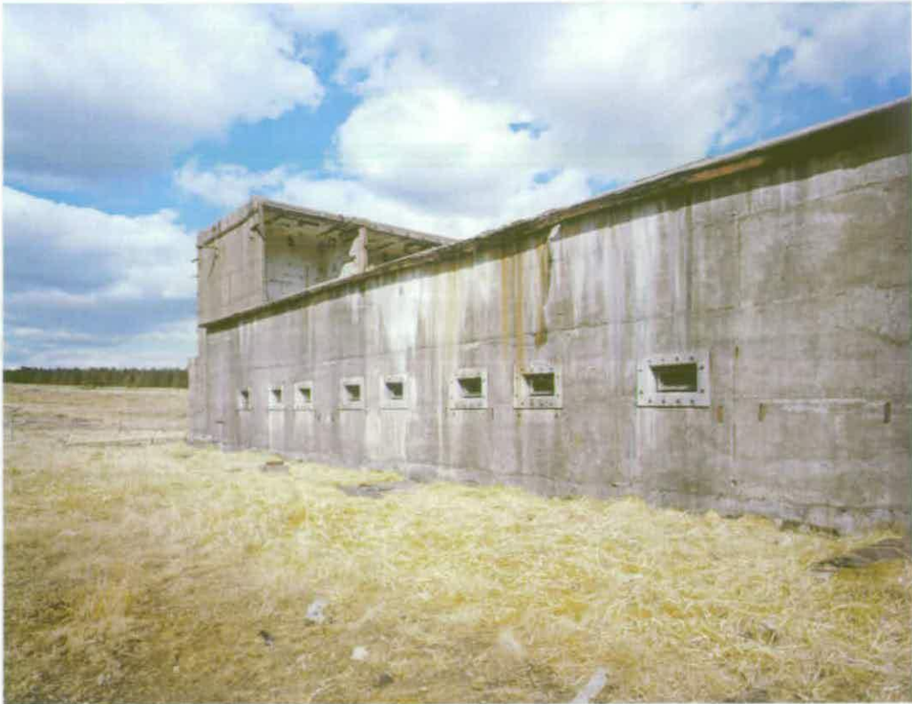
Figure 99 Component Test Area Control Room B1 © Crown copyright NMR (AA94/2952)
