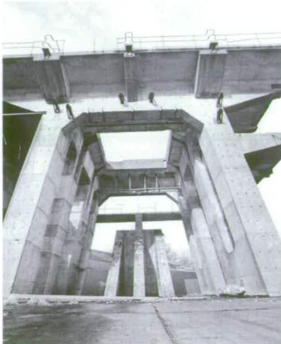
Figure 260 Thrust pad of Missile Test Stand C2 © Crown copyright NMR (AA94/2013)
