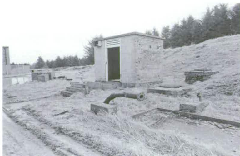
Figure 126 Switch House B2.3 © Crown copyright NMR (AA94/1940)
