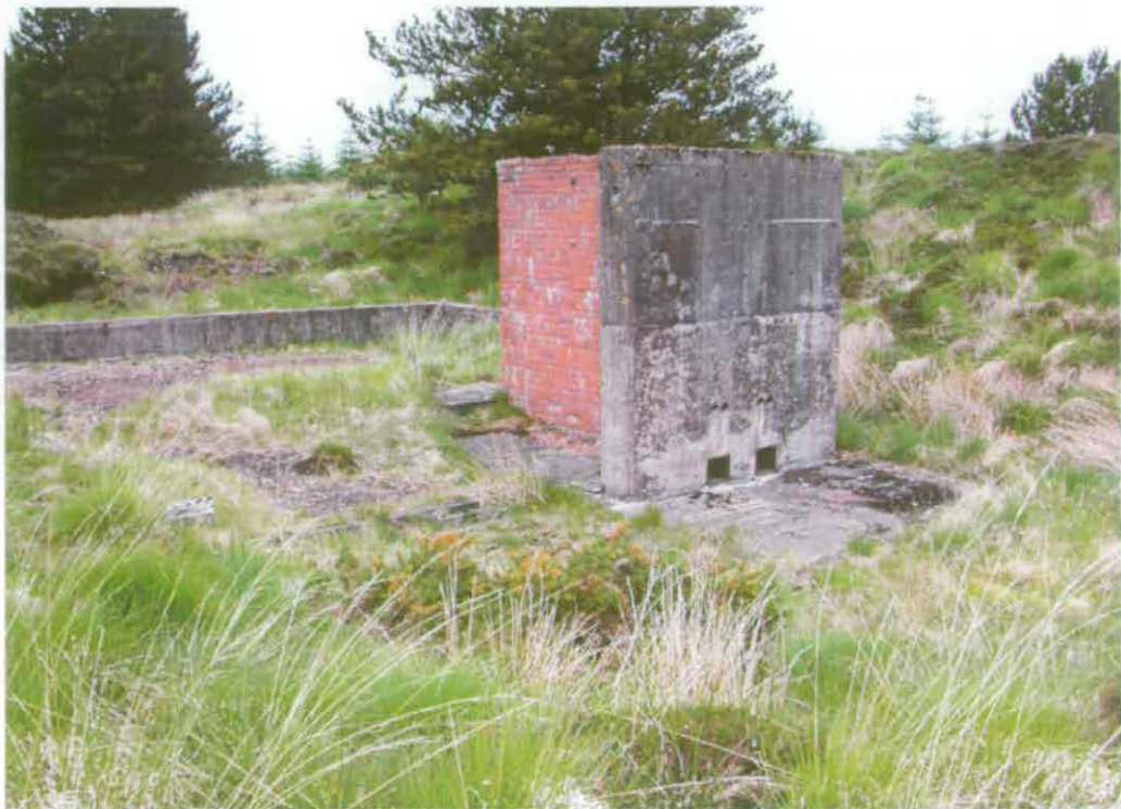
Figure 129 Remains of the Liquid Hydrogen-Liquid Oxygen Thrust Chamber Facility © English Heritage (AF00134/Thrust Chamber)
