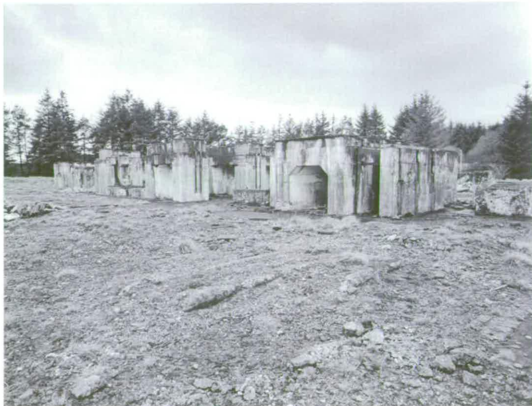
Figure 81 Concrete bases supported equipment used in the production of cryogenics in building D1 © Crown copyright NMR (AA94/2904)
