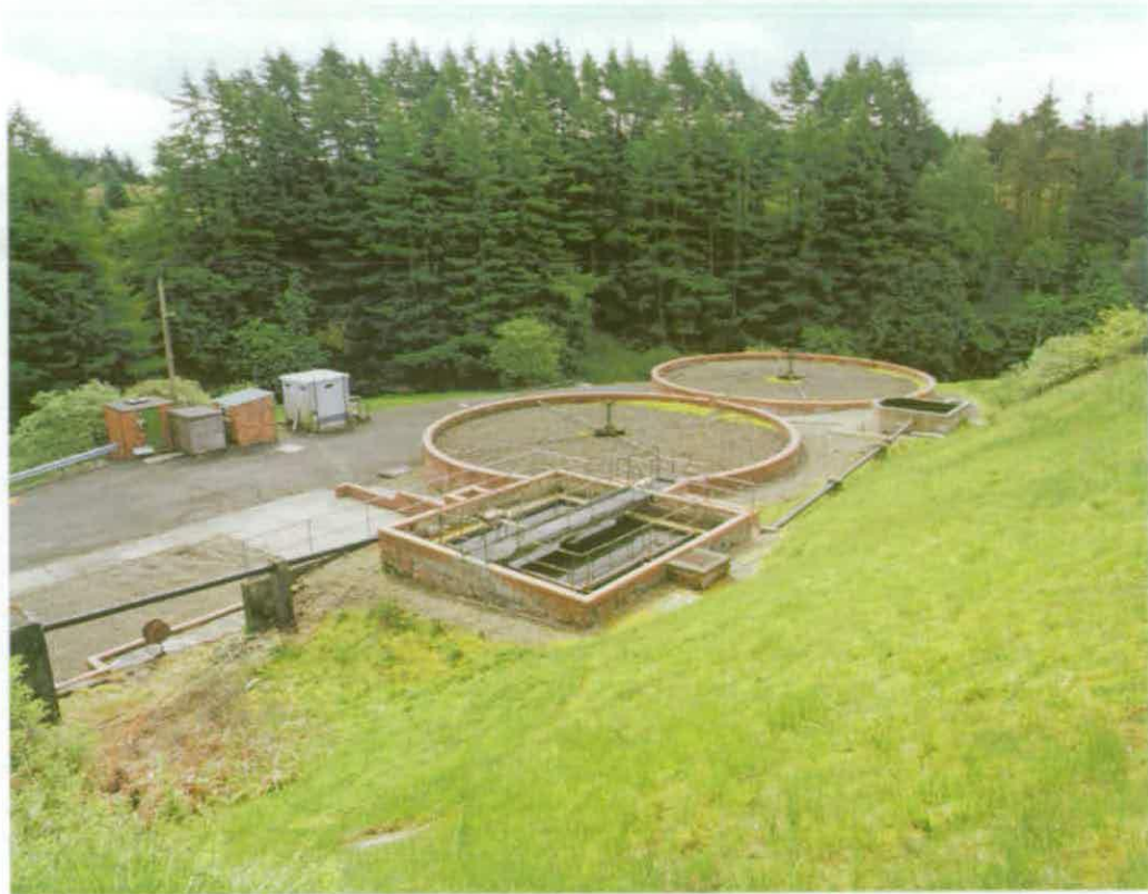
Figure 32 Sewage Plant © English Heritage NMR (DP003933)
