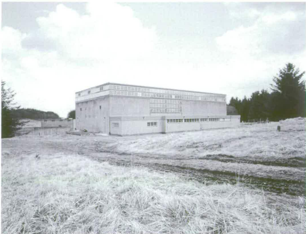
Figure 118 Water Flow Bench Laboratory B3 © Crown copyright NMR (AA94/2937)
