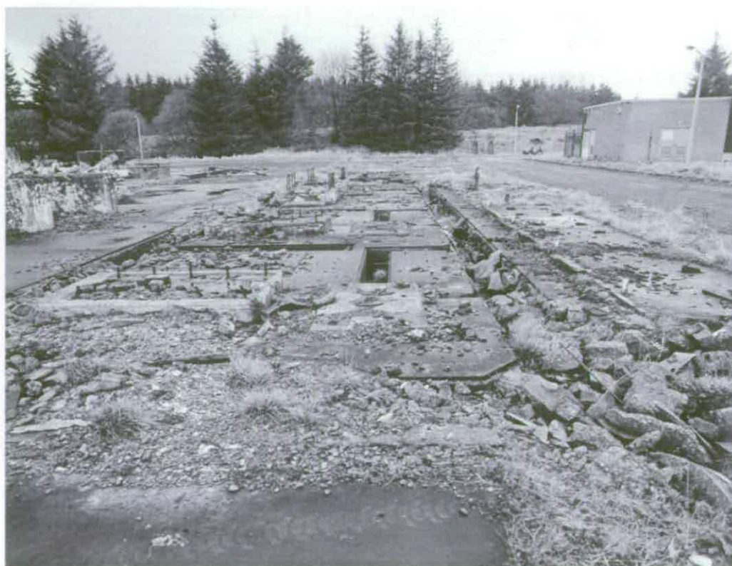
Figure 87 Steel edged conduits and concrete machinery plinths mark the position of the former plant room and electrical switch room © Crown copyright NMR (AA94/2909)
