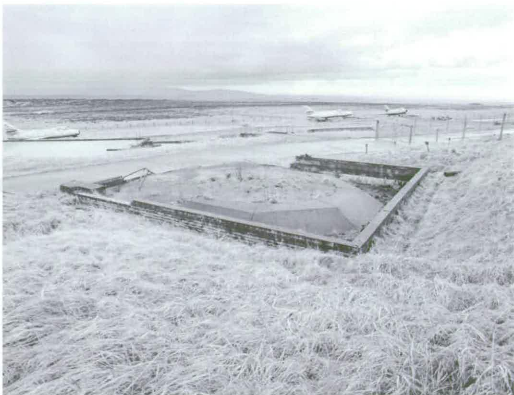
Figure 146 Support for a Kerosene Dump Tank A33.1 that received fuel from Engine Test Stand A1 in an emergency © Crown copyright NMR (AA94/1967)
