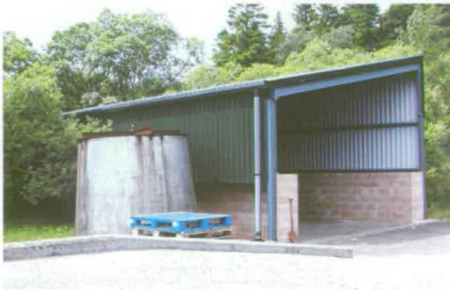
Figure 62 Modern steel framed garage F113 © English Heritage (AF00134/F113)
