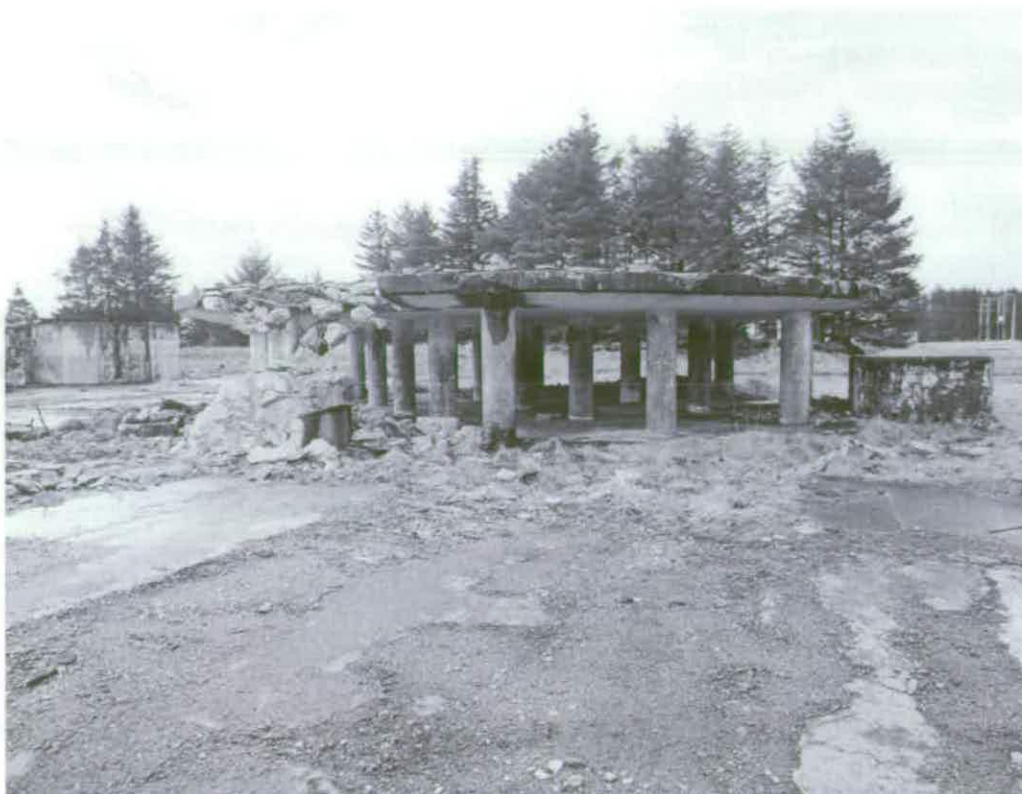
Figure 89 D3, raised concrete support for the Liquid Oxygen Storage Tank © Crown copyright NMR (AA94/2907)
