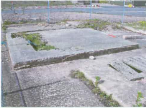
Figure 164 Concrete floor slab of the former Pneumatic Control Station A16.3 © English Heritage (AF00134/A16.3)
