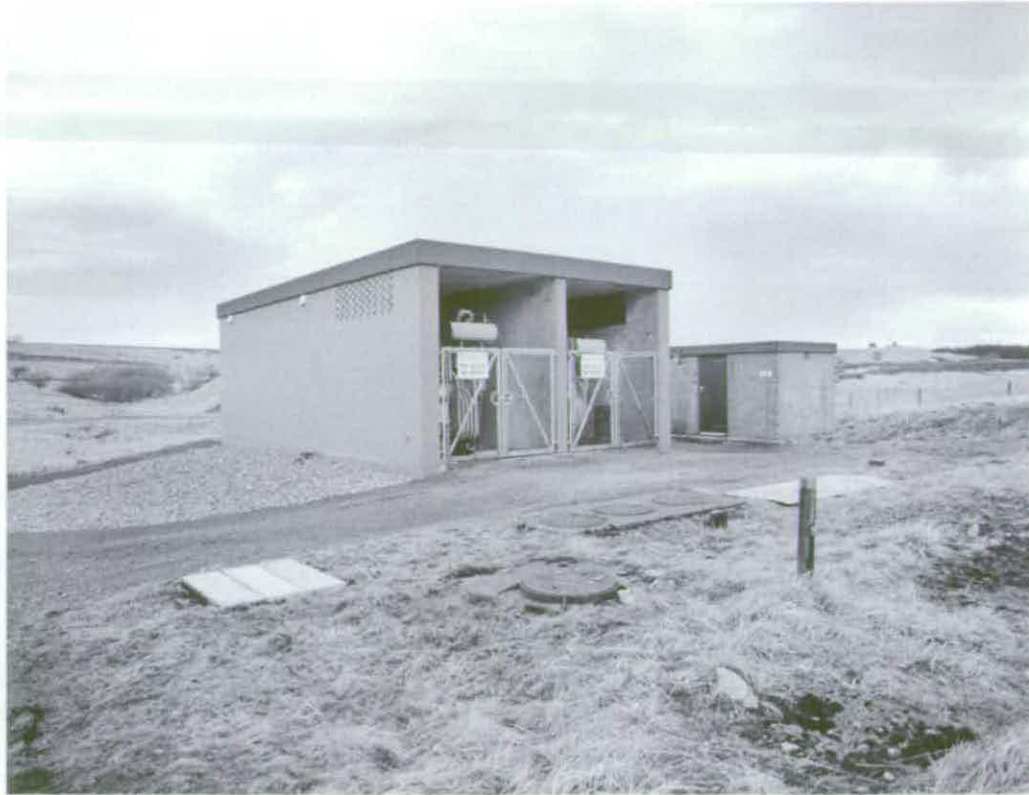
Figure 227 Electrical Sub-Station C5.4 © Crown copyright NMR (AA94/1989)
