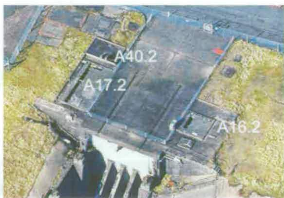
Figure 156 Hardstanding above Test Stand A2 © English Heritage NMR (17797/03)
