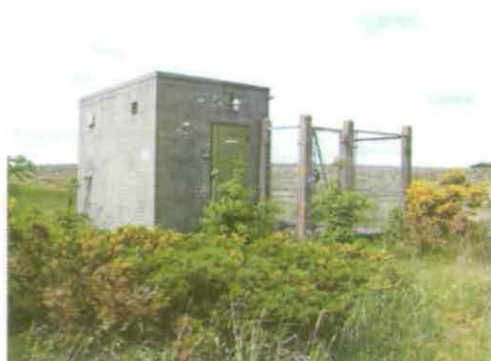
Figure 180 Electricity Sub-Station A10.4 © English Heritage (AF00134/A10.4)
