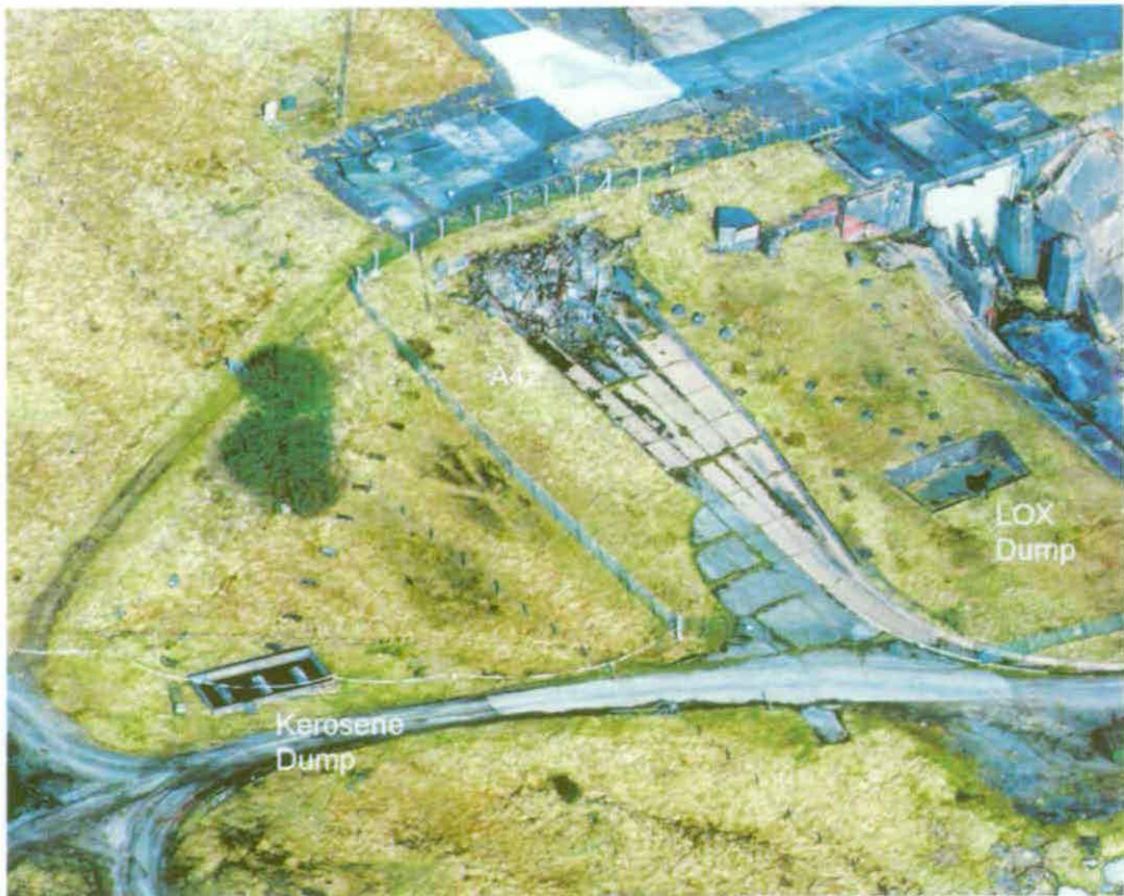
Figure 168 Modern aerial photograph of Engine Test Stand A42 with emergency dump systems for liquid oxygen (LOX) and kerosene
