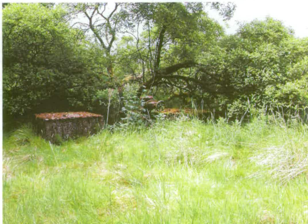
Figure 72 Site of the High Level Water Storage Tank Q2.101 © English Heritage (AF00134/Q2.101)
