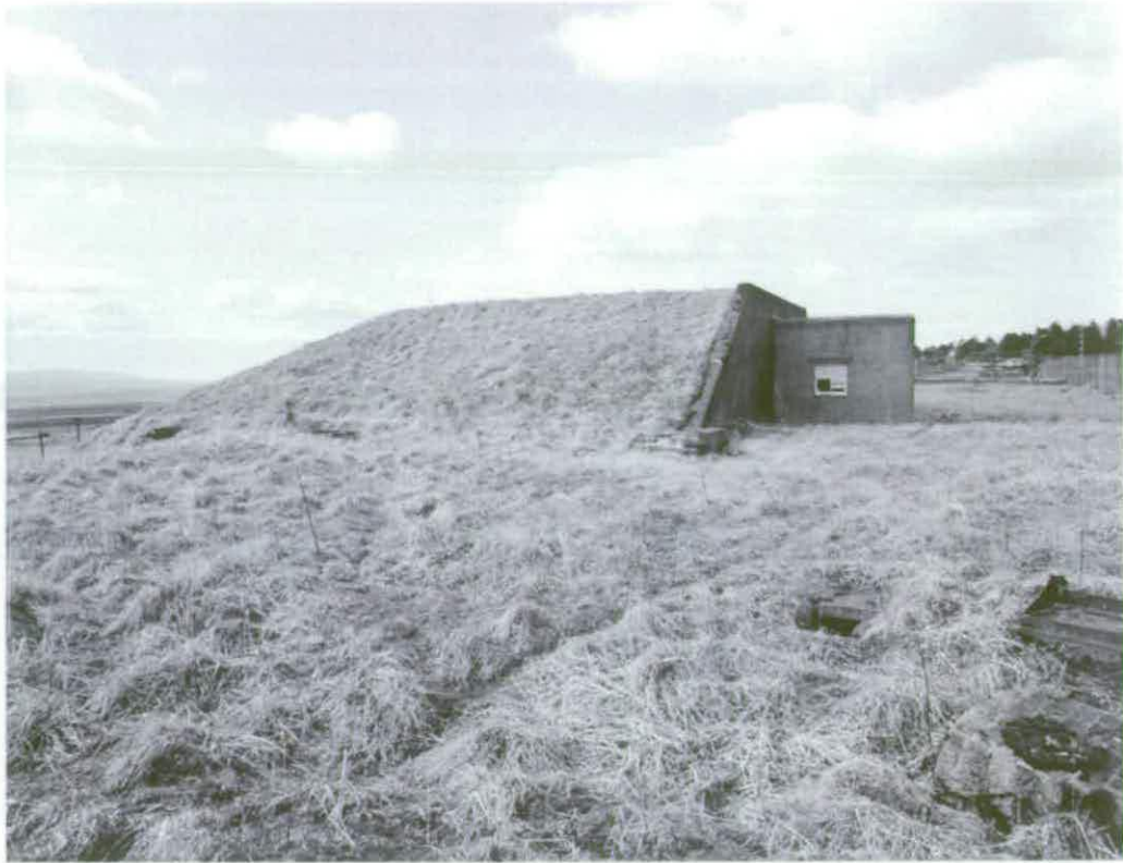
Figure 195 The Terminal House A4 was protected by an earthen mound © Crown copyright NMR (AA94/1965)
