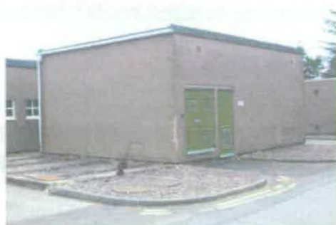
Figure 47 Sub-station F42.2 © English Heritage (AF00134/F42.2)
