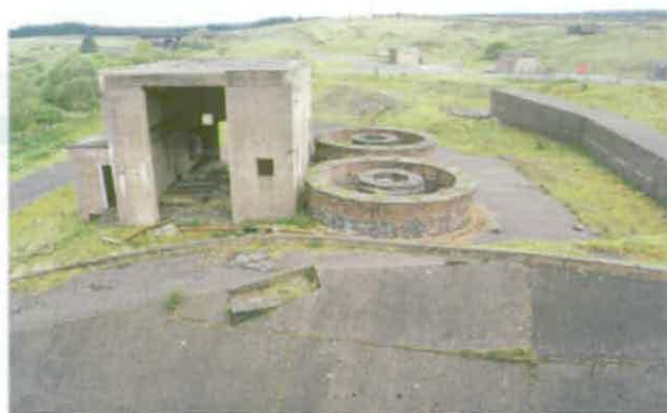
Figure 229 Liquid Oxygen (LOX) Store Tanks and Pump House C3.5 © English Heritage NMR (DP003888)
