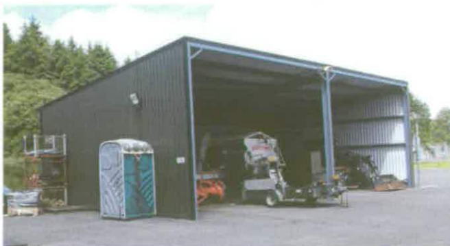
Figure 63 Modern steel framed garage F114 © English Heritage (AF00134/F114)
