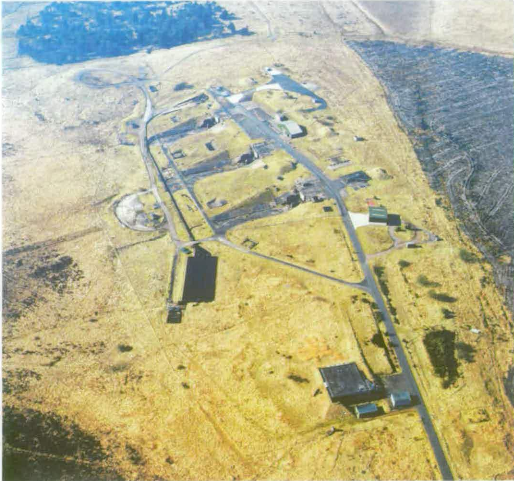
Figure 133 Modern aerial photograph of the Engine Test Area at Priorlancy Rigg © English Heritage NMR (17819/03)
