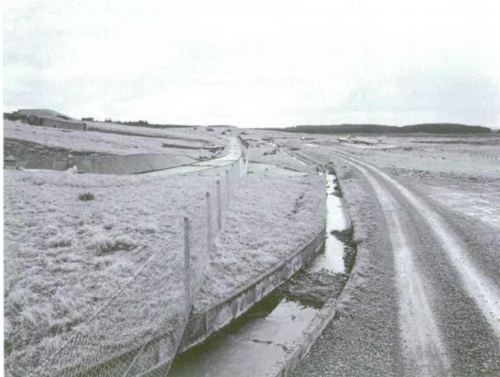
Figure 172 Cooling water and inspent fuel from Engine Test Stand A42 drained into a channel that flanked the south side of the test stands © Crown copyright NMR (AA94/2929)
