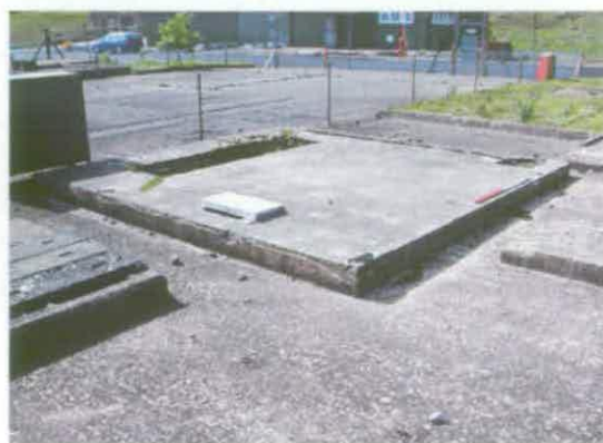
Figure 143 Concrete footing of the Electrical Control Station A17.1 © English Heritage (AF00134/A17.1)
