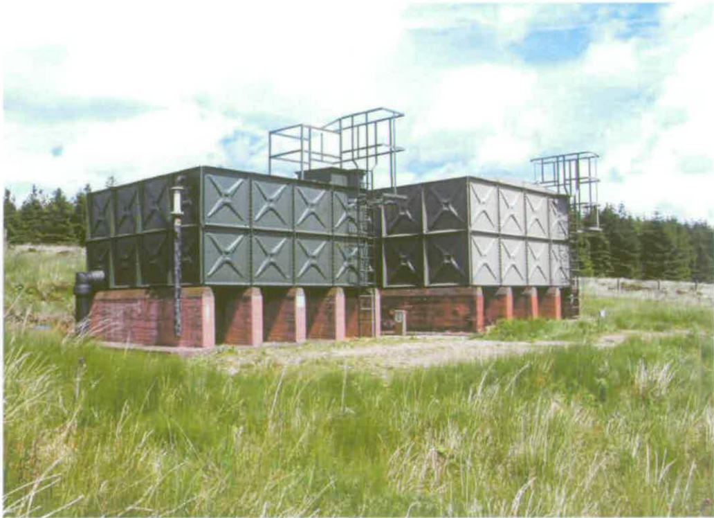
Figure 270 Braithwaite Water Storage Tanks C12 © English Heritage (AF00134/C12)
