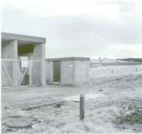
Figure 272 Chemical Treatment Plant C30 (right) © Crown copyright NMR (AA94/1989)
