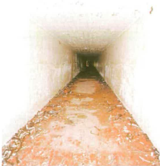
Figure 194 Inside the Instrumentation Duct A8 © English Heritage NMR (DP003916)
