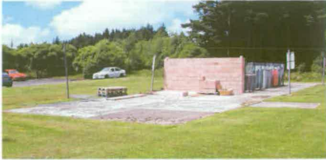
Figure 61 Gas Cylinder Store F111 © English Heritage (AF00134/F111)
