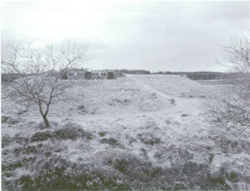
Figure 243 An earthen mound covers the concrete bunker but observation ports remain exposed © Crown copyright NMR (AA94/1992)
