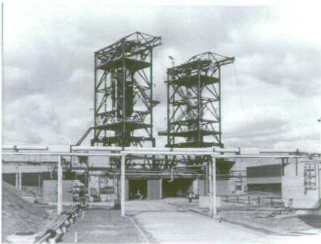
Figure 111 Contemporary photograph showing steel framework towers above the test cells © Rolls-Royce plc
