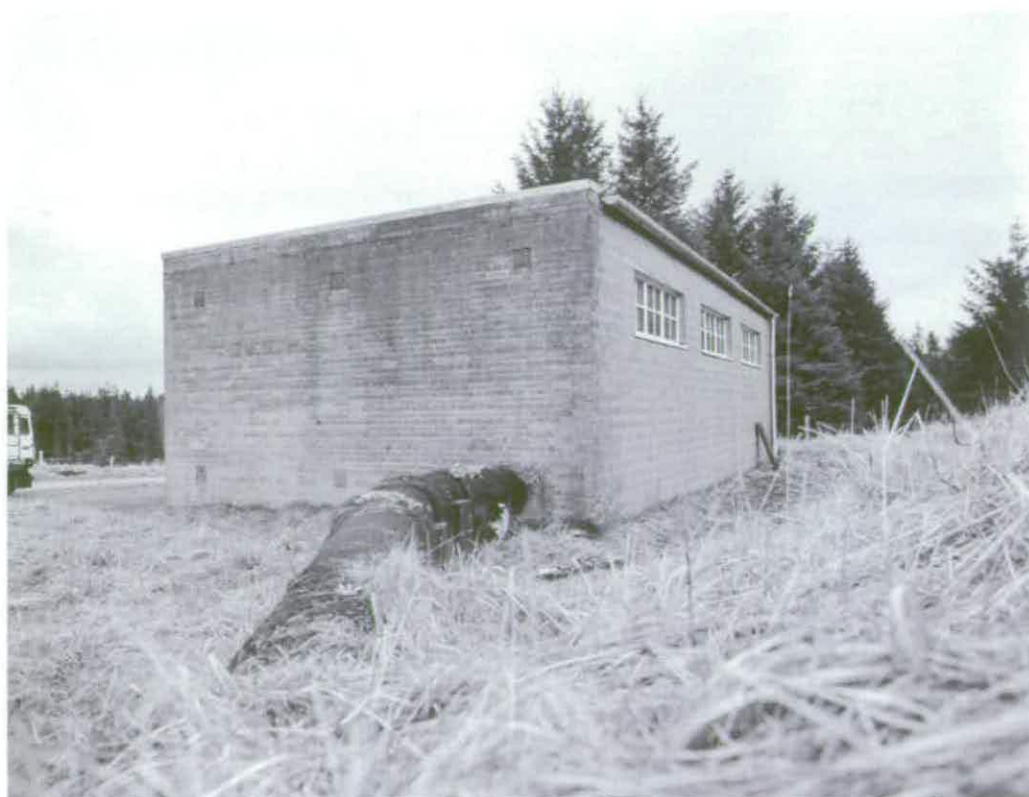
Figure 285 Central Pump House Q25.2 © Crown copyright NMR (AA94/1972)
