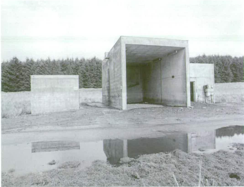
Figure 292 Sub-Station K4.1 (left), Protected Garage K4.2 (centre) and a third building of unknown function K3 (right) © Crown copyright NMR (AA94/2915)
