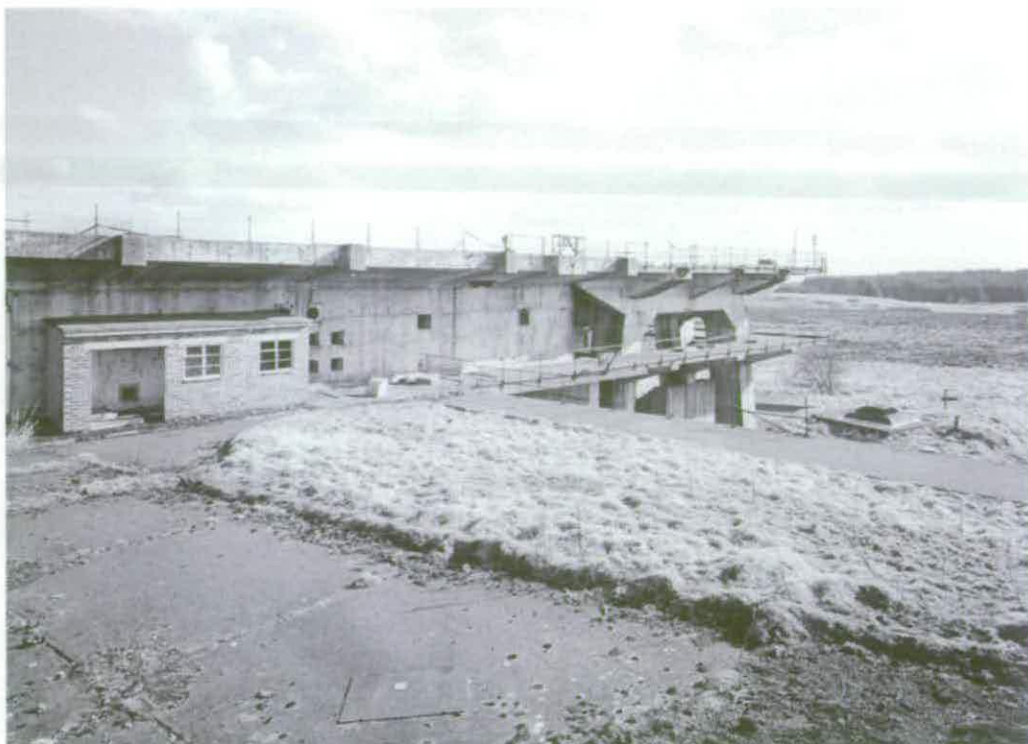
Figure 225 West side of Missile Test Stand C3 showing walkway level and brick outshot © Crown copyright NMR (AA94/2891)
