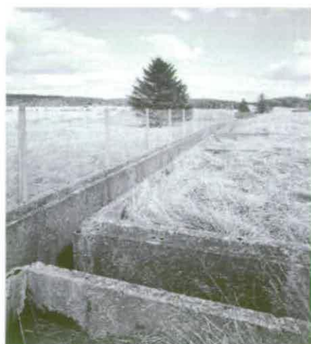
Figure 120 A network of channels that were originally covered fed into a single main Effluent Channel B6 © Crown copyright NMR (AA94/2935)
