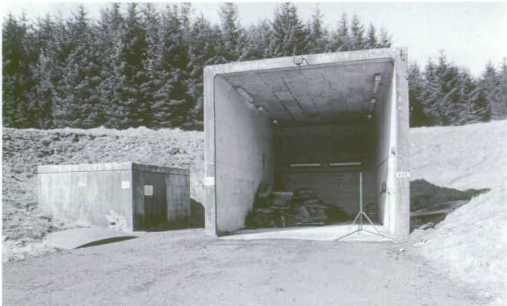
Figure 300 Electricity Distribution Sub-Station H4.2 (left) and Protected Garage H3.2 © Crown copyright NMR (AA94/1986)
