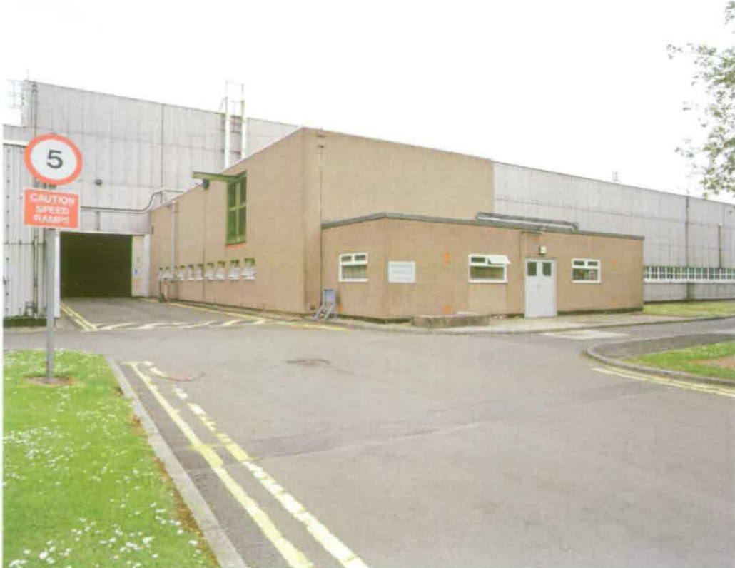
Figure 42 The Main Building F1 comprises two rectangular blocks separated by an internal covered roadway © English Heritage NMR (DP003980)
