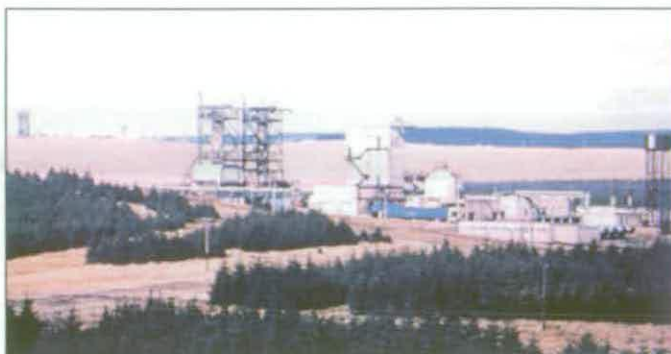
Figure 96 Contemporary photograph of the Component Test Area taken from the BOC Compound looking north © Rolls-Royce plc
