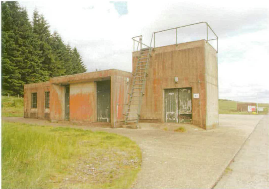
Figure 291 Control Building K1 © English Heritage NMR (DP003988)
