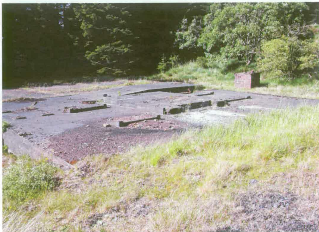
Figure 26 A building footing with complex internal ramps and levels at Paddy's Camp may have been a sub-station © English Heritage (AF00134/paddy3)
