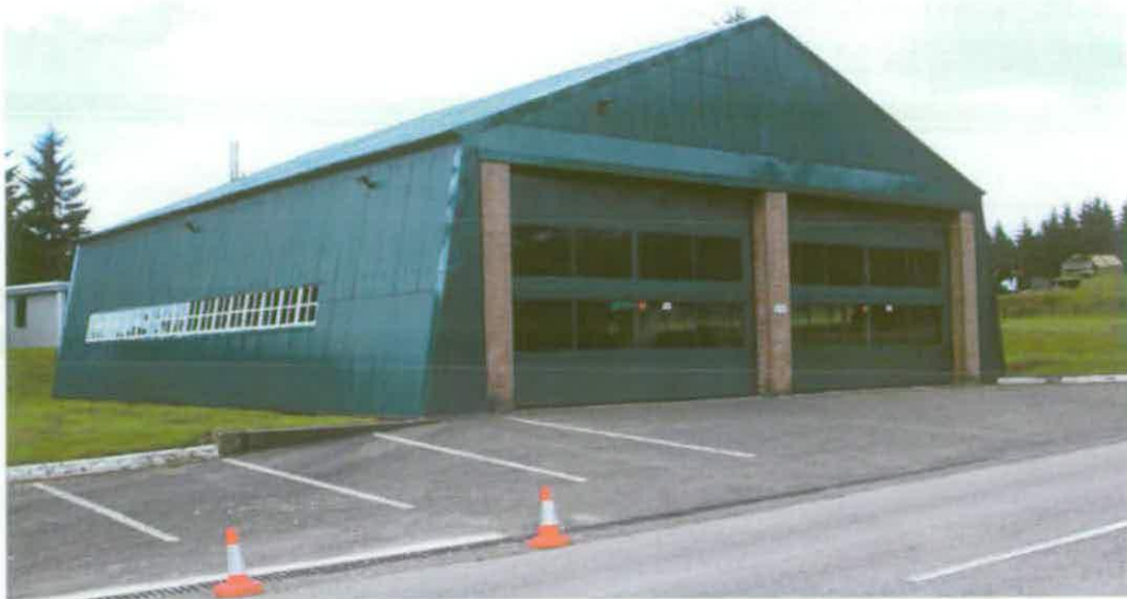
Figure 70 Fire Station Q2.19 © English Heritage (AF00134/Q2.19)
