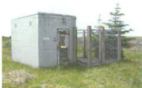
Figure 178 Electricity Sub-Station A10.2 © English Heritage (AF00134/A10.2)
