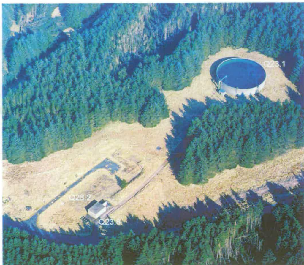
Figure 287 Reservoir Q23 supplied water to the Engine Test Area at Priorlancy Rigg © English Heritage NMR (17818/19)
