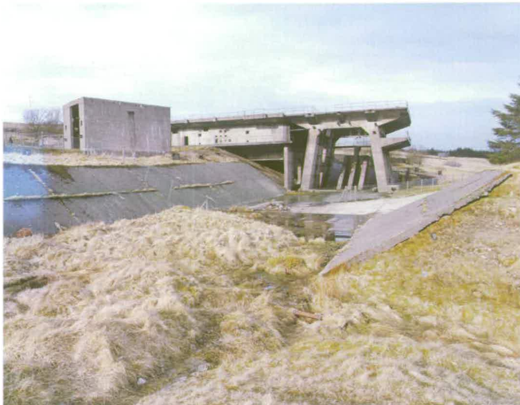
Figure 265 A concrete lined spillway was designed to carry cooling water and unspent fuel to the Effluent Lagoon C31.2 © Crown copyright NMR (AA94/2967)
