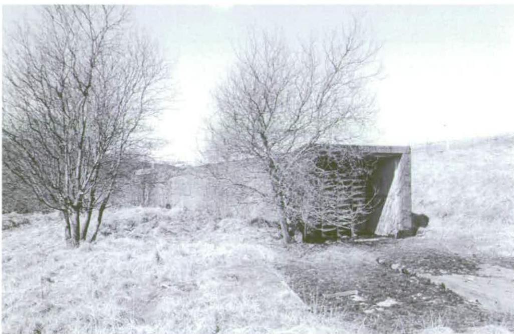
Figure 267 Monitoring and control cables entered a cable tunnel from the Instrumentation Duct © Crown copyright NMR (AA94/2020)
