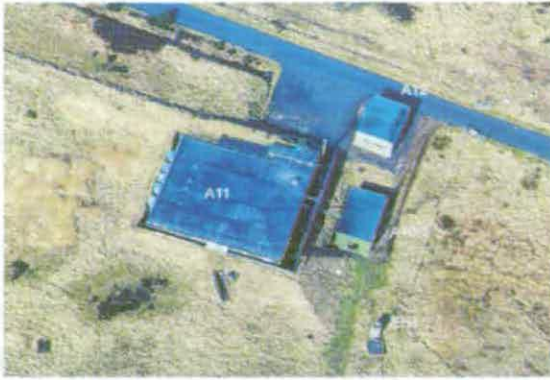
Figure 188 Control Centre A11 © English Heritage NMR (17797/04)
