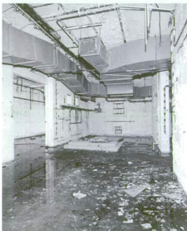
Figure 224 Galvanised metal roof ducting within the Equipment Rooms of Missile Test Stand C3 © Crown copyright NMR (AA94/2895)
