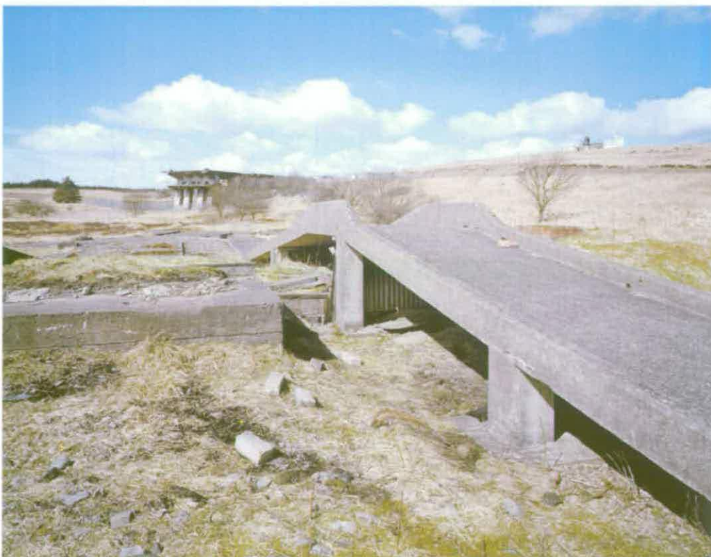
Figure 249 The Instrumentation Duct C22 was carried on a concrete runway © Crown copyright NMR (AA94/2959)
