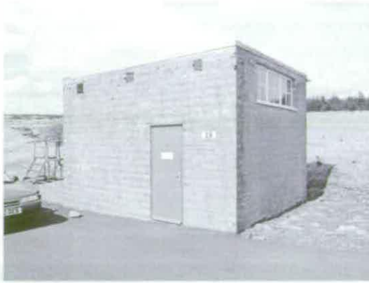
Figure 269 Demineralised Water Plant and Storage C9 © Crown copyright NMR (AA94/2039)
