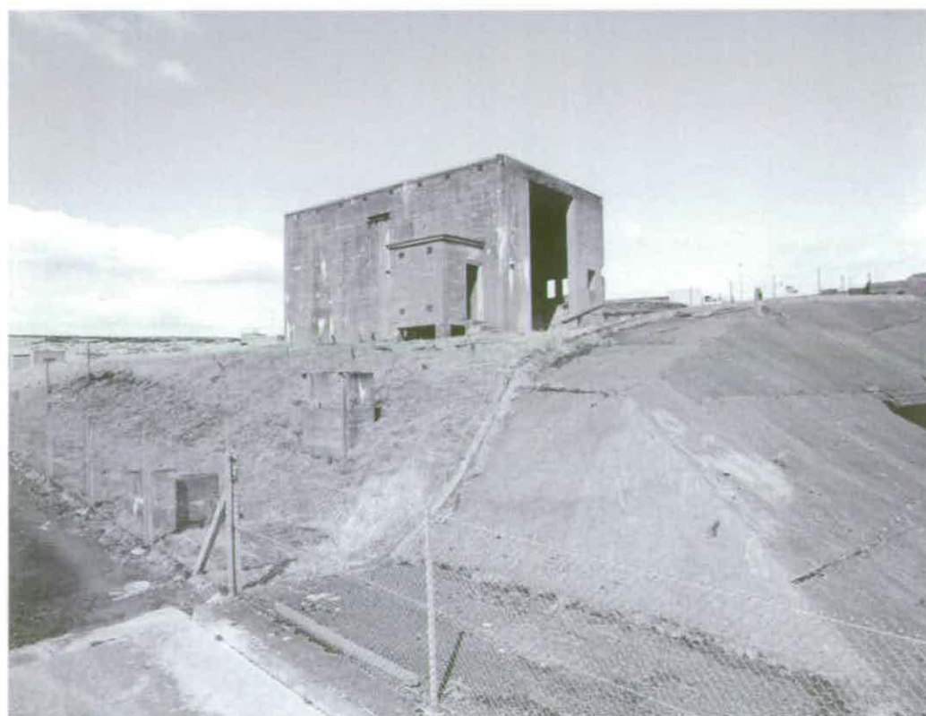
Figure 231 Concrete stanchions to the west of Missile Test Stand C3 carried a pipeline from the test stand to an emergency LOX dump Area
