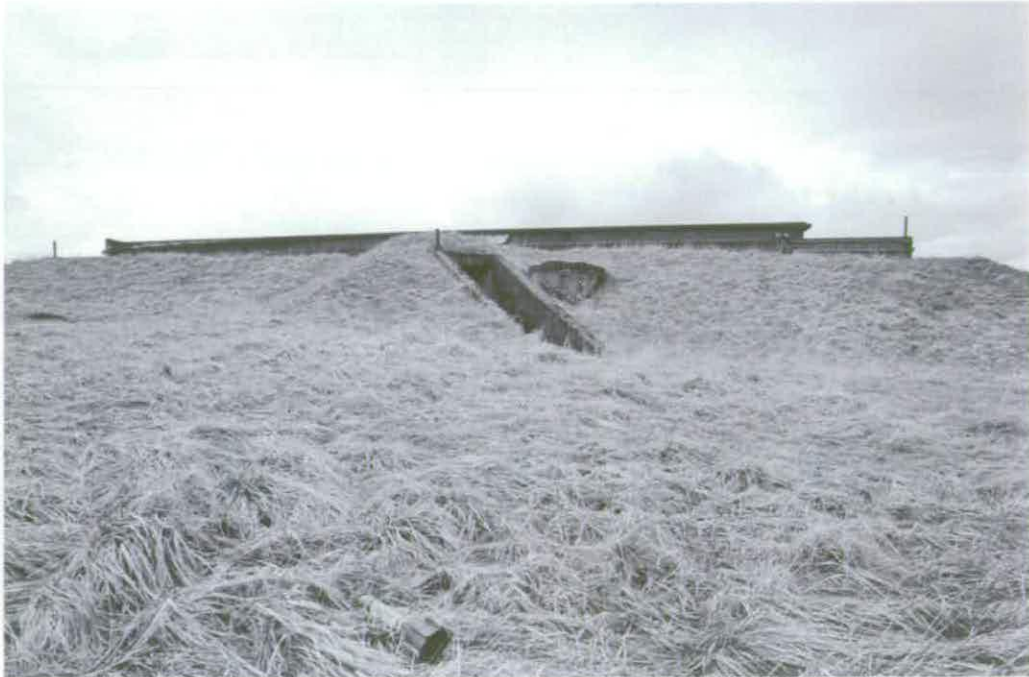
Figure 189 Control Centre A11 is protected on three sides by an earthwork traverse © Crown copyright NMR (AA94/1946)
