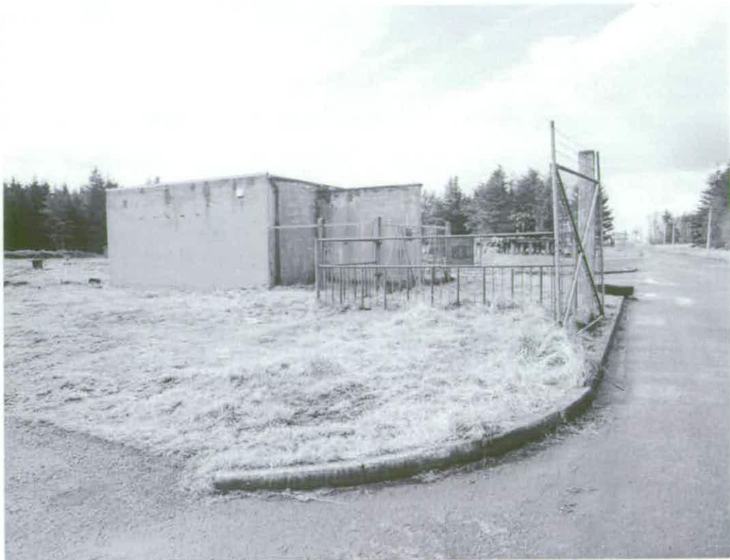
Figure 91 Sub-station D10 © Crown copyright NMR (AA94/2902)
