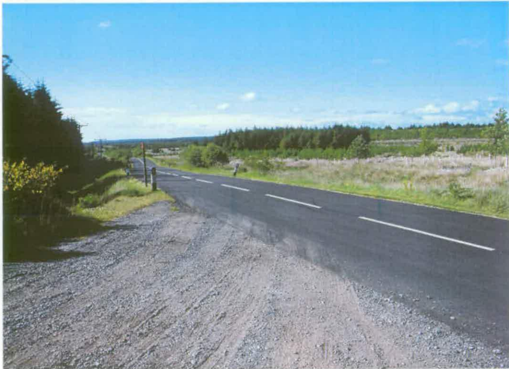
Figure 13 Access roads across waterlogged ground at Spadeadam were constructed on rafts of birch wood and today birch bushes have sprung up along the roadsides © English Heritage (AF00134/road)
