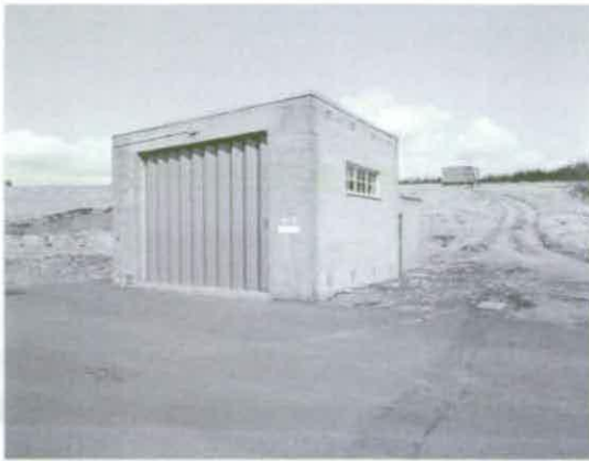
Figure 235 Gaseous Nitrogen Booster Compression House C16.1 © Crown copyright NMR (AA94/2040)
