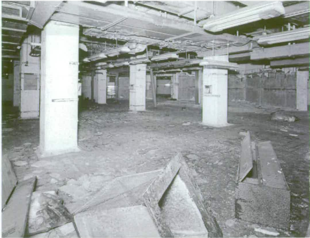
Figure 245 The interior of the Control Centre contained a range of recording equipment © Crown copyright NMR (AA94/2897)
