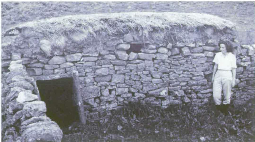
Figure 2 Hut with turf roof at Tinkler Crag © Crown copyright NMR; Ramm et al 1970
