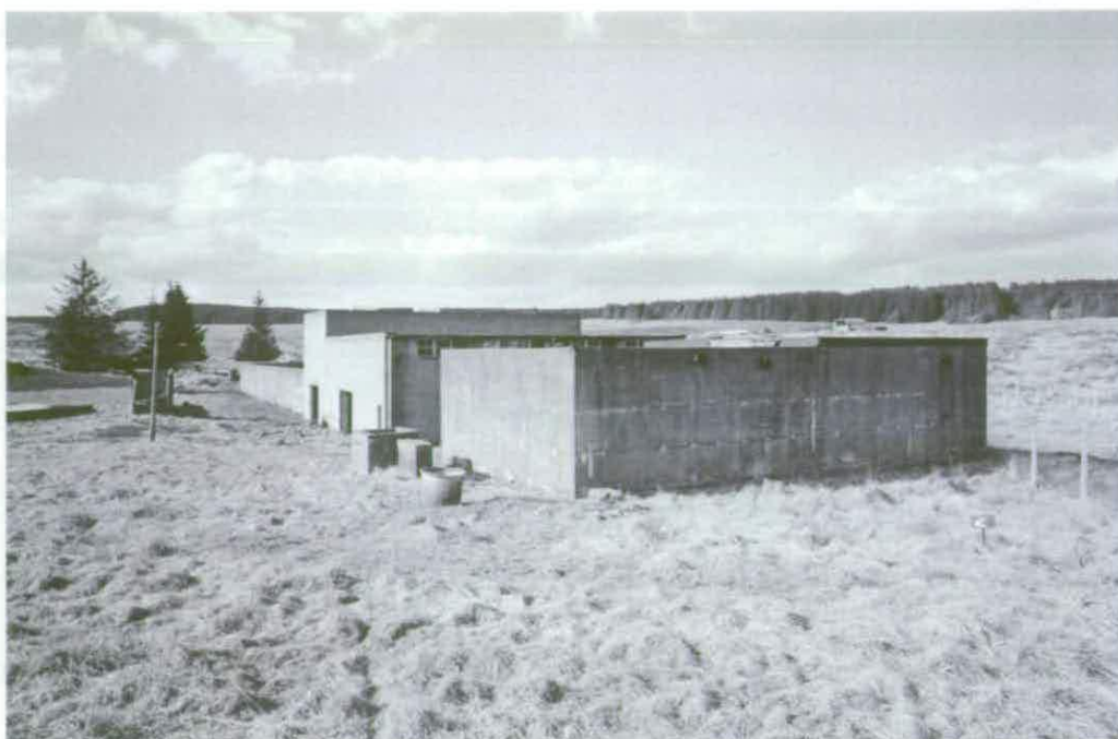
Figure 124 Pump House and Effluent Treatment Plant B6.1 (middle distance) and the Process Water and Firewater Storage Tanks B6.3 (foreground) © Crown copyright NMR (AA94/2934)
