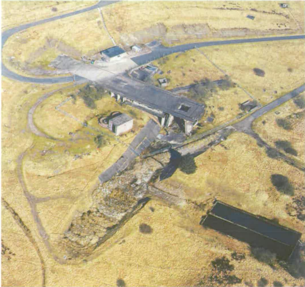
Figure 258 Missile Test Stand C2 was similar to Test Stand C3 but was never completed © English Heritage NMR (17801/04)
