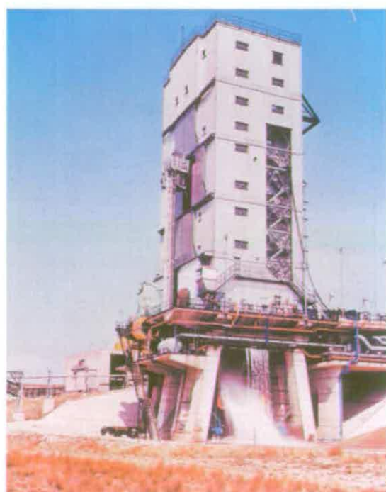
Figure 222 Contemporary photograph of Missile Test Stand C3 showing cooling water pouring from the efflux deflector bucket © Rolls-Royce plc
