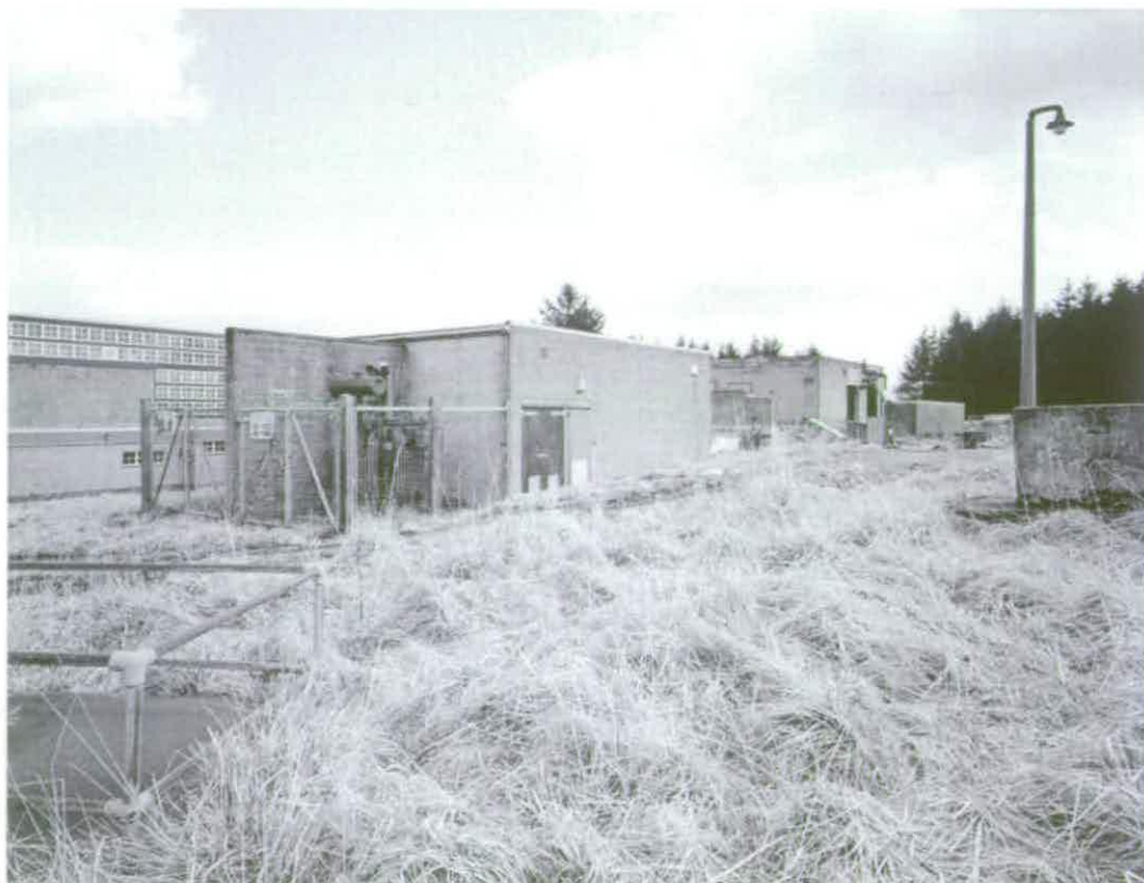
Figure 114 The LOX Evaporation Pit is visible in the foreground with the Sub-station and Transformer B7 behind © Crown copyright NMR (AA94/2938)
