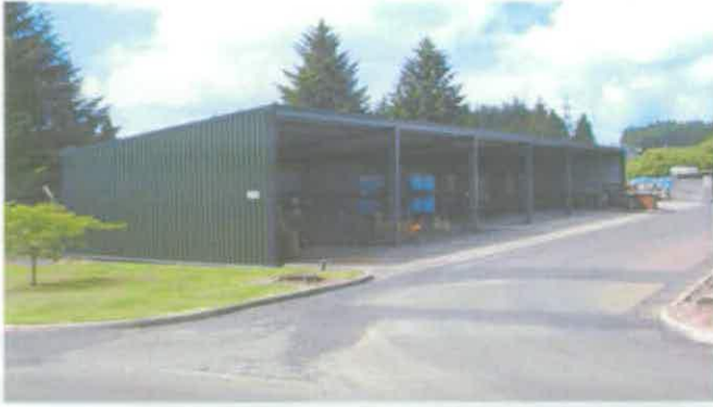
Figure 60 Modern steel framed garage F112 © English Heritage (AF00134/F112)
