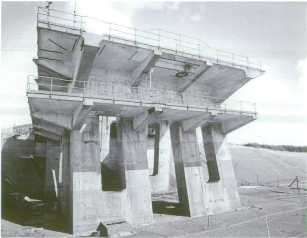
Figure 219 Thrust pad of the Missile Test Stand C3 © Crown copyright NMR (AA94/2028)
