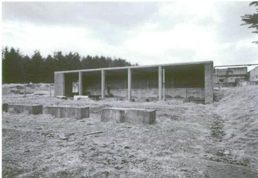
Figure 116 The High Pressure Gaseous Nitrogen Store B10 was open to the east. Blocks in front supported five horizontal gas cylinders © Crown copyright NMR (AA94/2939)
