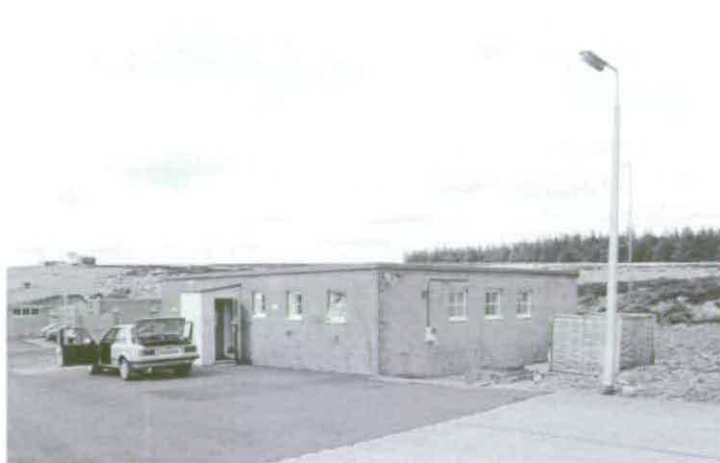
Figure 257 Staff Welfare Building C29.3 © Crown copyright NMR (AA94/2037)
