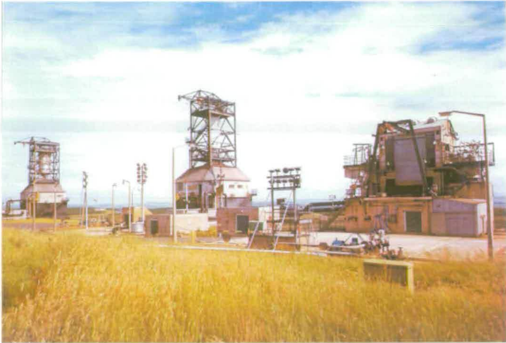
Figure 170 Contemporary photograph of Engine Test Stand A42 © Rolls-Royce plc
