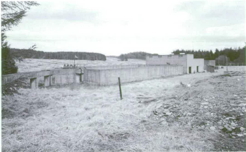
Figure 121 The main drainage conduit is supported on concrete stanchions as it approaches the Settling Tank B6 © Crown copyright NMR (AA94/2933)
