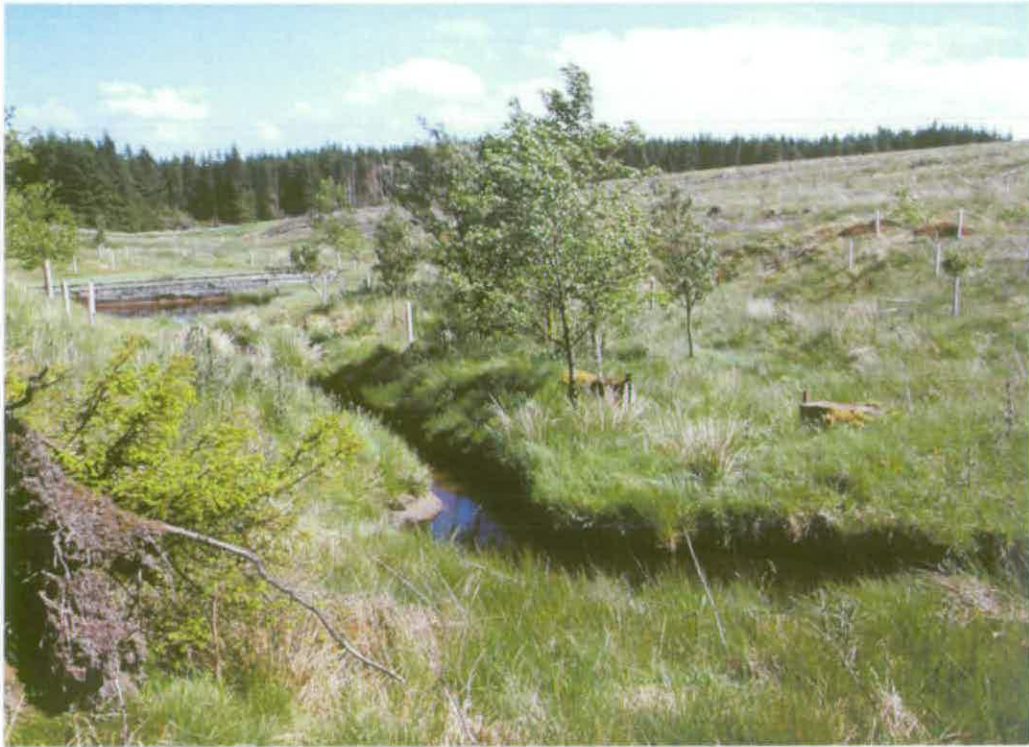
Figure 278 Work on the Underground Launcher Facility was started in the bottom of a valley at Whipper Slack © English Heritage (AF00134/launcher silo1)
