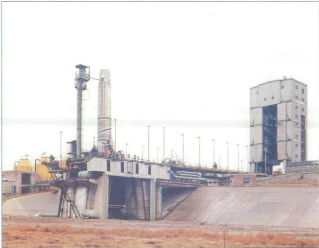
Figure 216 Missile Test Stand C3 showing a vehicle in position on the thrust pad and the Mobile Service Tower behind © Rolls-Royce plc
