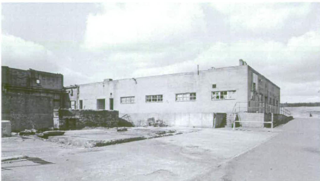
Figure 107 Workshop B1.3 looking north © Crown copyright NMR (AA94/1938)
