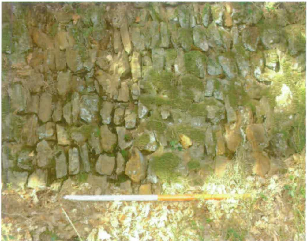
Figure 13. The western interior of building c, showing detail of the carefully constructed, battered wall.
