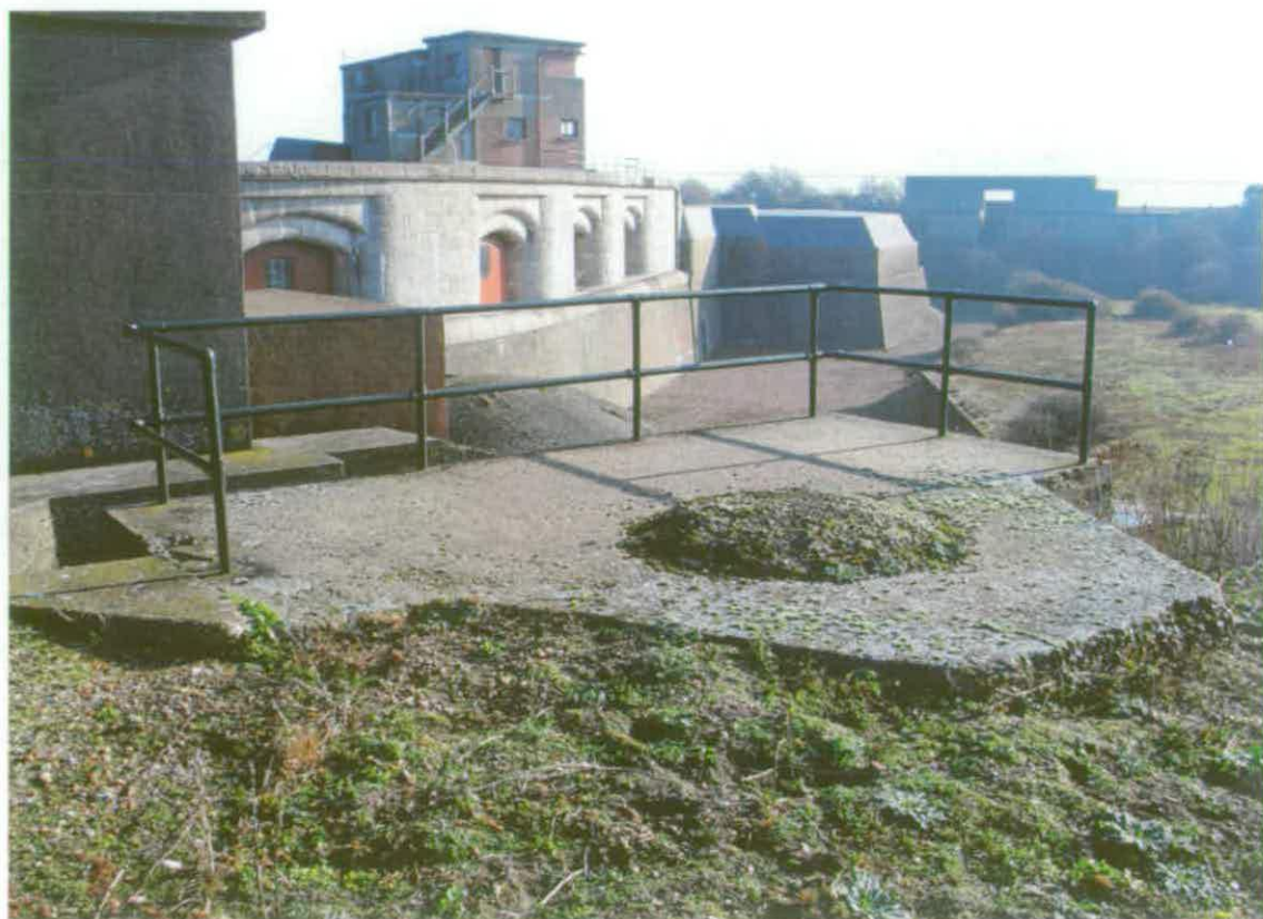
Figure 20 Photo of the open gun platform of no 2 6/12-pdr QF emplacement; Landguard Fort is in the background (Paul Pattison)
