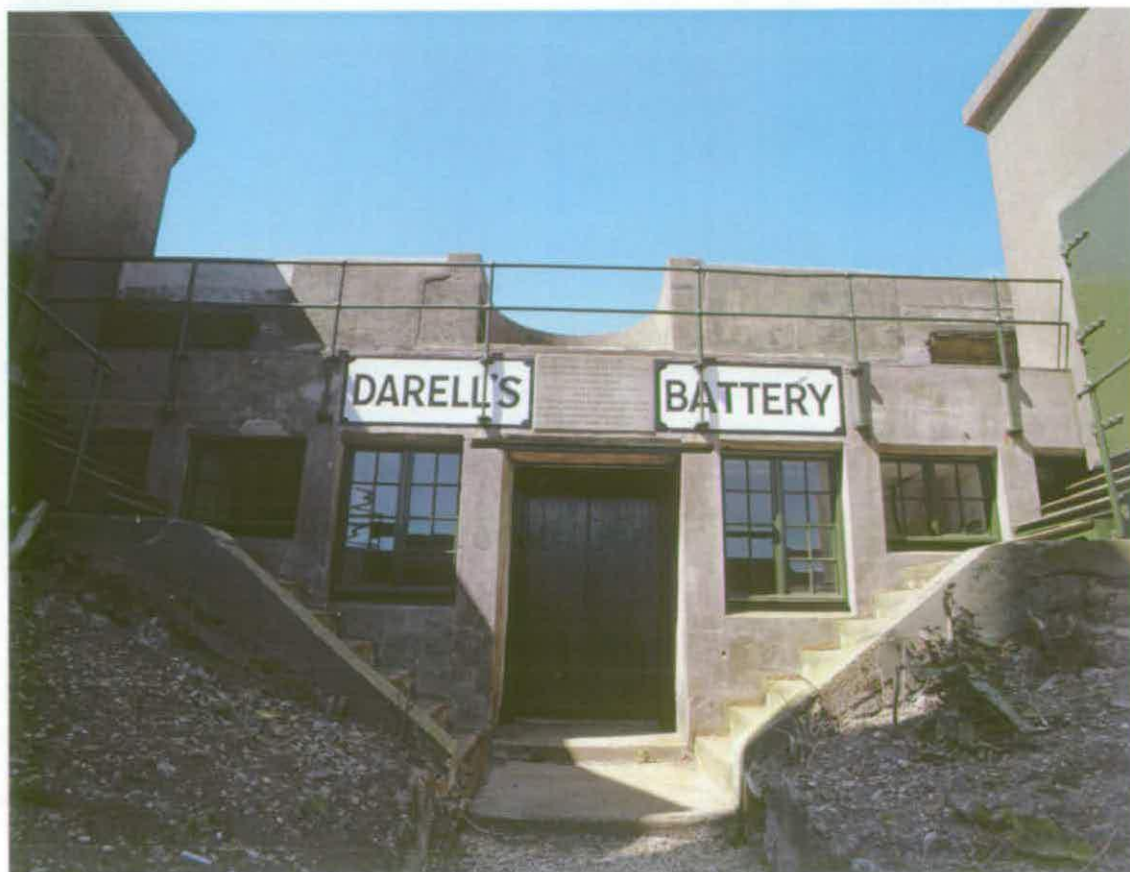
Figure 18 Photo of the entrance elevation to the shelter/Royal Artillery store of the 4.7-inch QF battery (NMR: AA046766)
