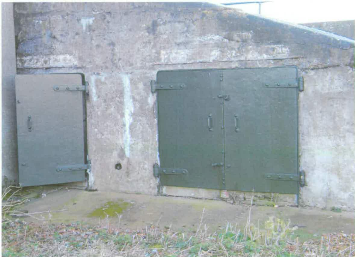
Figure 15 Photo of cartridge recesses in the right wing wall of the 4.7-inch QF battery (Paul Pattison)
