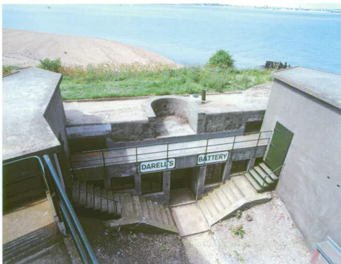
Figure 16 Photo looking down on the covered way and modified Battery Command Post of the 4.7-inch QF battery (NMR: AA046770)
