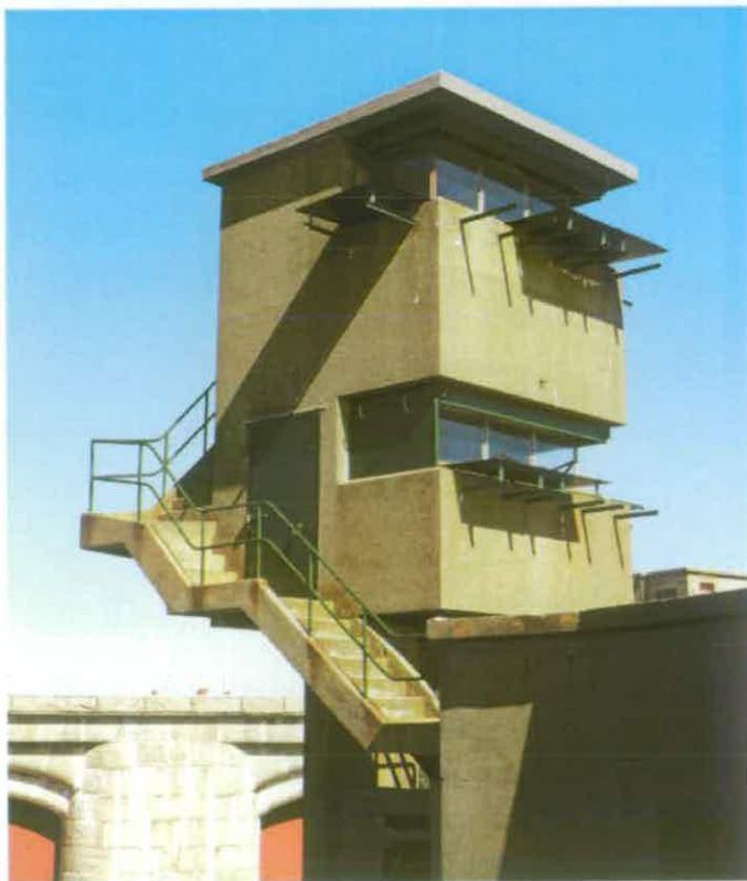
Figure 31 Photo from the west showing levels 3 and 4 of no 2 director sight tower, with its external staircase, observation windows and shutters (NMR: AA046786)
