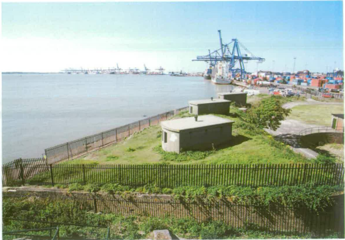
Figure 35 Photo looking north from Darell's Battery showing CASL nos 5, 6 and 7 (NMR: AA046727)
