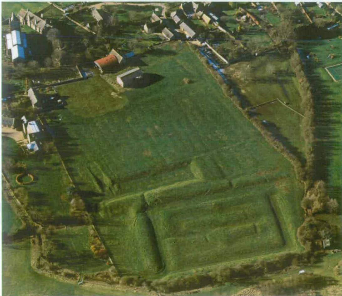
Figure 10– Aerial photograph from the south-east with the fishponds in the foreground, the Bede House is top left to the right of the church © English Heritage NMC SP 8797/03
