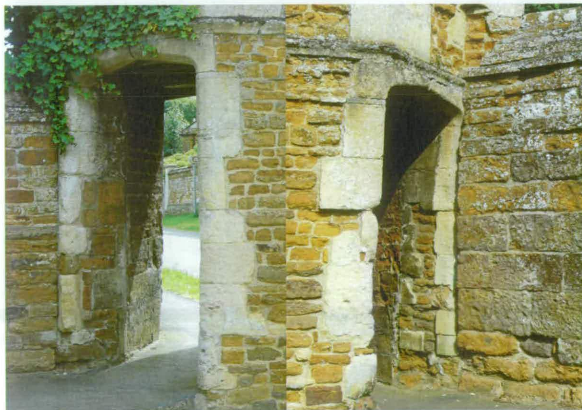
Figure 2 – The walls abutting the corner tower, that on Main Street to the left, on Church Lane to the right
