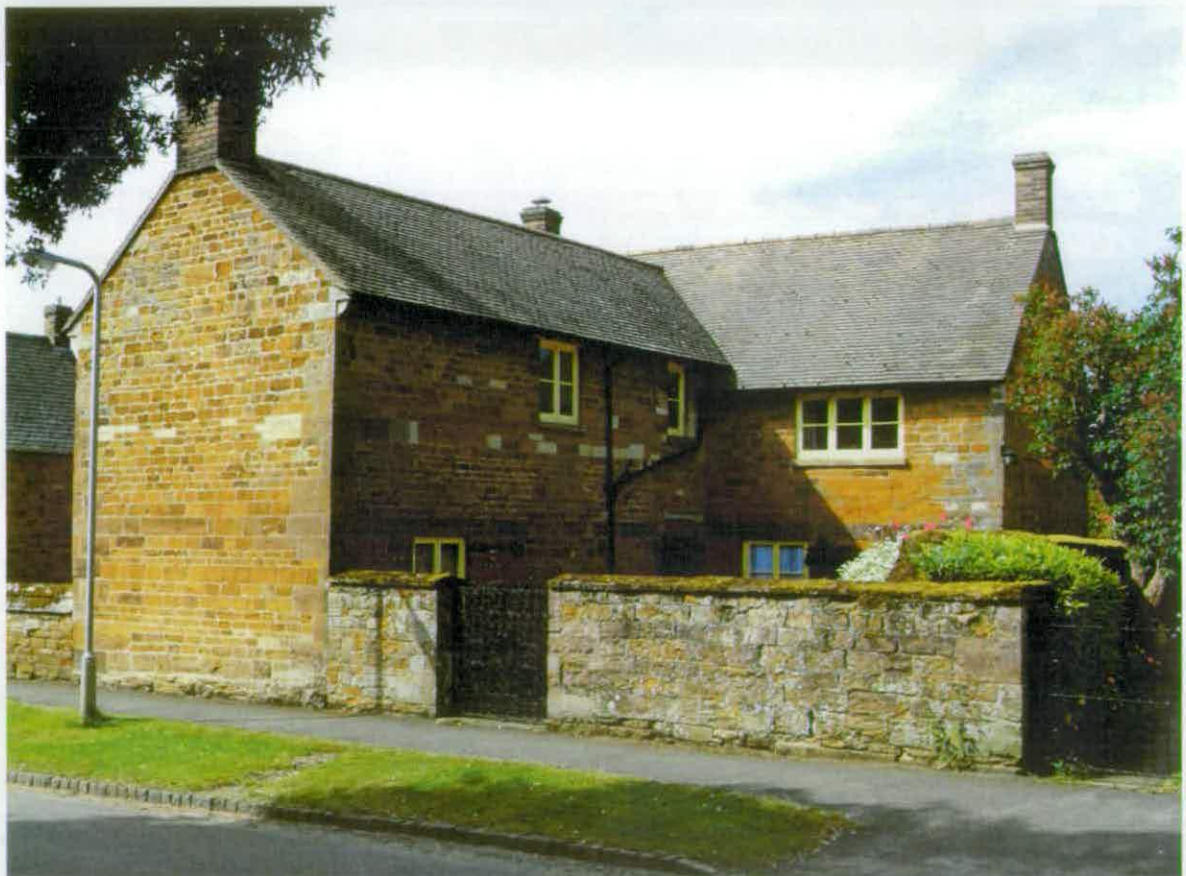
Figure 4 – An example of encroachment south of The Green, the front part of no 43 Main Street appears to be a later addition to the rear cross wing
