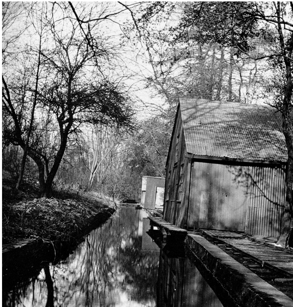
Figure 28. Western end of the corning house (probably in the late 1920s), from the south west. (NMR: AA035276, reproduced by permission of David Willacy)
