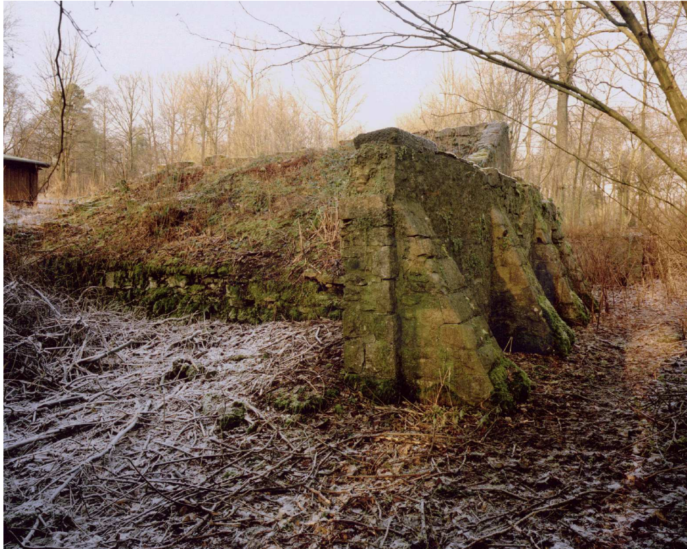
Figure 27. Blast bank between first powder press house and corning house , from the south east. (NMR: AA012916)
