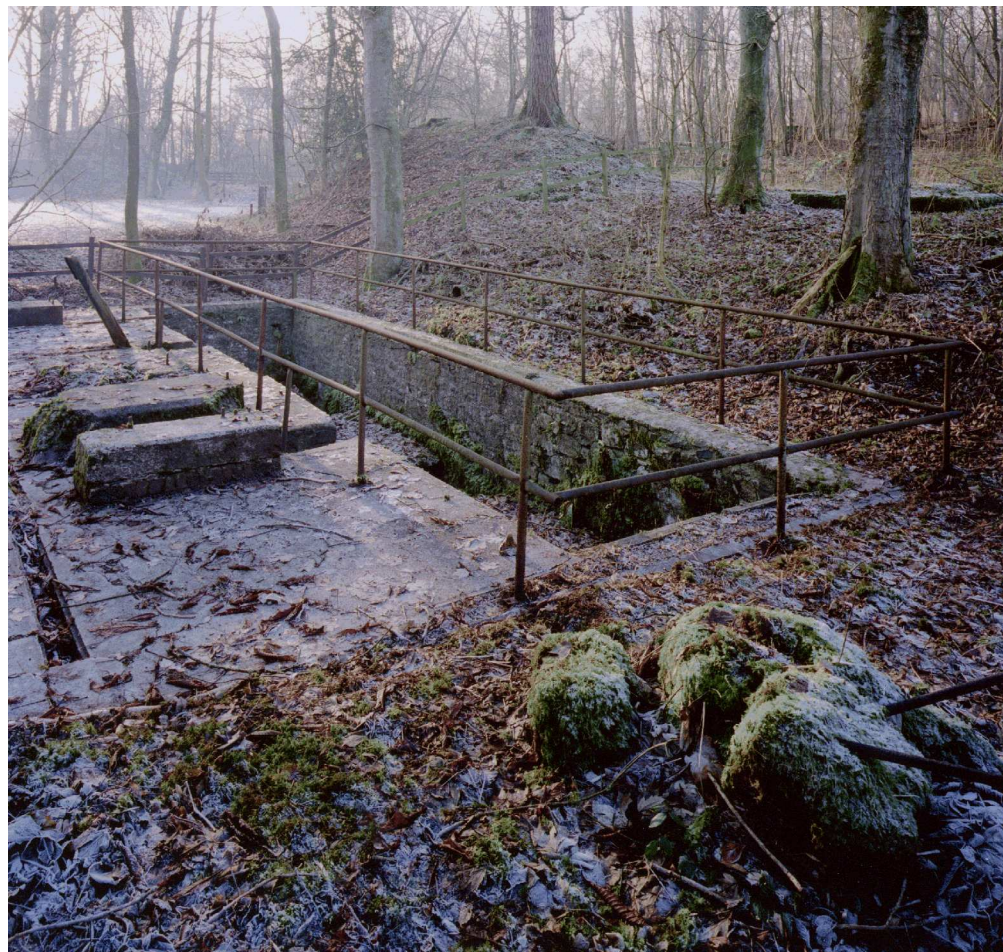
Figure 36. Cartridge press pump house and near-by blast bank from the north east. (NMR: AA012904)
