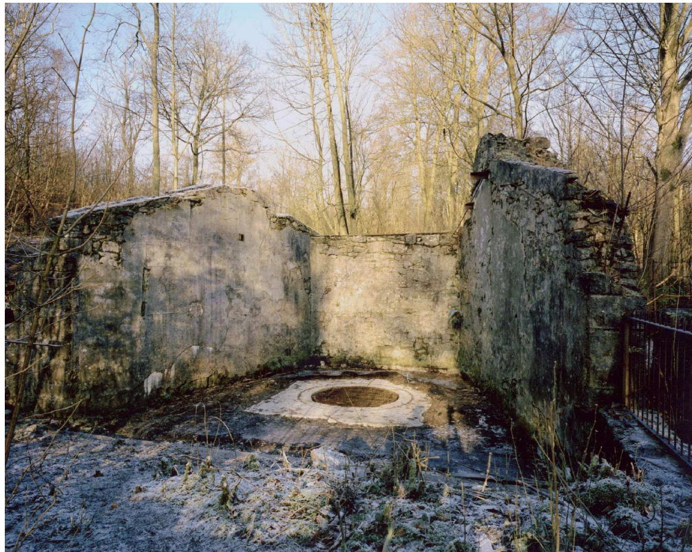
Figure 20. Incorporating mill 3, general view from south. (NMR: AA012870)
