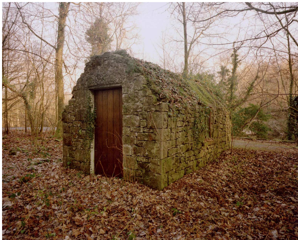
Figure 34. The electric motor house from the west. (NMR: AA012927)
