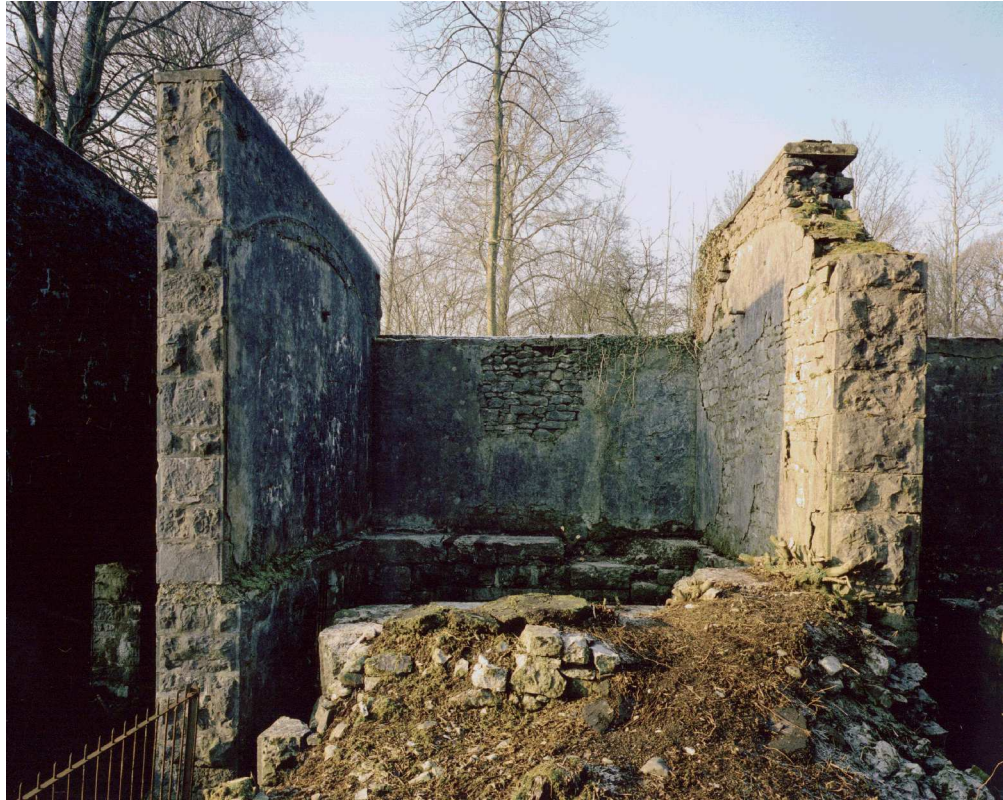
Figure 26. Incorporating mill 8 from the east. (NMR: AA012895)
