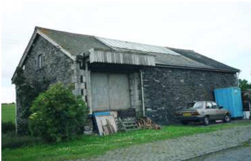
Figure 52. The gunpowder warehouse at Hincaster Junction, from the east. (NMR: DP001584, reproduced by permission of Christopher Dunn)
