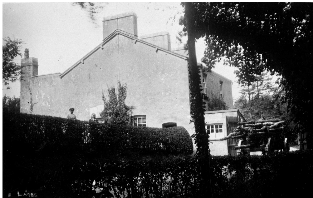
Figure 42. The gate house and weighbridge office (probably in the late 19th or very early 20th century) from the south. (NMR: AA035270, reproduced by permission of David Willacy)
