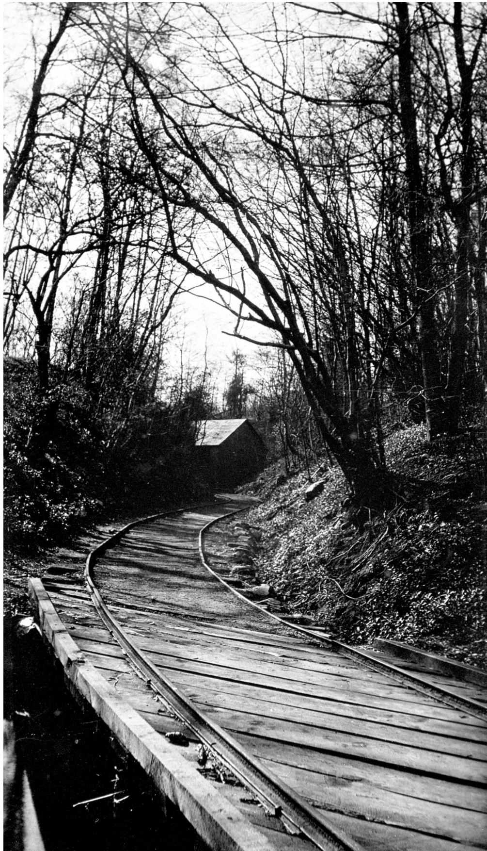
Figure 35. Cartridge compressing house 2 and the tramway (probably in the late 1920s) from the east. (NMR: AA035275, reproduced by permission of David Willacy)
