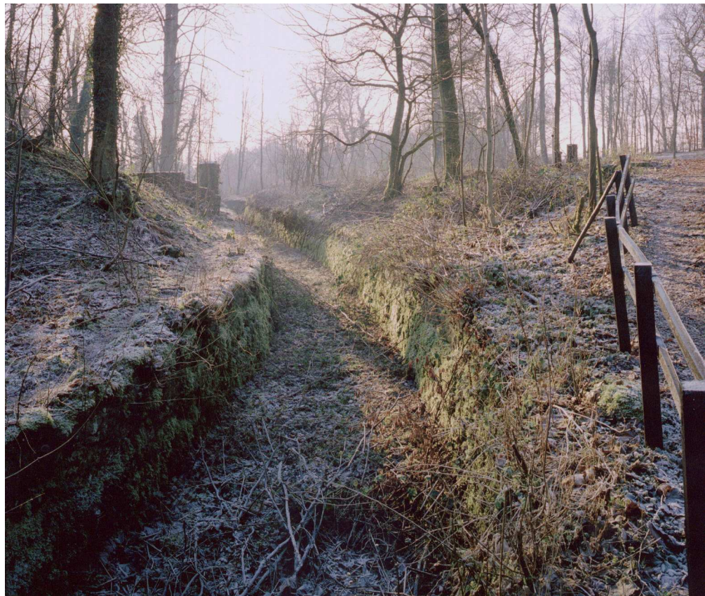
Figure 12. The main leat looking south from near the incorporating mills (blast walls of green charge house visible above on left). (NMR: AA012871)
