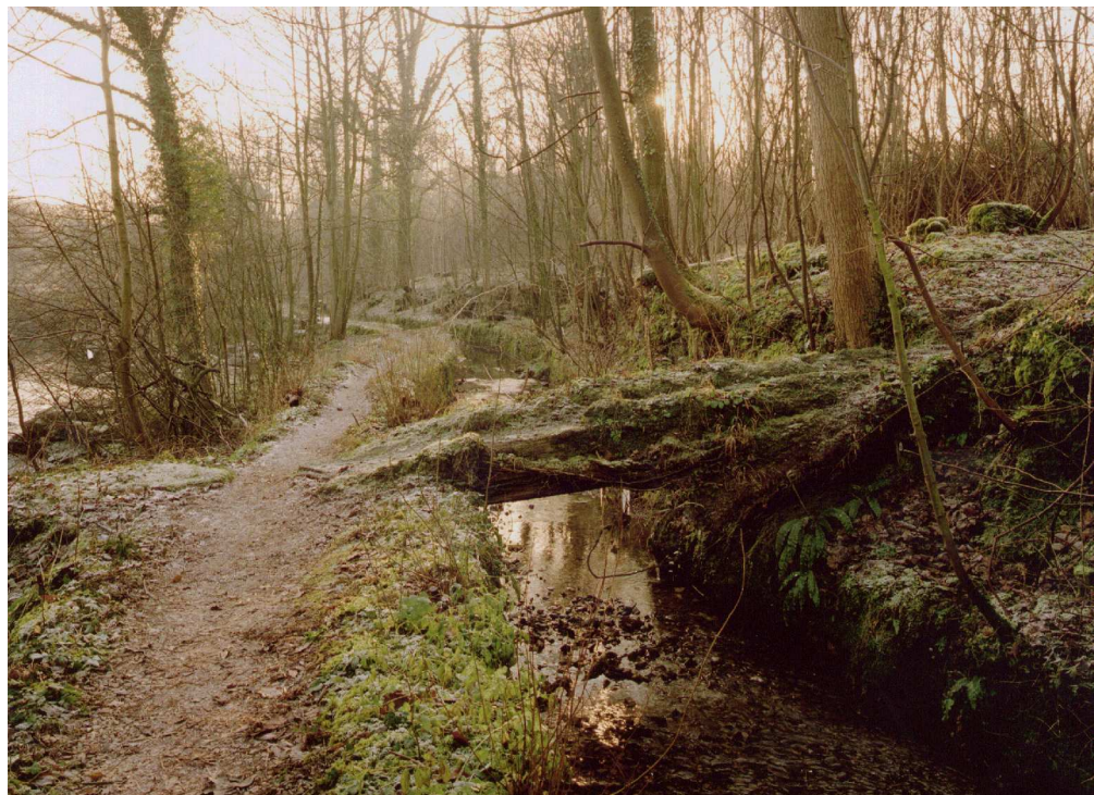
Figure 14. The aqueduct and main leat from the north. (NMR: AA012923)
