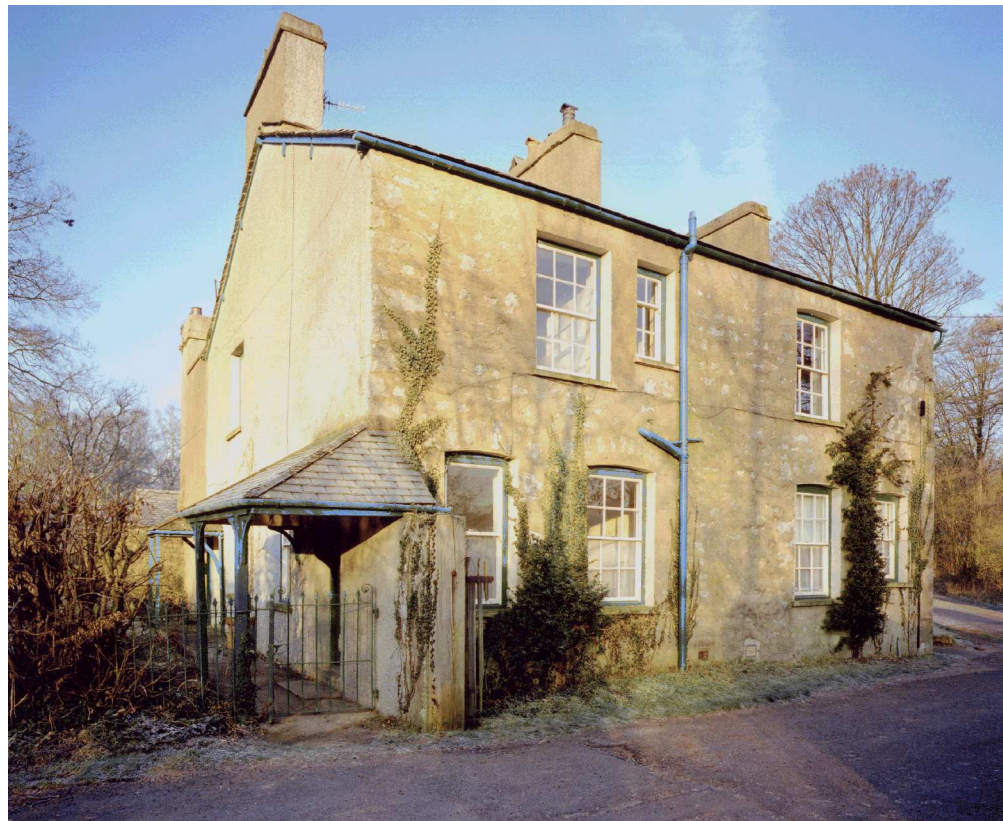
Figure 41. The gate house from the south east. (NMR: AA012835)
