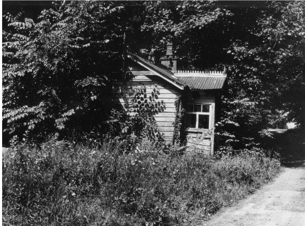
Figure 38. The proofing house in 1977, from the south. (Reproduced by permission of the National Trust)
