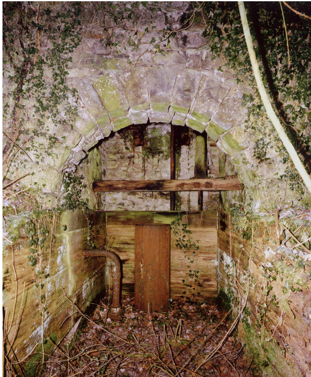
Figure 45. Detail of the new saw mill showing the arched opening from the main leat into the turbine house which served the cooperage, from the north east. (NMR: AA012853)
