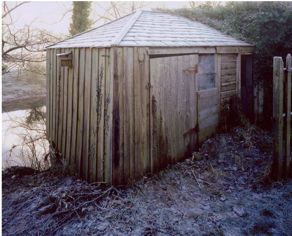
Figure 40. The clocking-in shed from the north west. (NMR: AA012833)
