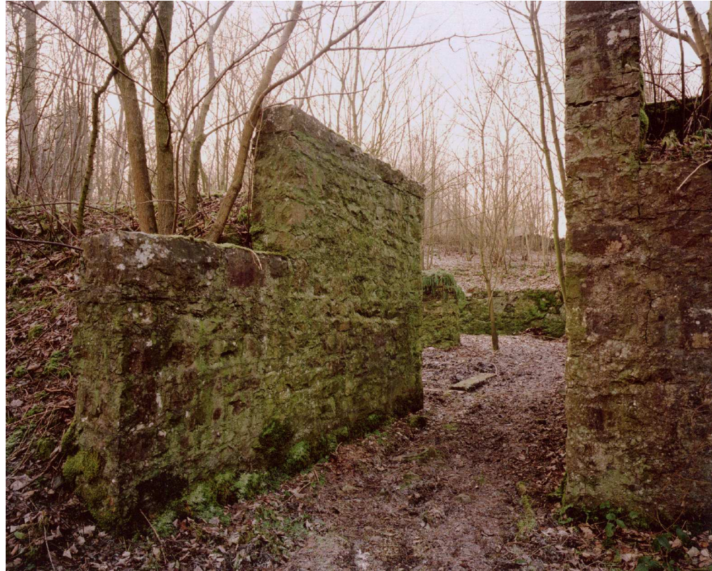
Figure 33. The entrance to the new stove house, from the east. (NMR: AA012910)
