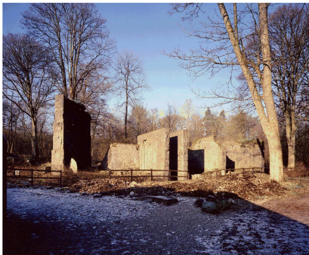
Figure 24. Blast wall (left) and incorporating mills 7,8 and 9 from the south east. (NMR: AA 012873)
