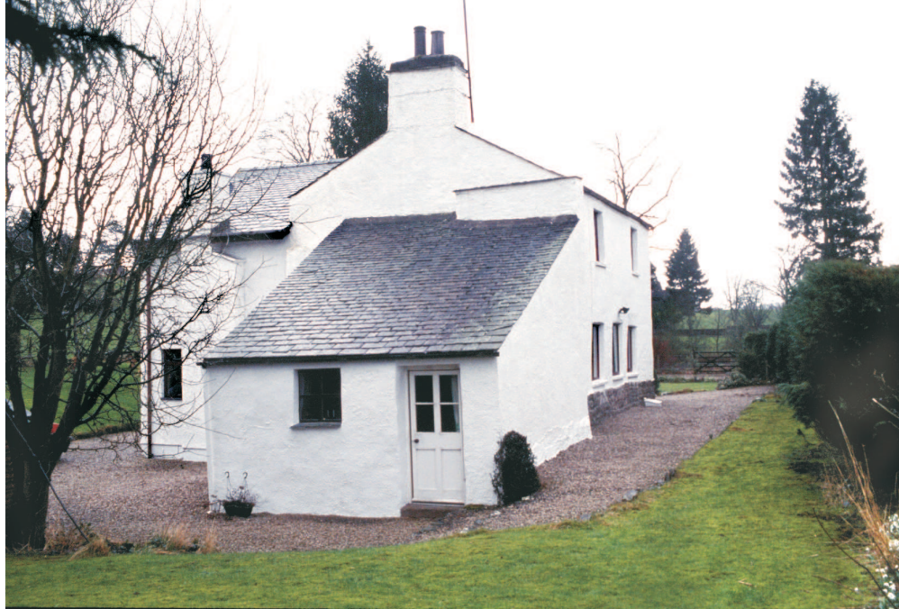
Figure 12. 'Garden Cottage' from the north, showing the northern annex which probably incorporates the steam-boiler house
