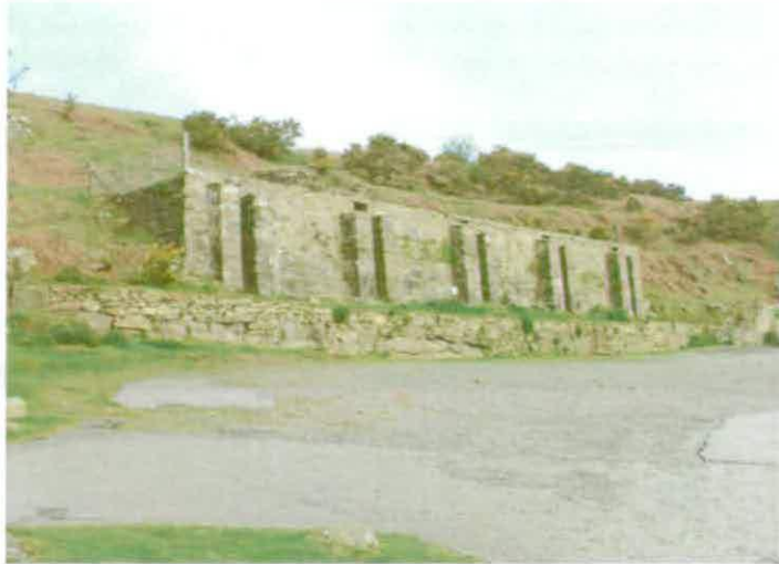
Plate 7. The thickening tank and the site of the drying pan, now used as a car park
