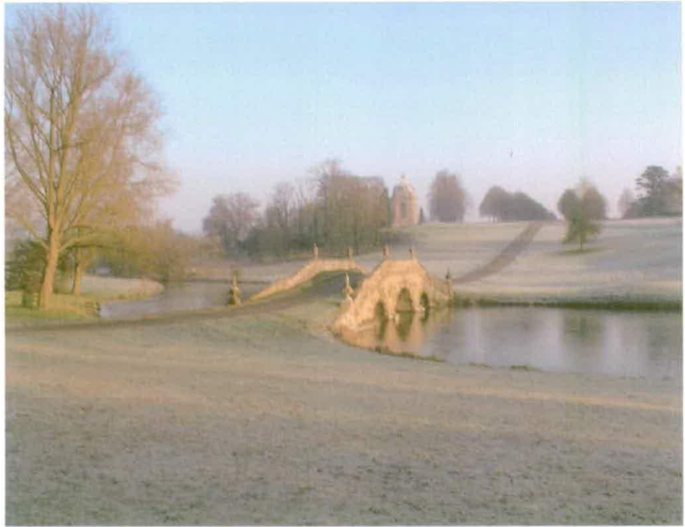
Frontispiece: Oxford Bridge and the West Boycott Pavilion
