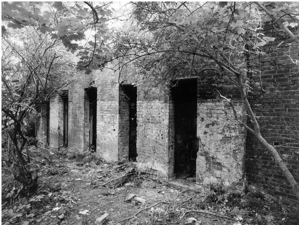
Figure 32 The Guard House Privies in 1999 (NMR: AA99/01924 © English Heritage)
