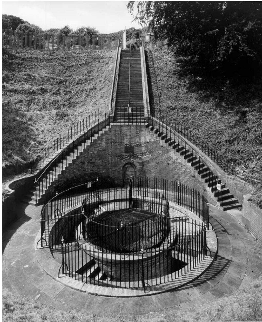
Figure 15 The top of the Grand Shaft in 1998, showing the stairs descending the bowl-like depression from the Parade Ground, the railings and the entrances to the three staircases at the top of the shaft (NMR: AA008568 Crown Copyright 1999)
