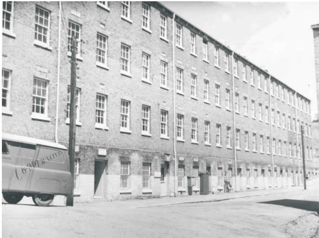
Figure 19 The Soldiers' Quarters (Range B), shortly before demolition. The size and sombre nature of the barracks is apparent (d08611 © Dover Museum)
