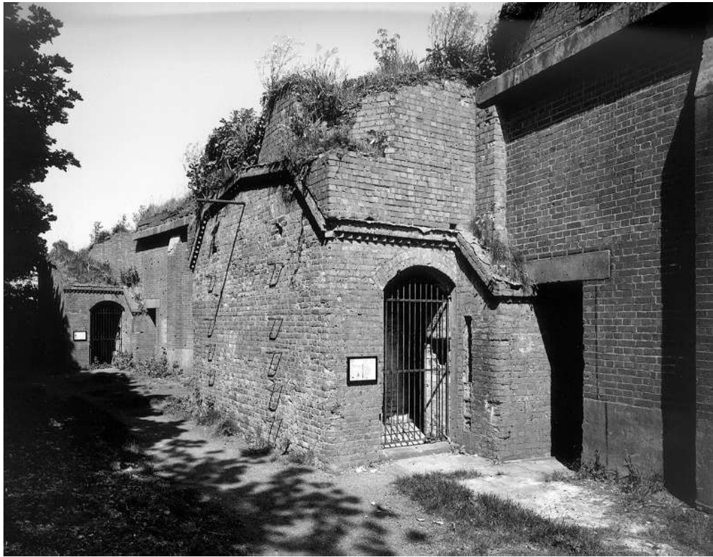
Figure 9 St Martins Battery: rear of the battery, showing original porch to cartridge store E and shell store D (extract from NMR: AA 99 09714 © Crown Copyright 1998)
