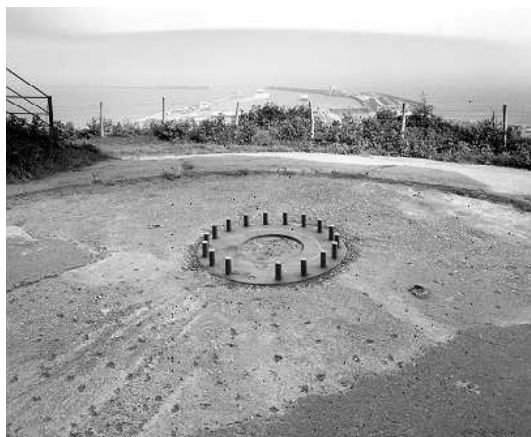
Figure 16 Western Heights Battery: steel plate and securing bolts for the gun holdfast, no I gun (NMR: AA 99 09710 © Crown Copyright 1998)
