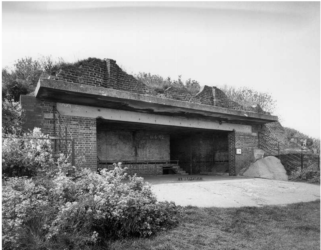
Figure 15 Western Heights Battery: front elevation of 6-inch gunhouse. Note the undulating parapet, designed to break up the outline of the battery from a distance (NMR: AA 99 09707 © Crown Copyright 1998)
