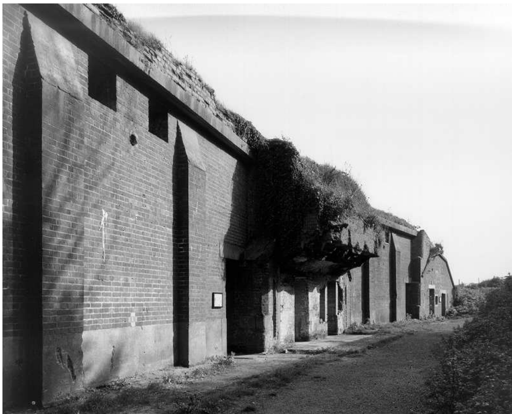
Figure 14 Western Heights Battery: 6-inch gunhouses, rear elevation (NMR: AA 99 09713 © Crown Copyright 1998)
