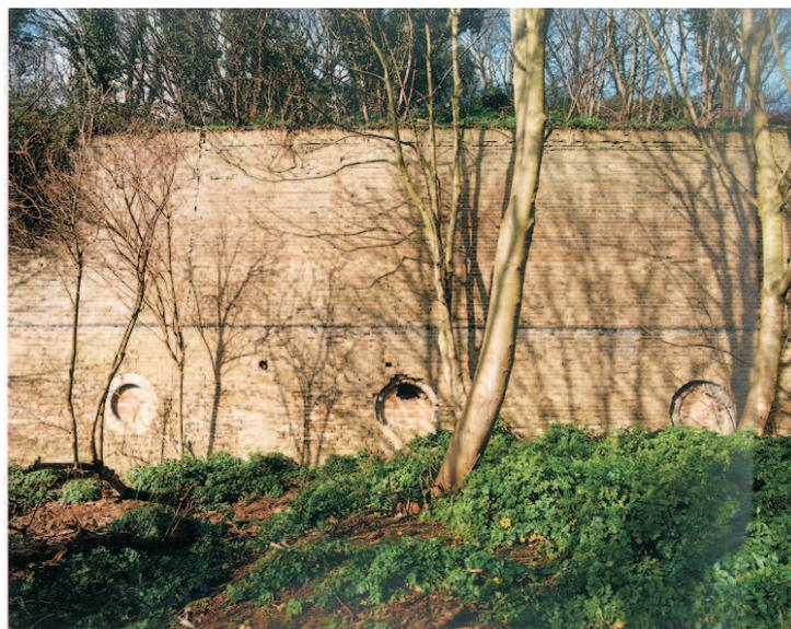
The counterscarp survives for the southern half of the ditch. It comprises an unrevetted chalk face, except near the cliff edge where there is a short section of faced flint retaining wall, incorporating two blind alcoves finished with round relieving arches in brick. This
