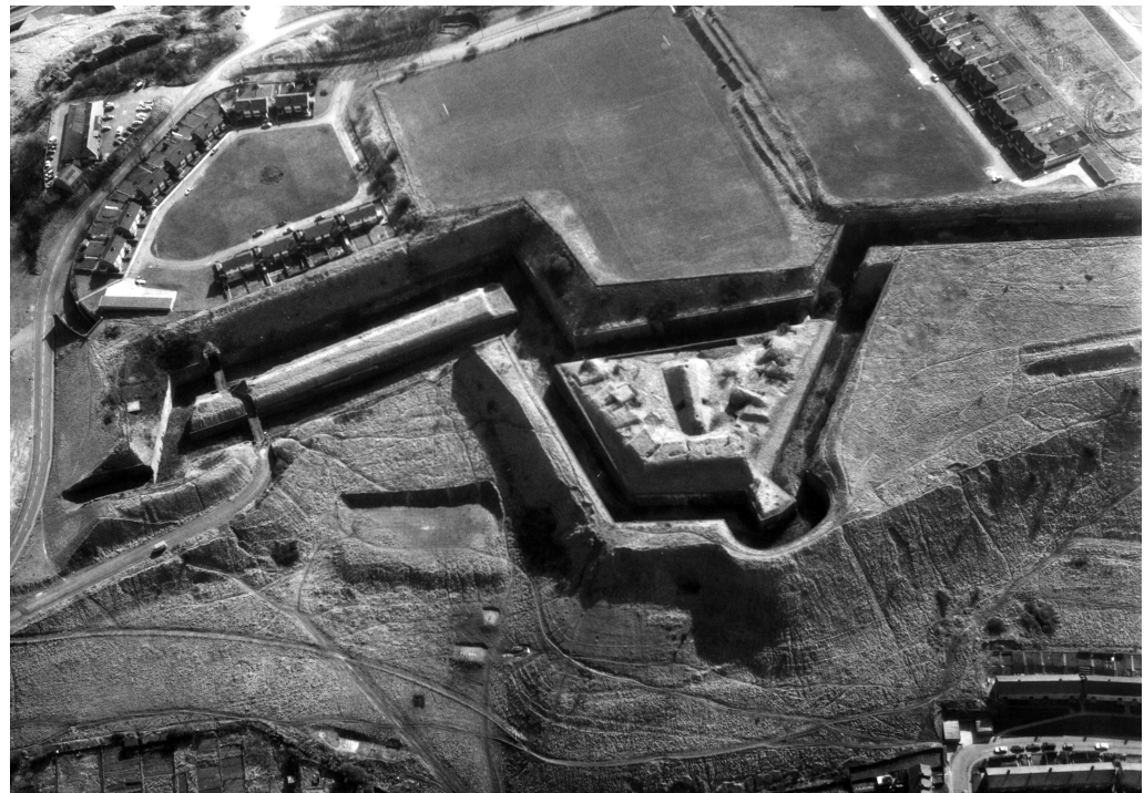
Figure 16 North Centre and Detached Bastions, from the air in 1978 (NMR: TR3040/4/147 © Crown Copyright)
