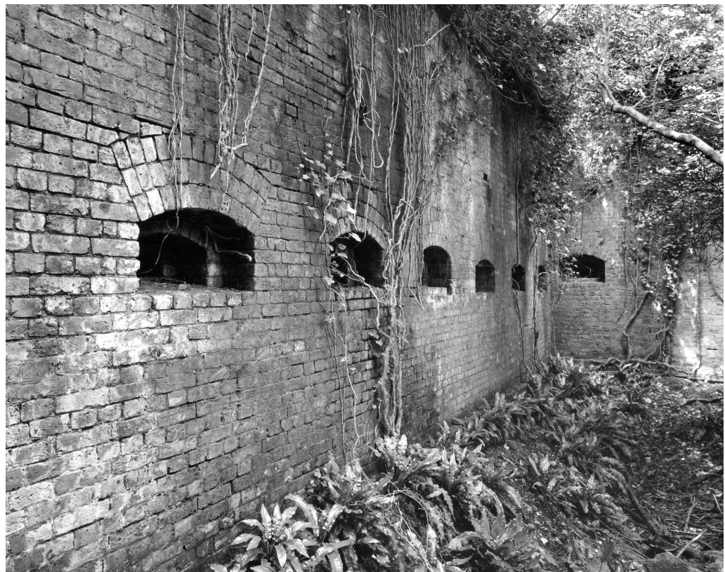
Figure 17 Detached Bastion; photo of the south caponier, east face exterior, showing horizontal musket loopholes (NMR: AA008604 © Crown Copyright 1998)
