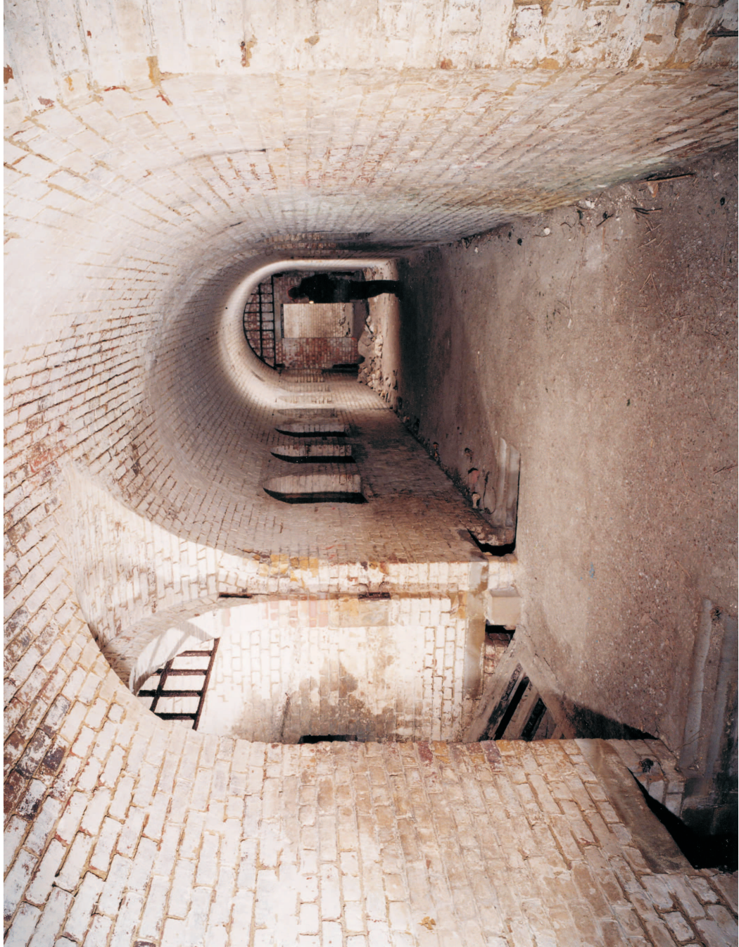
Figure 19a Detached Bastion; the interior of the south caponier, looking south; at left is the entrance to a ramp leading up to the terreplein (NMR: BB 029680 © English Heritage 2001)
