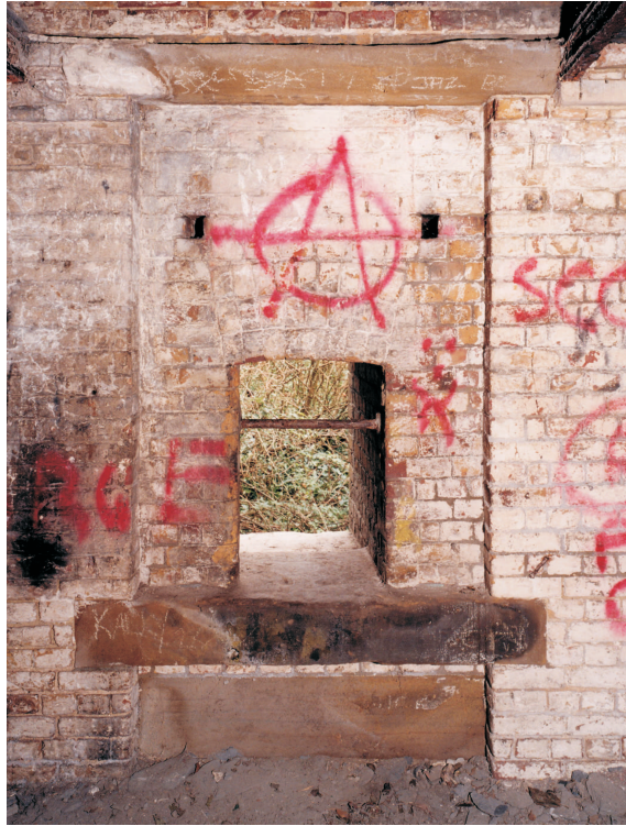
Figure 34 Detached Bastion; a carronade embrasure and mounting in the west flank wall of the north-west caponier (NMR: BB 029682 © English Heritage 2001)
