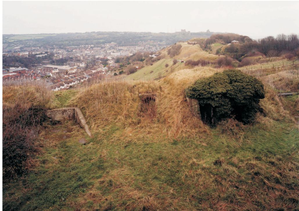
Figure 21 Detached Bastion; photo of the east terreplein, showing emplacement no II (at left), for 7-inch RBL gun, c 1890, together with its shell recess (centre) and the entrances to the artillery store and east gallery (NMR: BB 029679) © English
