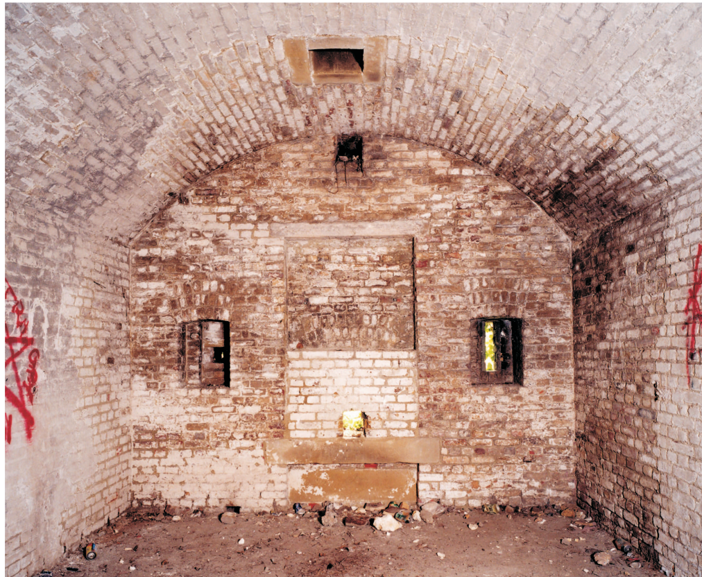
Figure 12 North Centre Bastion; photo of one of three gunrooms in the east gallery, showing the central carronade embrasure flanked by musket loops and smoke vents in the vault (NMR: BB 029684 © Crown Copyright 1998)
