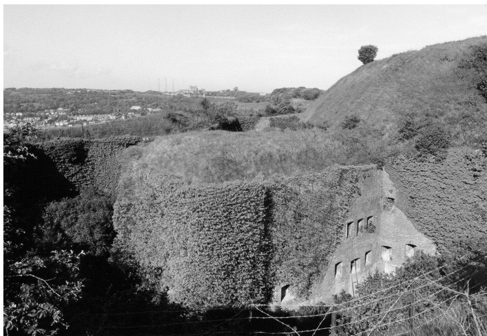
Figure 32 Detached Bastion; external view of the NW caponier, from the west, showing musket loops and carronade embrasures (NMR: AA008621 © Crown Copyright 1998)
