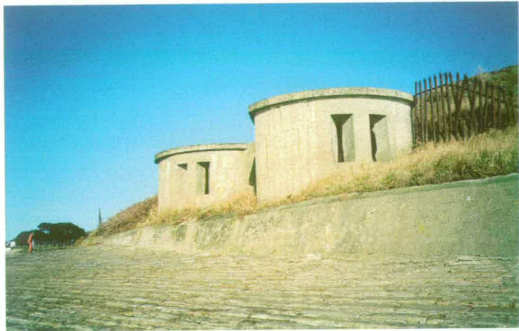
Figure 38 Photograph of two CASLs, built for the Cornwallis Battery; view from the promenade
