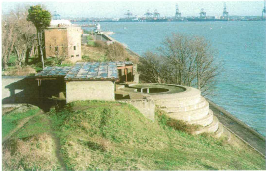
Figure 34 Photograph of the 6-inch Mark VII emplacement which replaced the 1901 6-inch BL emplacement; view from south showing the terraced concrete buttressing
