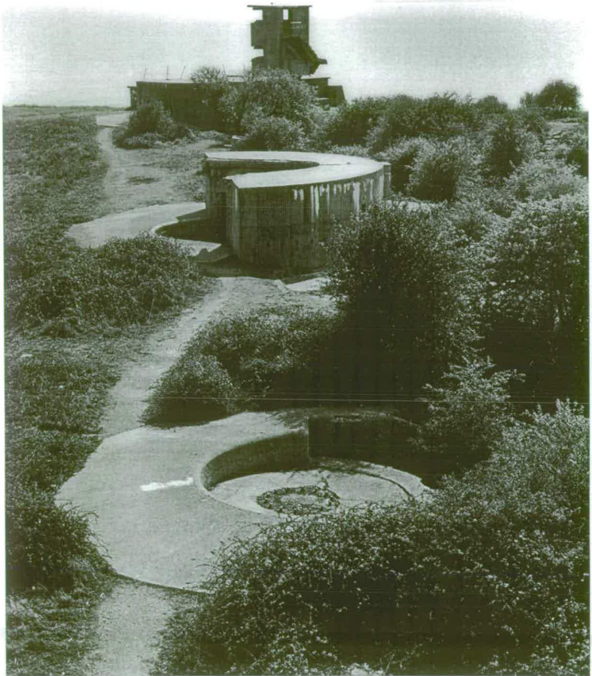
Beacon Hill Fort, Harwich; photograph showing three of the main gun emplacements, demonstrating different phases in the Fort's history. Foreground: 1892 4.7-inch quick-firing gun emplacement. Middle: 1890 6-inch breech-loading gun emplacement, replaced around 1904 by a 6-inch Mark VII emplacement, with Second World War casemate over. Background: 1941 Cornwallis Battery for Twin 6-pounder guns (NMR: BB97/5431).
