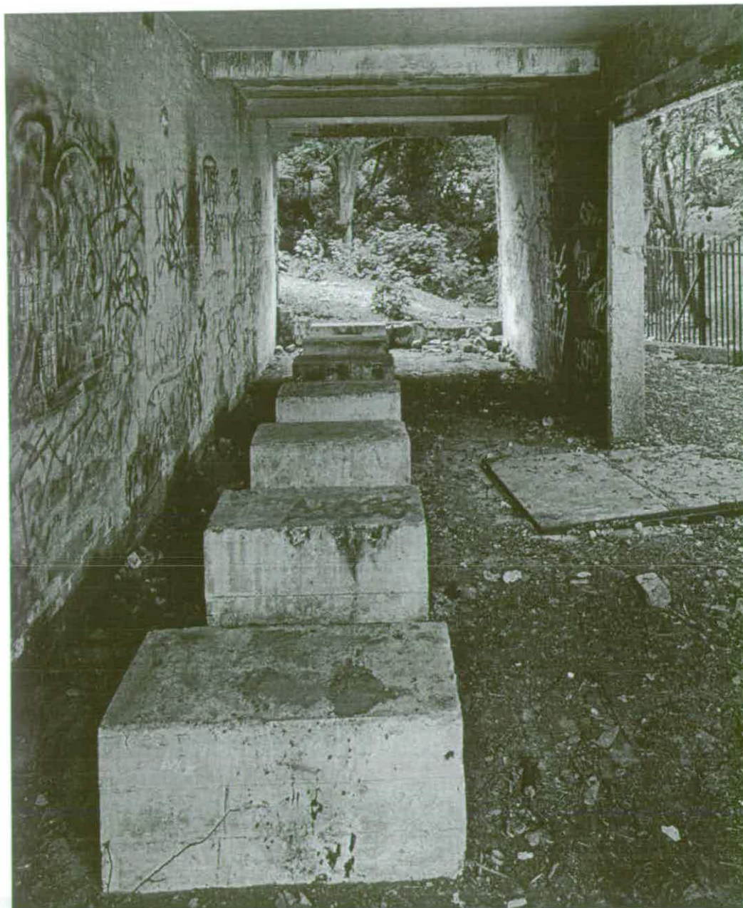
Figure 33 Photograph of the oil store; interior showing supports for the oil tanks (NMR: BB97/5462)
