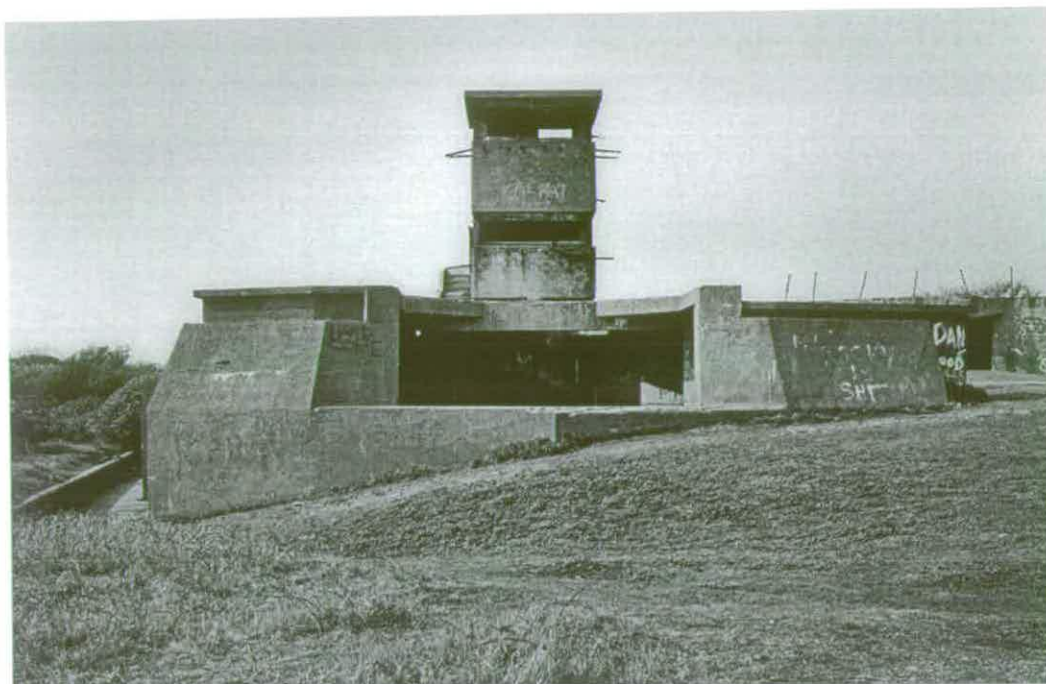
Figure 36 Photograph of the Cornwallis Battery showing the emplacement and its BOP to the rear; view from the south-east (NMR: BB97/5383)
