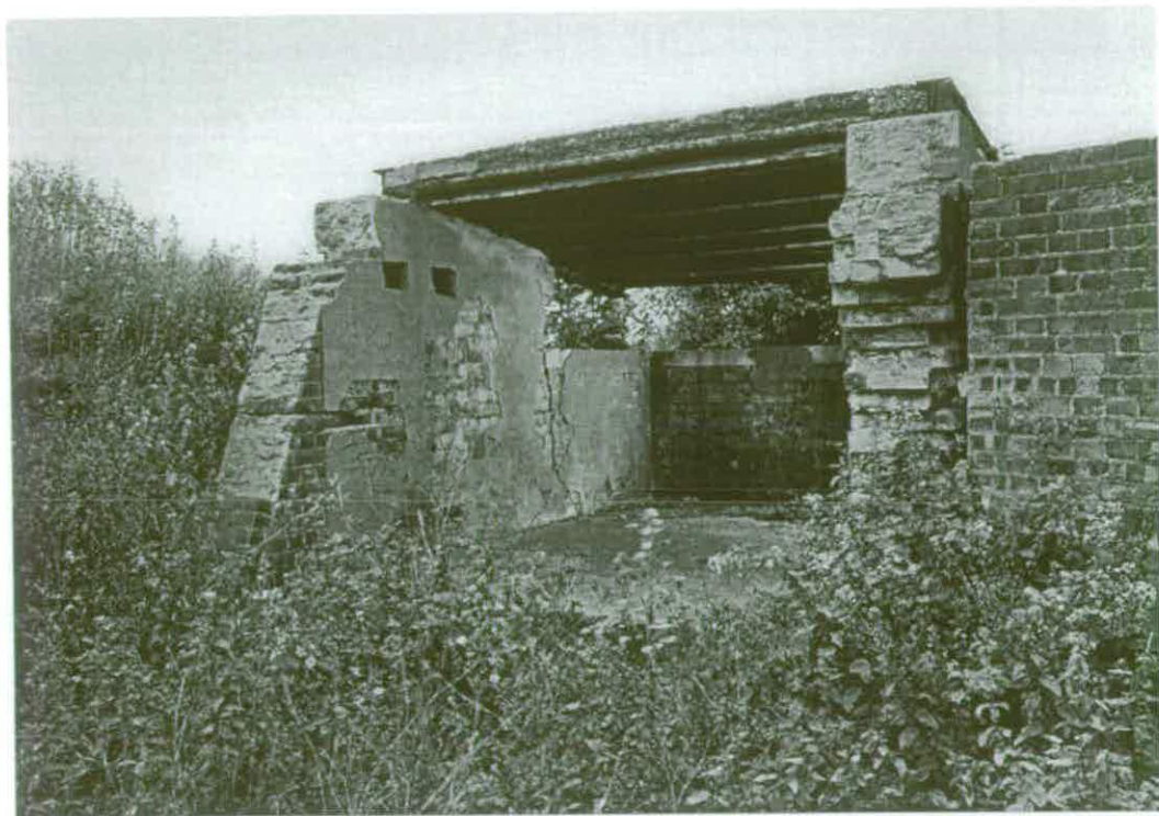
Figure 45 Photograph of a PF cell; view from the west showing the rear of the cell and the slit embrasure to the front (NMR: BB97/5465)
