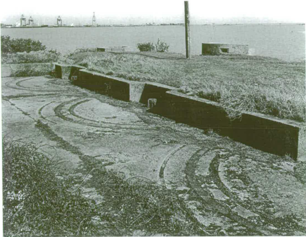
Figure 23 Photograph of the 1894 practice battery showing racers and gun pivots (NMR: BB97/5406)
