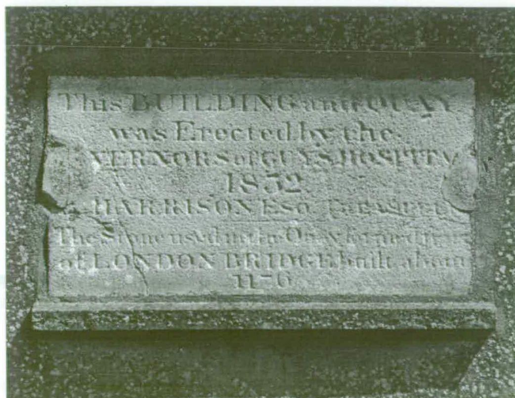
Figure 2: Limestone plaque recording the building of Beaumont Quay in 1832 (NMR AA96/5750)
