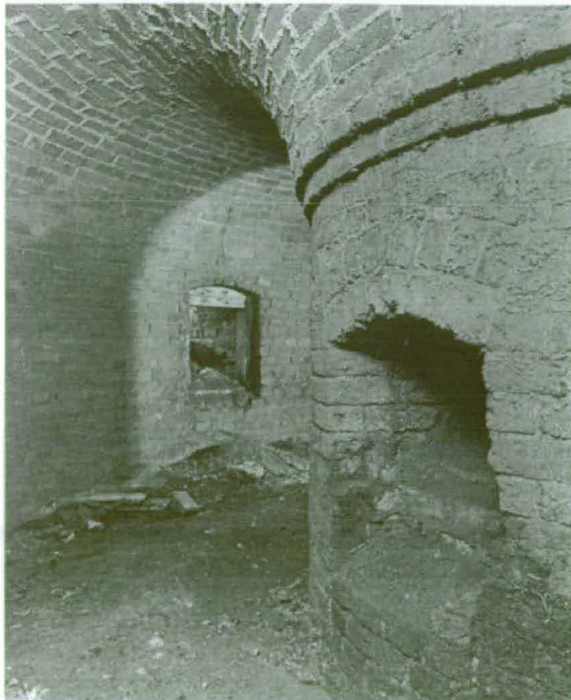
Figure 13: Beaumont Quay, interior of the limekiln with vent (centre left) and draw hole (right foreground) (NMR AA96/5758)
