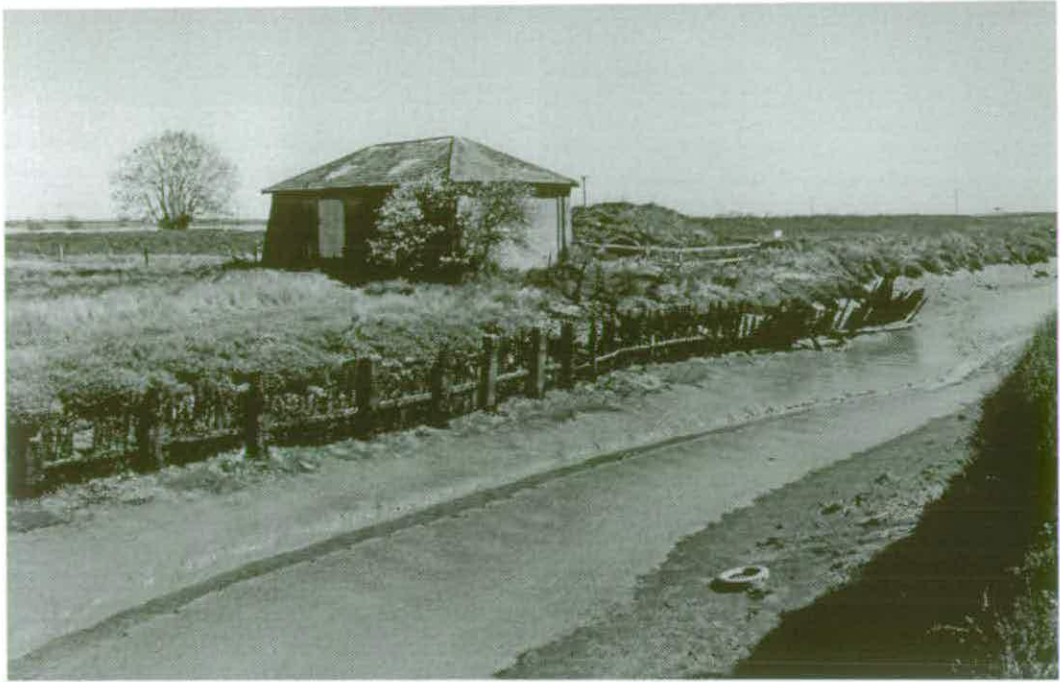
Figure 12: Beaumont Quay, store building and limekiln from the south-west (NMR AA96/5745)
