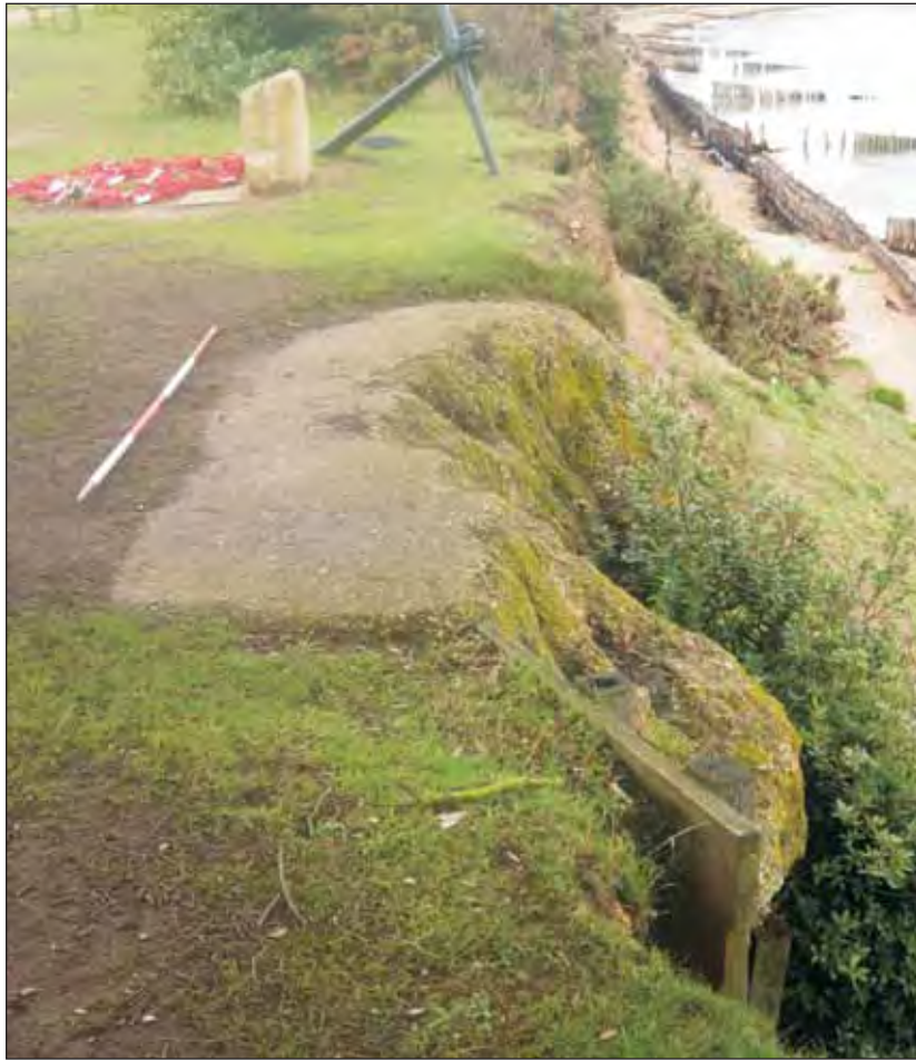
Plate D11: WA4152 . Remains of a WWII concrete structure, eroded from the top of the cliff at Lepe
