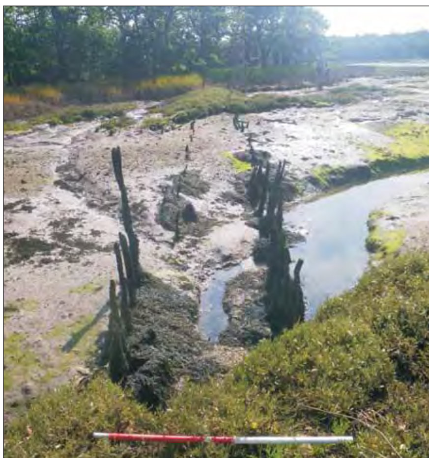
Plate D8: WA4083 . Bridge across an inlet on the Beaulieu River
