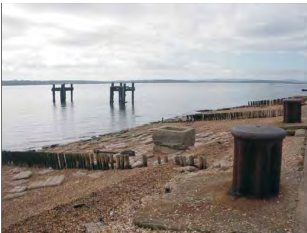
Plate D10: WA4157 & WA4159 . Two offshore WWII 'Dolphins' along with concrete hardening mats and bollards along the coast at Lepe
