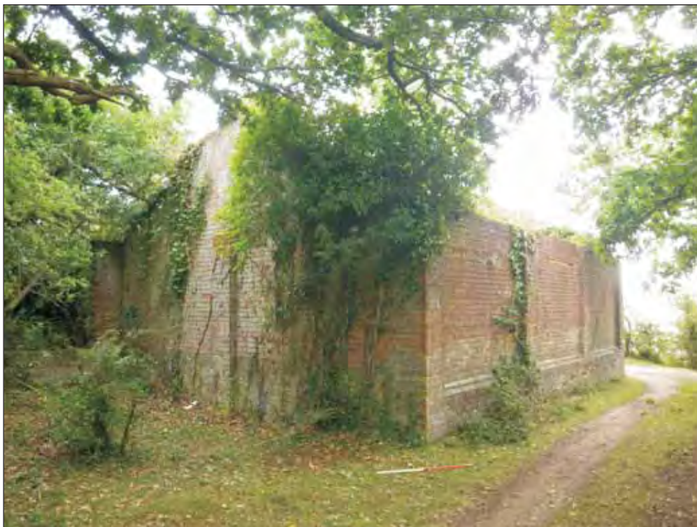
Plate C3: WA3033 . Standing remains of an 18th/19th century brickworks site at Pitts Deep
