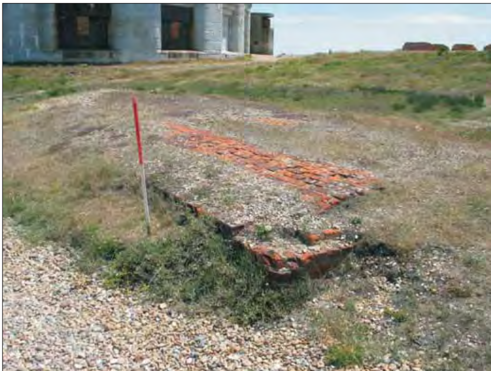
Plate B13: WA2064 . Red brick culvert, with adjacent red-brick structure, to the west of the castle on Hurst Spit
