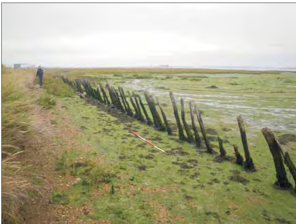
Plate E6: WA5029 . Calshot timber revetment
