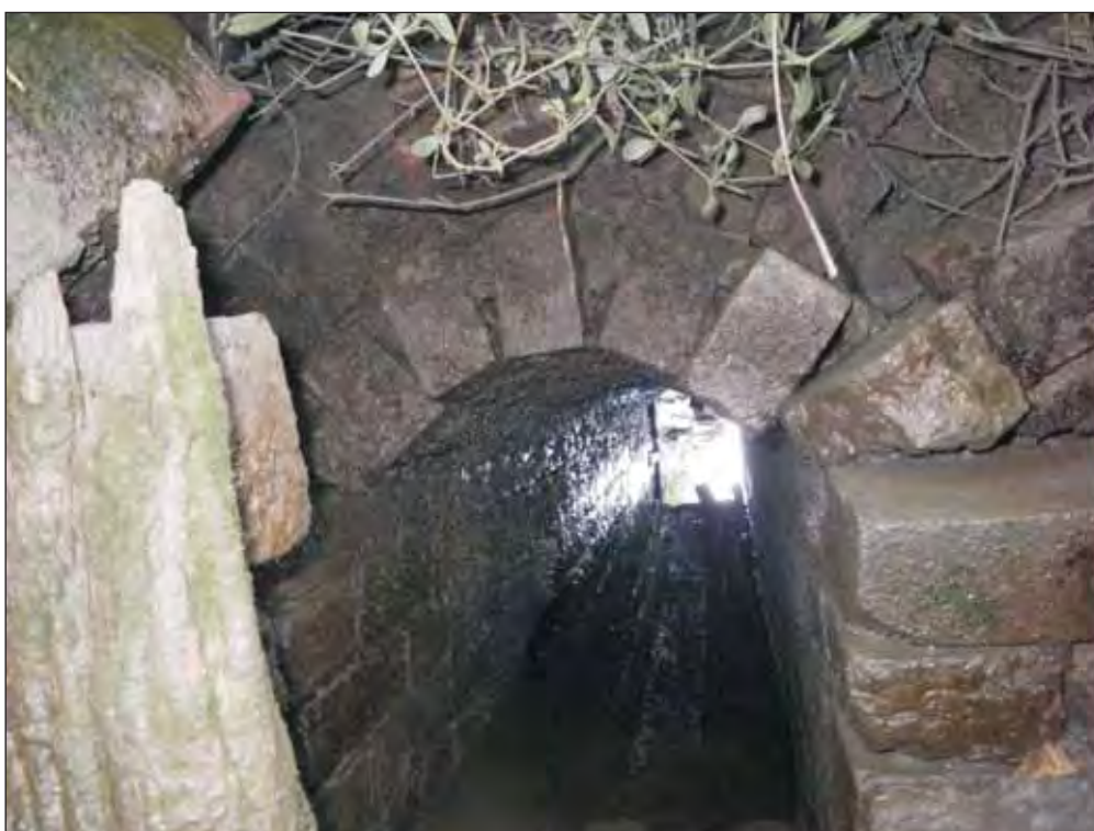
Plate E4: WA5007 . Langdown brick culvert
