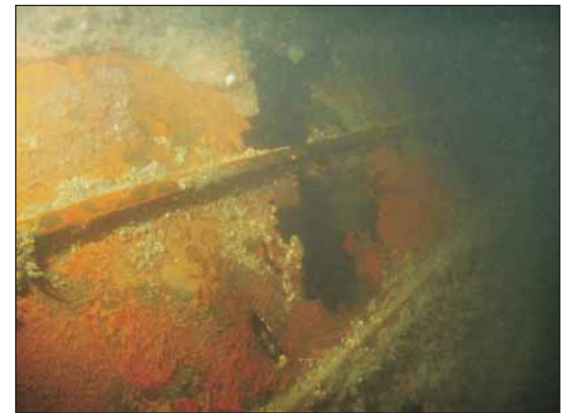
F: Horizontal treads on ramp door
