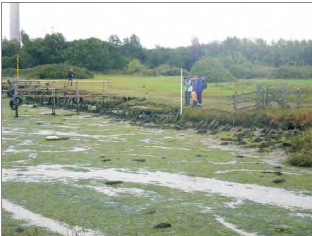
Plate E5: WA5045 . Ashlett timber revetment
