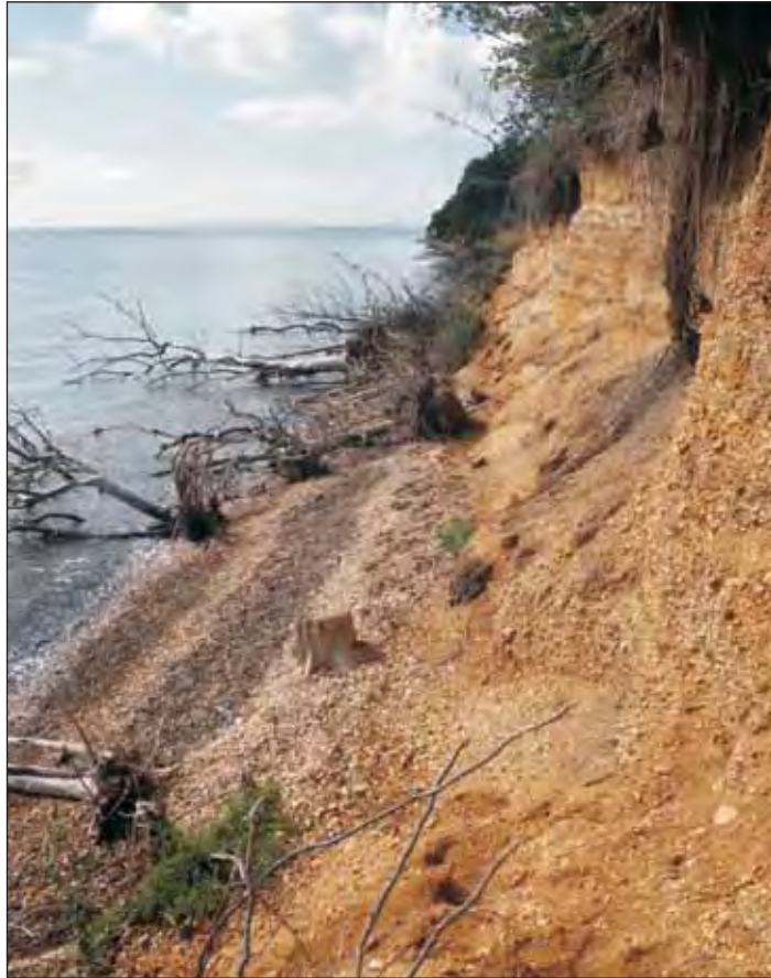
Plate D1: Section 8.1.6. Evidence of coastal erosion at Stanswood Bay
