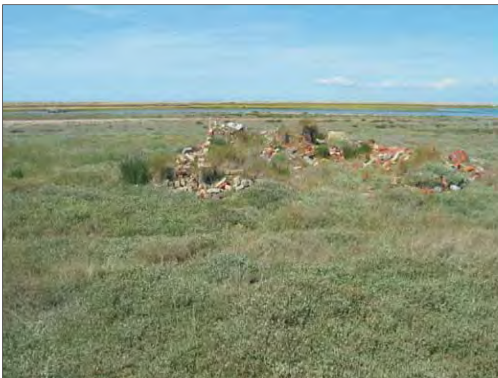
Plate B16: WA2089 . Remains of a derelict cottage to the north of the castle on Hurst Spit, supposedly abandoned in the 1950s. Various detritus is still visible at the site
