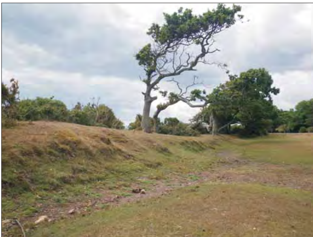
Plate C8: WA3020 . Bank earthwork forming part of the original medieval sea defences at Sowley Marsh
