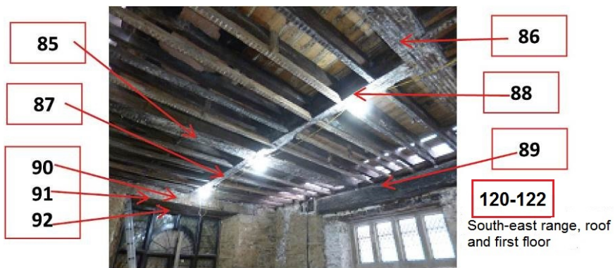
Figure 10c-f: Annotated photographs to help locate the sampled timbers (photographs Robert Howard)
