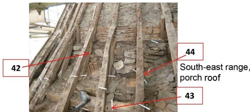
Figure 9m-p: Annotated photographs to help locate the sampled timbers (photographs Robert Howard)
