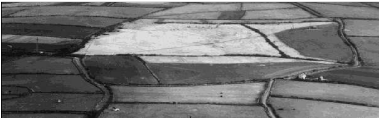
Figure 58. A complex of radar buildings at Baxworthy, MDV 102234, including two buildings in the foreground, transmitter block centre left (detailed below left), and receiver block top right (detailed below right). Between them posts are visible across Baxworthy Moor. In the centre foreground built into the hedgebank is brick structure MDV 102248, described below. NMR RAF/SOP/122 PSFO-0007 SS2922/1 3-MAR-1954. English Heritage (RAF Photography).
