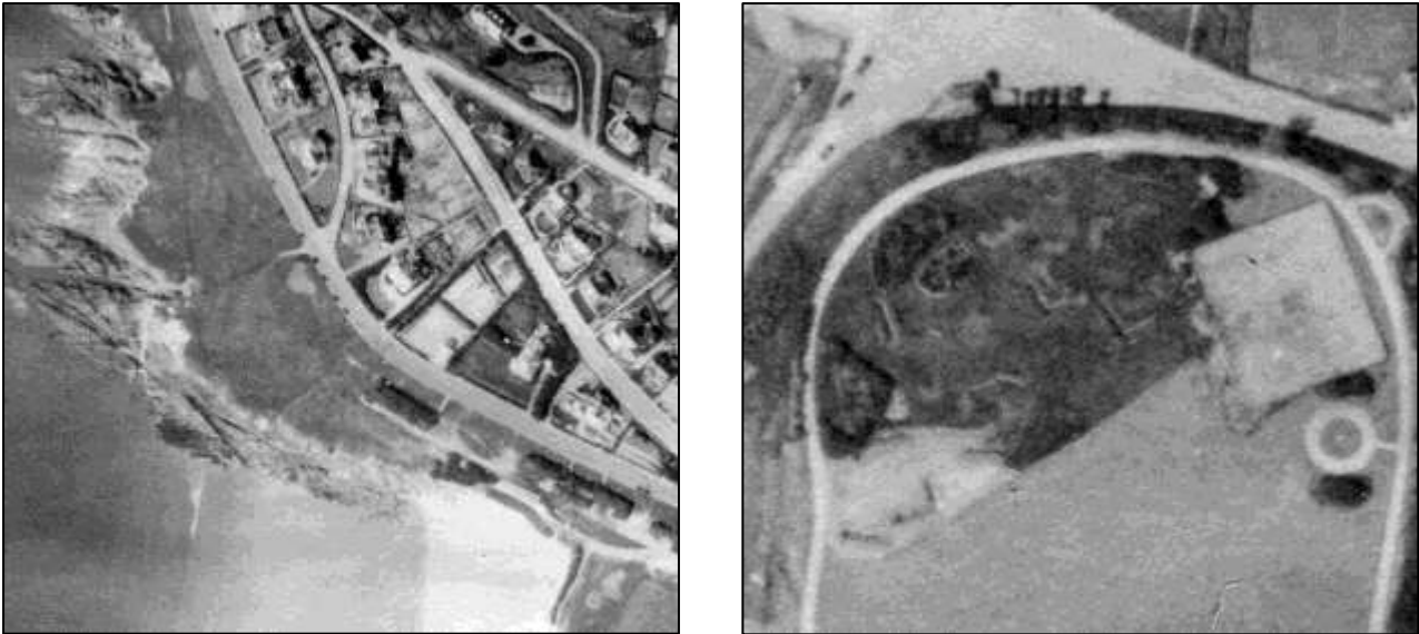
Figure 23. Slit trenches on the cliff top at Woolacombe, infilled (left, MDV 103257) and open (right, MDV103263). Note the Nissen-type huts on the cliffs above the beach. NMR RAF/106G/UK/1501 3277 13-MAY-1946. English Heritage (RAF Photography).
