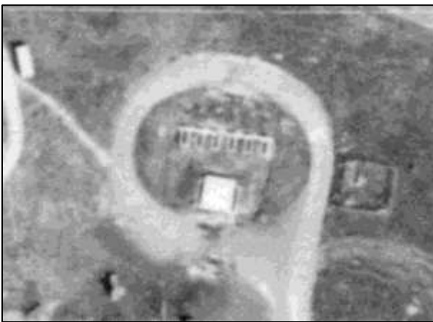
Figure 24. Possible air-raid shelters at RAF Chivenor. Top: Five oblong earthwork mounds covering hardened structures along the northern access road at the airfield, hardened entrances visible as pale lines in the earthworks. Left: A roughly square earthwork with six possible entrances on its northern side might have provided larger accommodation. RAF/106G/UK/1655 4328 11-JUL-1946. English Heritage RAF Photography.
