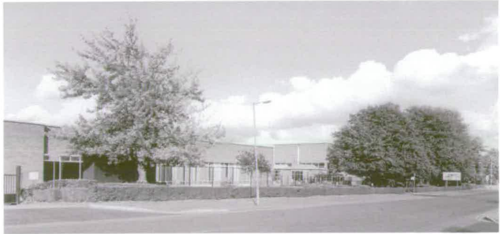
Figure 25 BAE Systems, view of rear in Paycocke Road from south west, note ornamental planting (AA021647). (C) English Heritage
