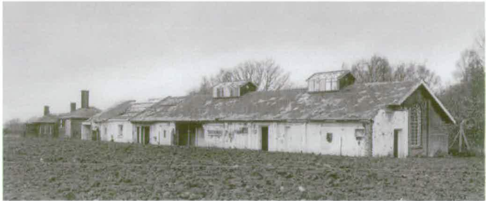
Figure 19 Exterior of the radio workshop incorporating the 1903/4 Shell and Cartridge Stores (AA00/1085). (C) English Heritage
