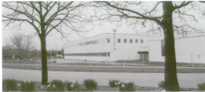
Figure 21 Taveloc House, Freebournes Road from east (AA0021636). (C) English Heritage
