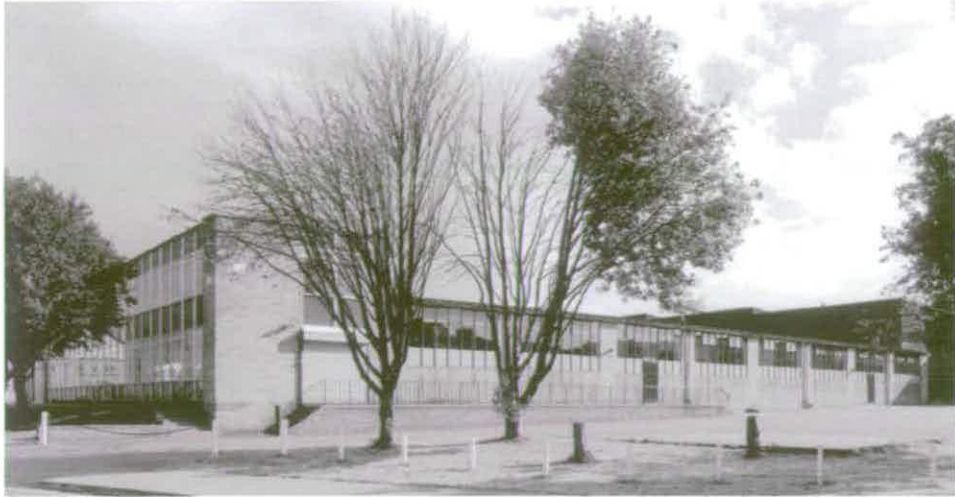
Figure 23 Former Marconi Communications Systems, Radford Crescent, from south east (AA021631). (C) English Heritage
