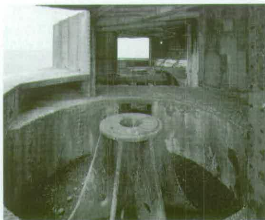
Fig 5. East six-inch gun emplacement showing pedestal (NMR AA98/02136).
