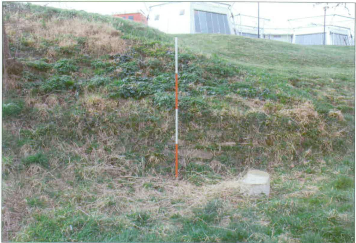
Plate 4 Conisbrough Castle: revetment wall at base of terrace facing west
