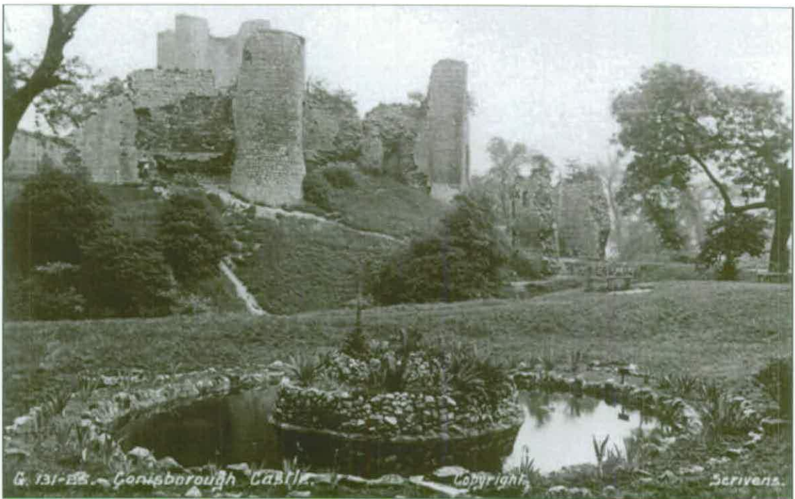
Plate 38 Conisbrough Castle: castle pond (© English Heritage)
