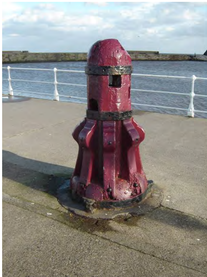
Plate 2 Detail of one of the capstans on the West Pier at Whitby
