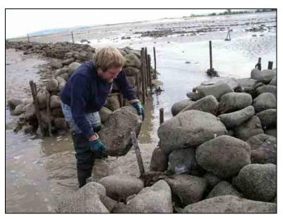
Figure 5-39 A stone weir at Minehead under much needed repair in 2007 Reproduced with the kind permission of © Nick Russell
