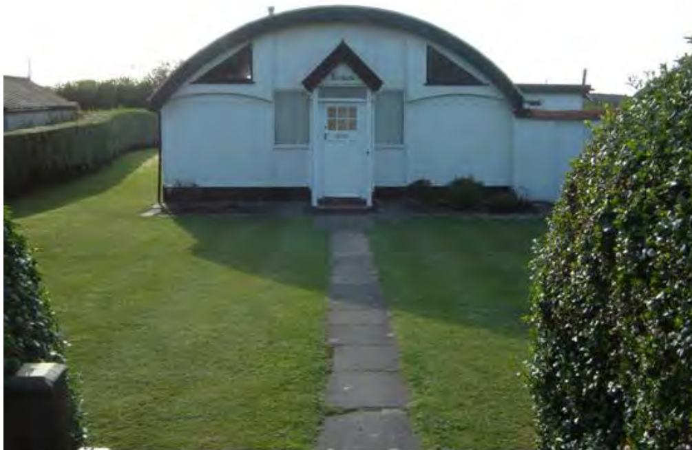
Plate 18 Eastern gable of Lindum (MS77), showing panelled carriage ends either side of the doorway, Mablethorpe
