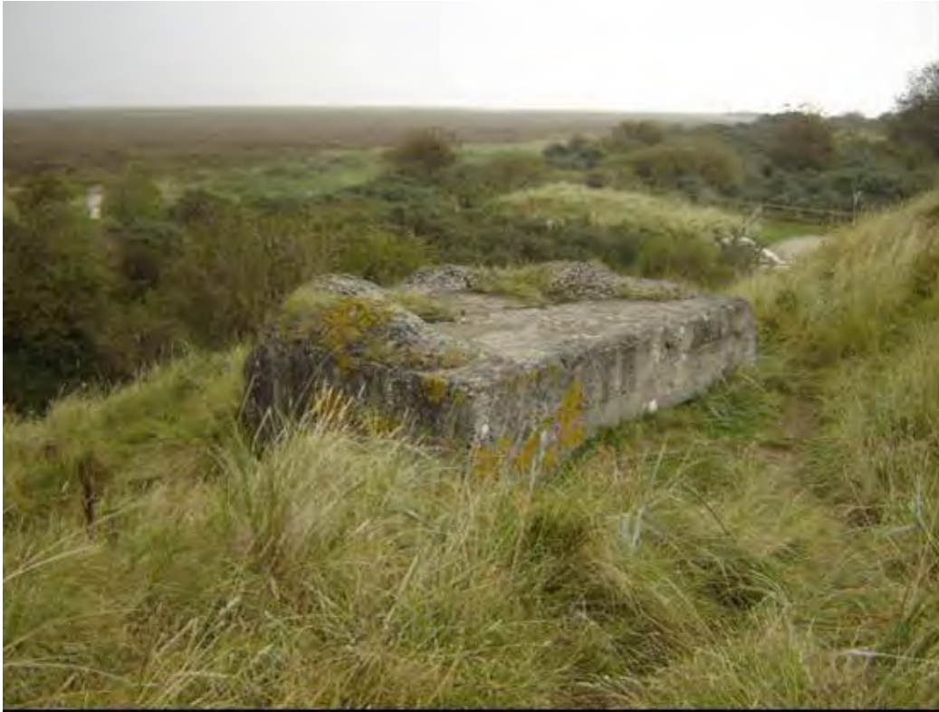
Plate 9 Pillbox (SA11), with concrete on roof to break up outline, Saltfleetby
