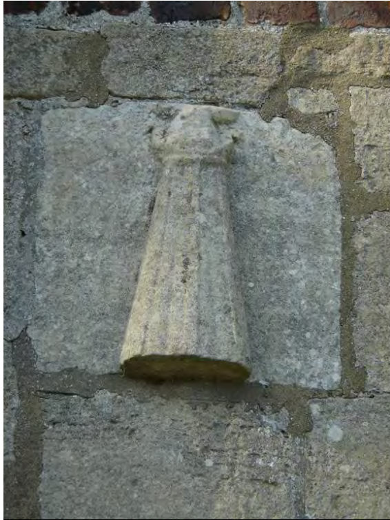
Plate 23 St Clement's Church, Mablethorpe (MS86). Detail of reused medieval stone with carved pinnacle west of the porch door
