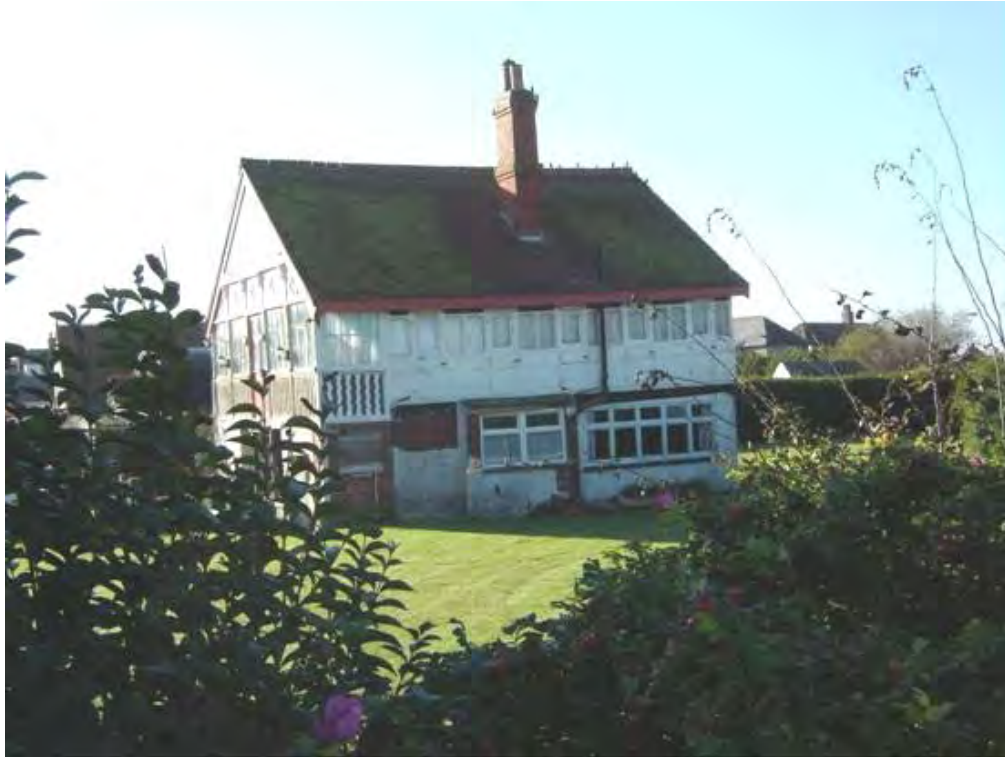
Plate 17 Wavelands (MS75), partially constructed from railway carriages, Mablethorpe
