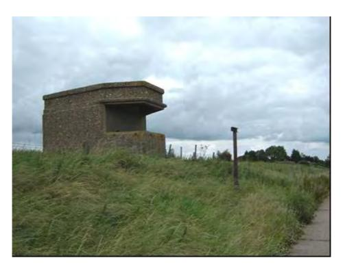
Plate 11 WW2 coast artillery searchlight emplacement (FR20) on seabank forming part of Freiston Shore Battery near TF 3961 4216; this building has been converted to a store by blocking the embrasure and placing a door across the rear access
