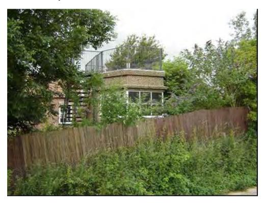
Plate 14 WW2 coast artillery searchlight (CASL) emplacement (FR10) forming part of Freiston Shore Battery, converted to summerhouse on seabank, near TF 3969 4234
