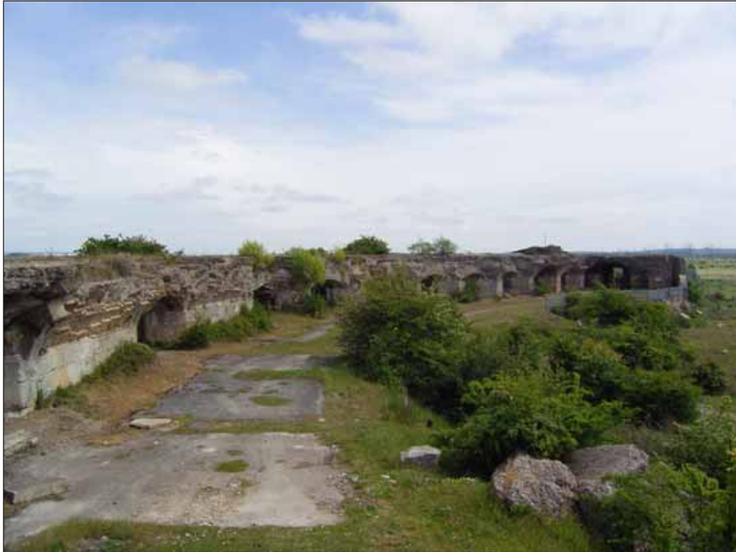
Plate 6: Higham Stretch, showing part of Shornemead Fort (TQ 67 SE 63).
