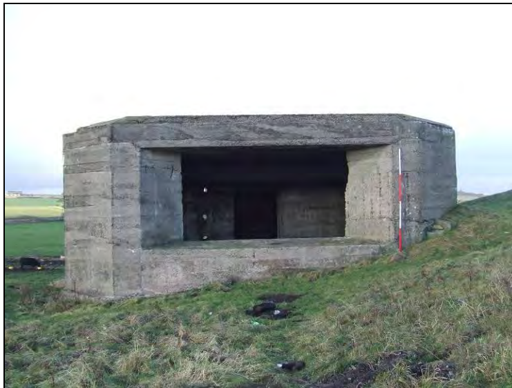
Fig 7.16 Gun emplacement at Scremerston, built on top of a trackway associated with a limestone quarry and associated kilns (Scale = 2m).
