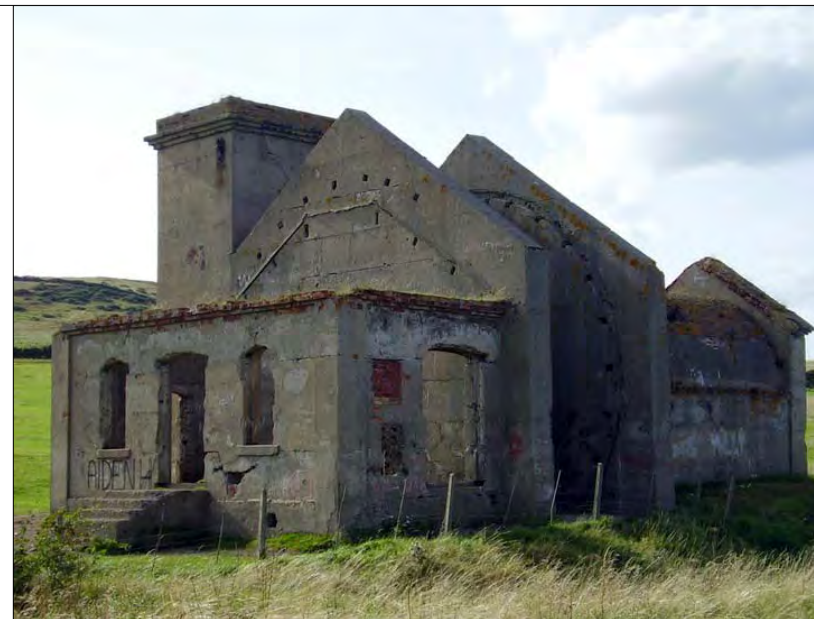
NERCZA2_0032: GPS 19. Huntcliffe Ironstone Mine, Guibal Fan House
