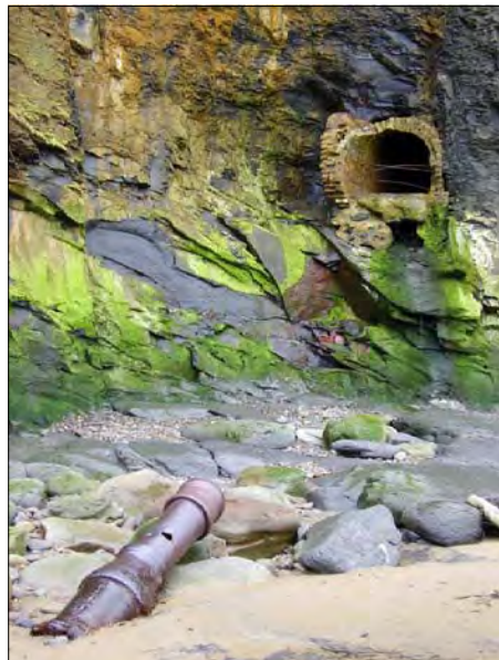
NERCZA2_0065: GPS 24-25. Outfall Sewer
