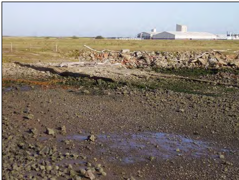
Fig. 7.19 The preserved slipway to the First World War seaplane base at Seaton Carew.
