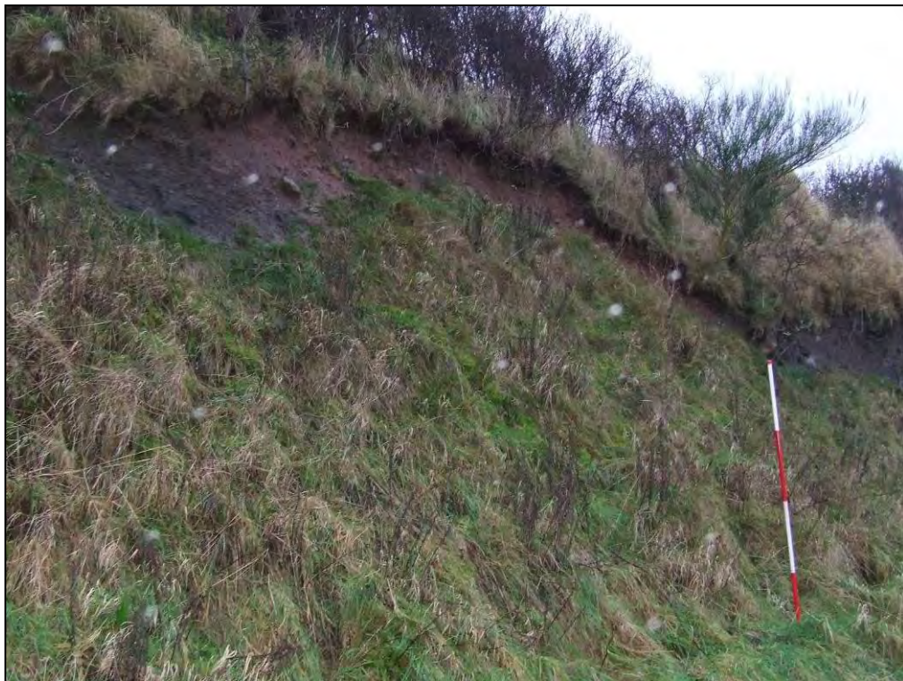
Fig. 7.6 The location of a slump below the Fenham enclosure. The ranging pole shows the location of the original centre of the enclosure bank which can be seen as a slight upstanding earthwork on the ground surface above (Scale = 2m).
