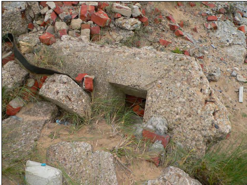
Fig 5.4.11 remains of loop holes in concrete wall fragments from demolished pillbox
