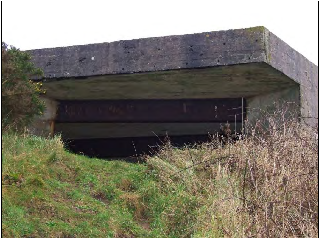
Fig 5.16.13 Budle battery (500), clearly demonstrating scale of construction.
