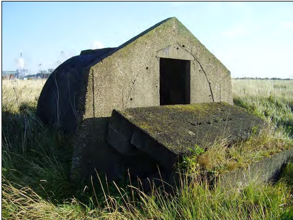
Fig 5.4.3 Stanton type air raid shelter at Greatham Creek, part of former bombing decoy.
