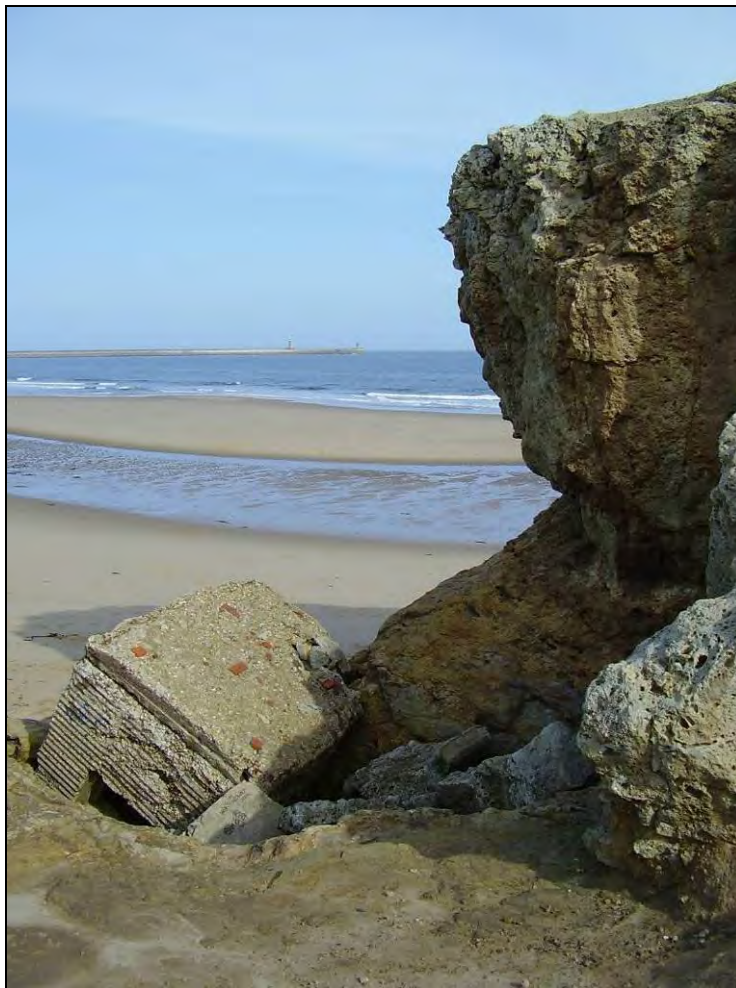
Fig 5.6.11 The gun position 139 on the beach having fallen from the top of the cliff on to the beach.
