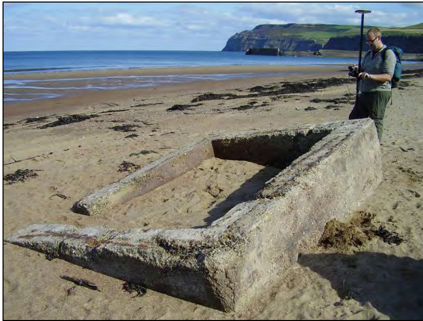
Figure 5.3.15 Slumped pillbox on the beach looking south towards Skinninggrove harbour as seen in September 2009 .
