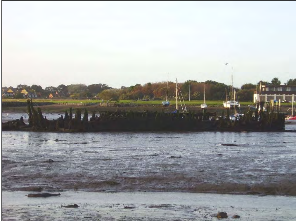
Fig 5.11.7 Vessel 355 lying against the former harbour wall 453
