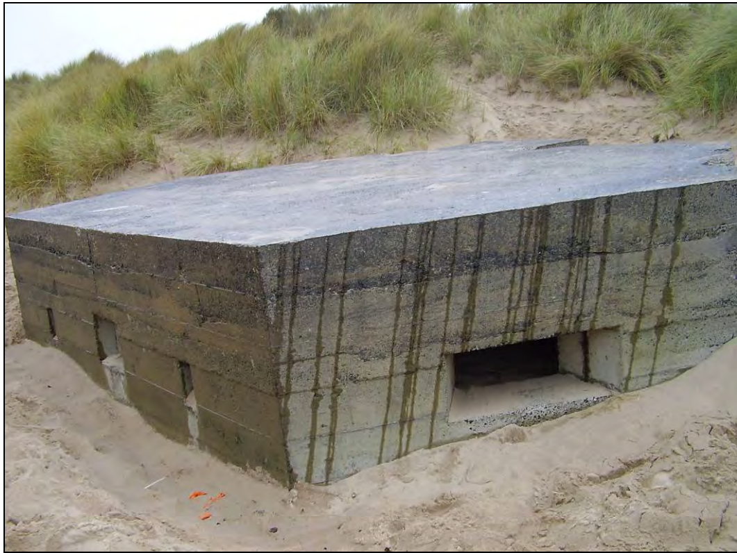
Fig 5.8.15 Pillbox exposed in dune in central Druridge Bay.
