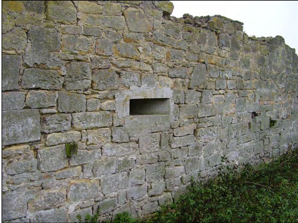
Fig 5.10.14 A Second World War loophole placed in the wall of the post-medieval guano shed.
