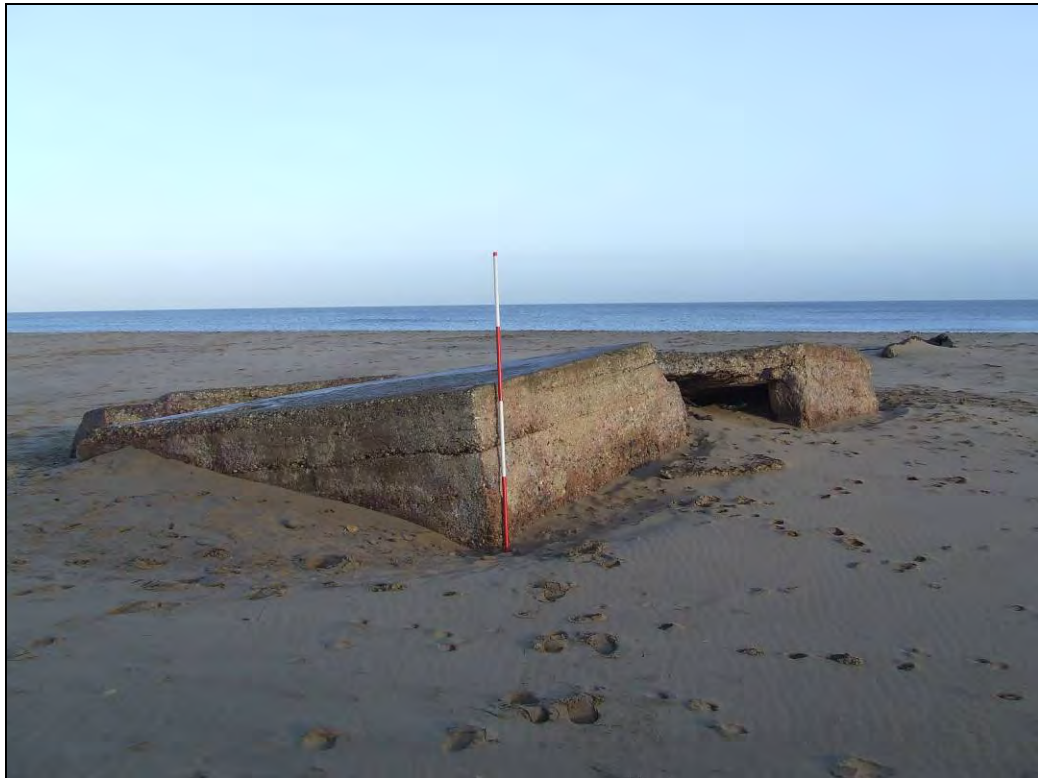
Fig 5.5.12 One of the exposed pillboxes (106) on the beach at Crimdon Dene.
