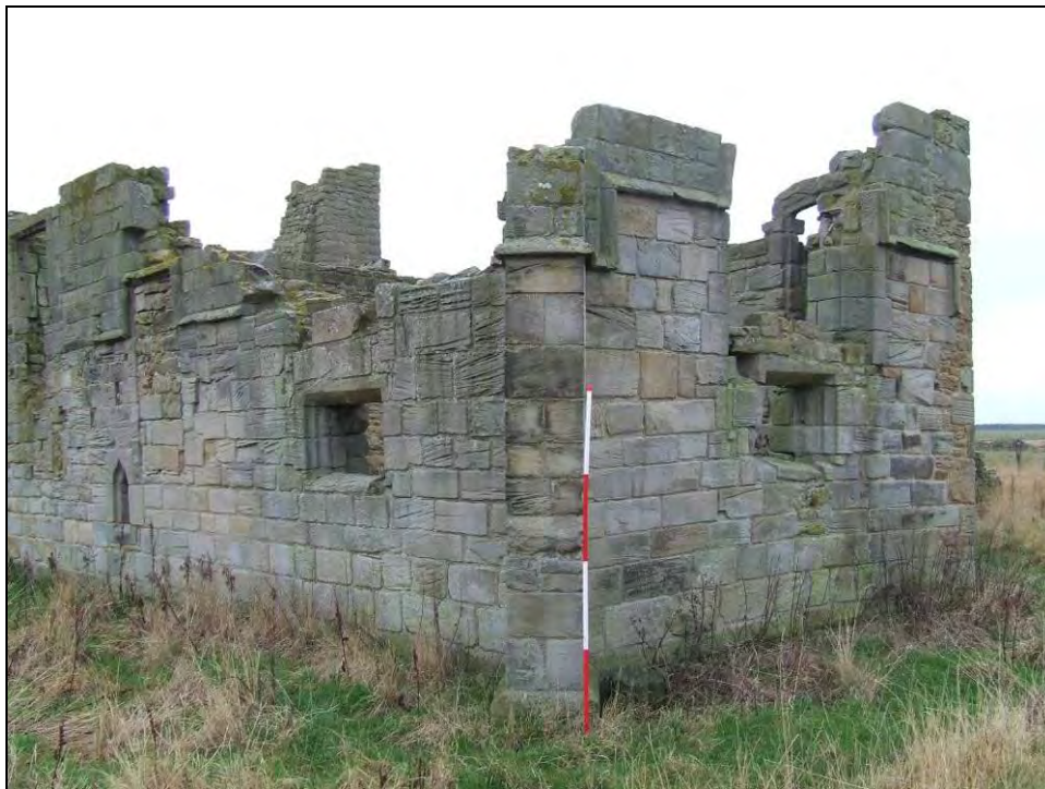
Fig 5.8.5 Part of the original Preceptory at Low Chibburn, with Second World War alterations to windows.
