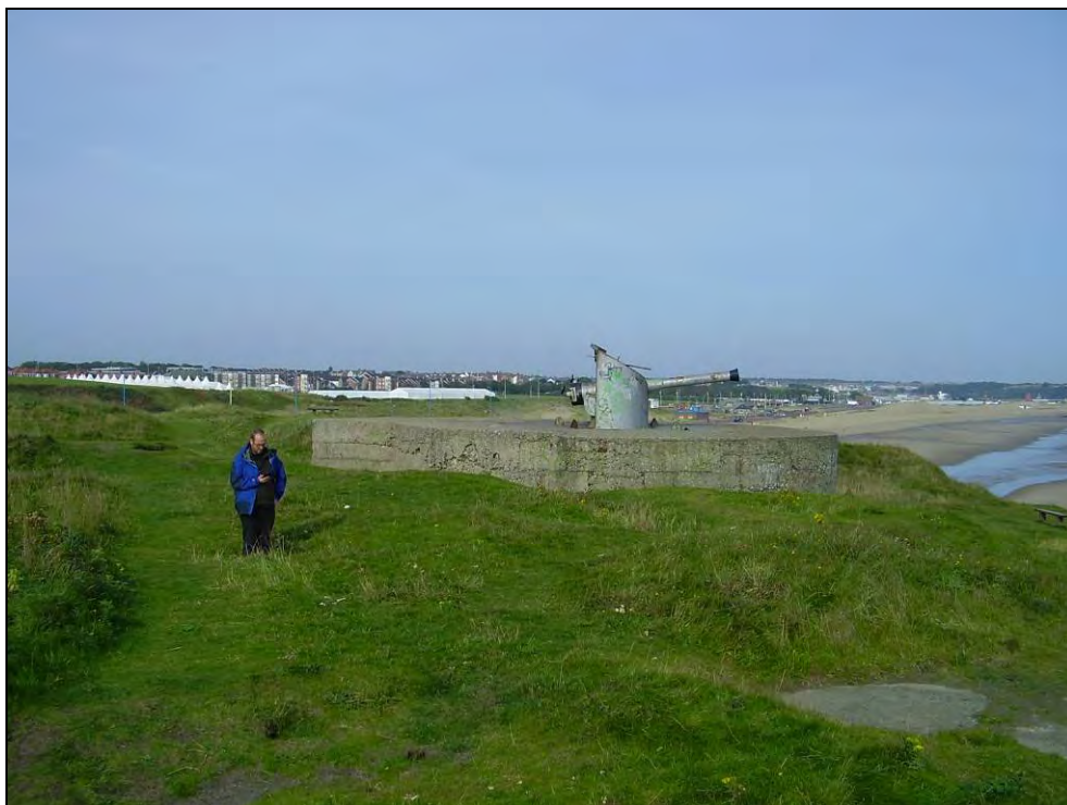
Fig 5.6.7 The position and depth of one of the weapons pits with one of the WW1 gun positions visible in the foreground.
