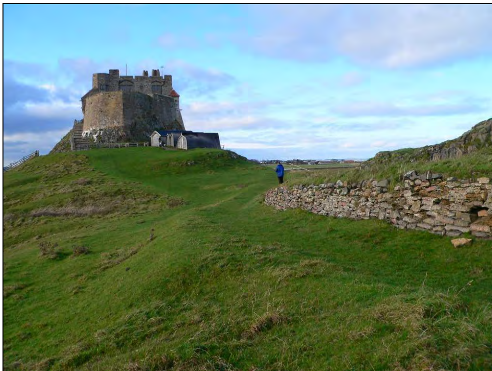
Fig 5.14.15 The stone built fire step, or loading bay and raised bank for the lime kilns.
