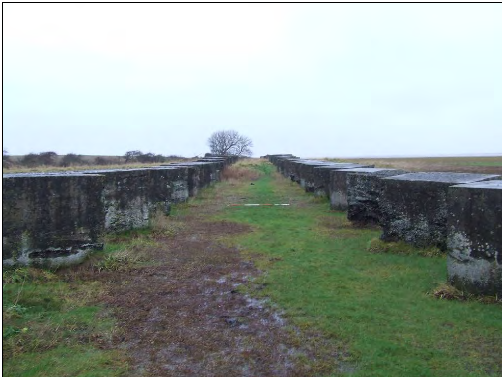
Fig 5.13.12 Row of anti-tank blocks north of Fenham
