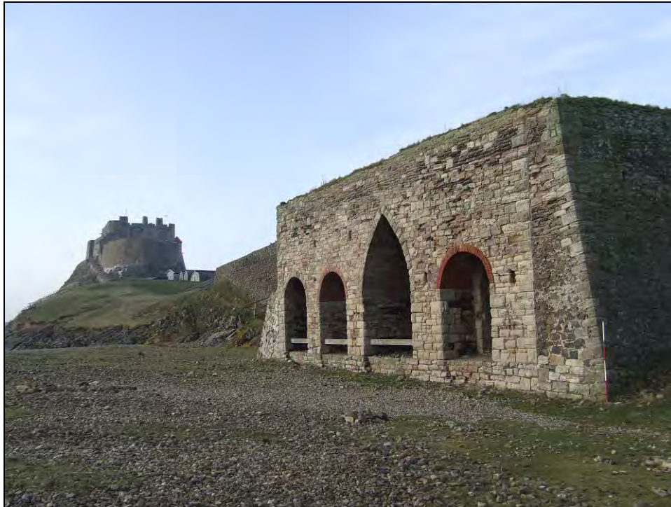
Fig 5.14.11 The impressive Lime Kilns (403) below Lindisfarne Castle
