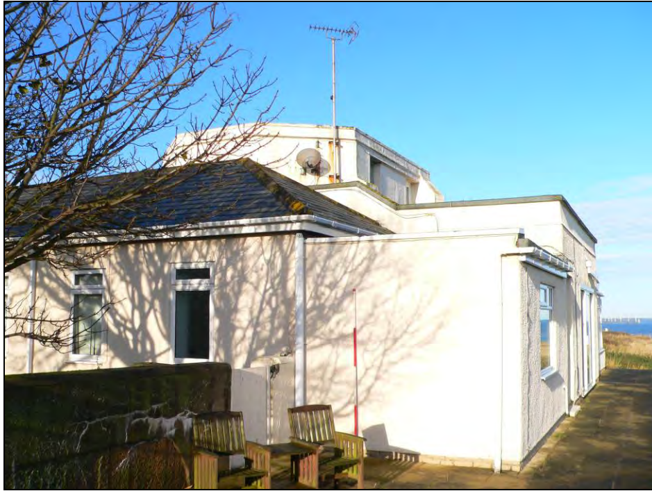
Fig 5.7.8 Exterior of Fort House looking north.
