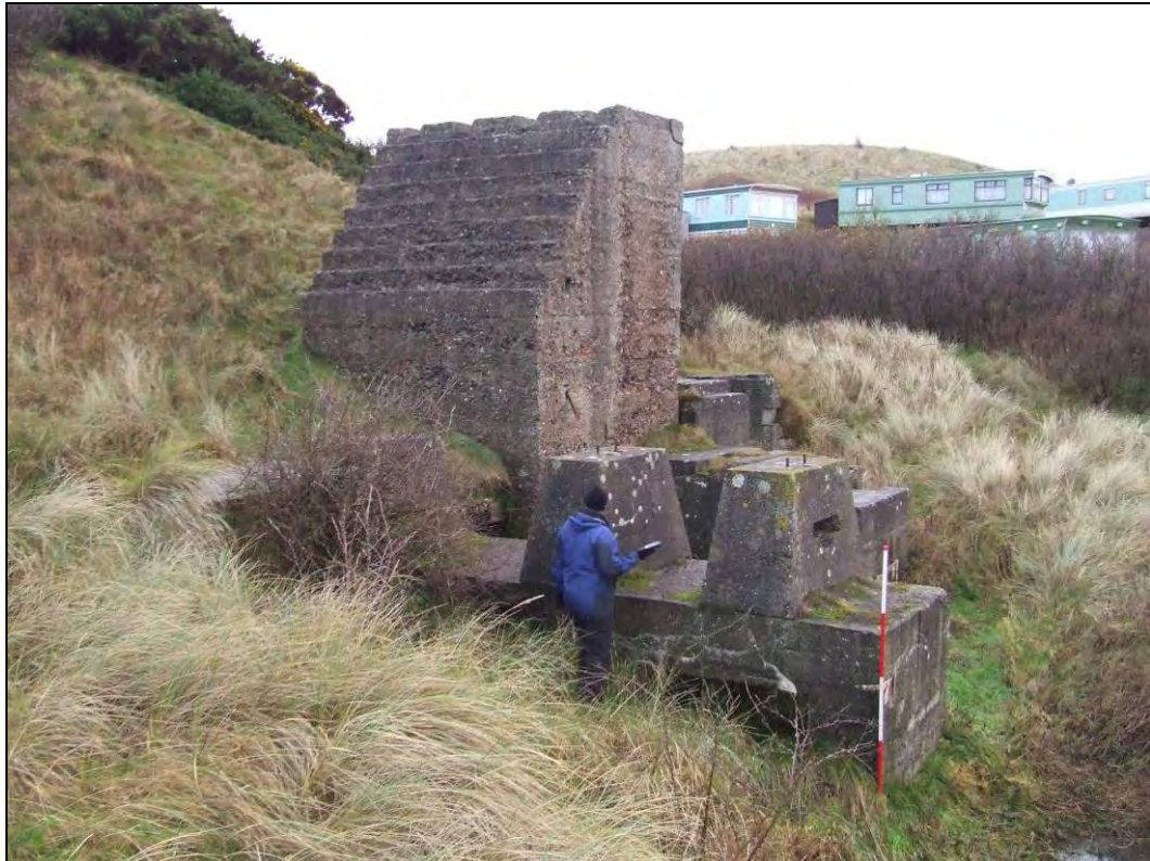
Fig5.16.25 Concrete base for winding gear for the quarry 2km to the south.
