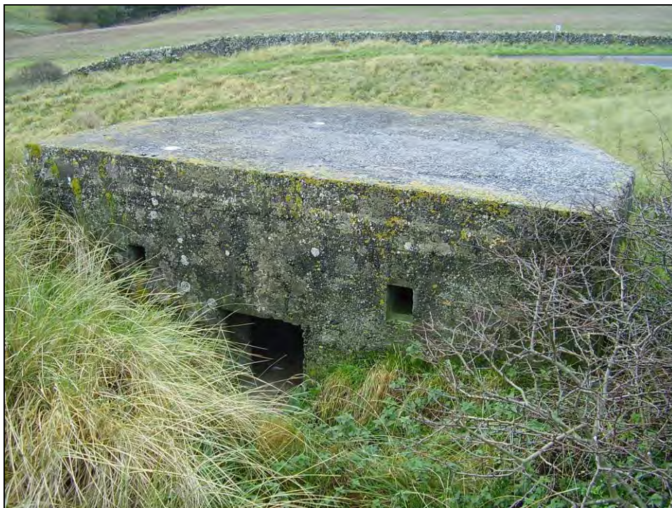
Fig 5.15.8 The rear entrance of the same pillbox.
