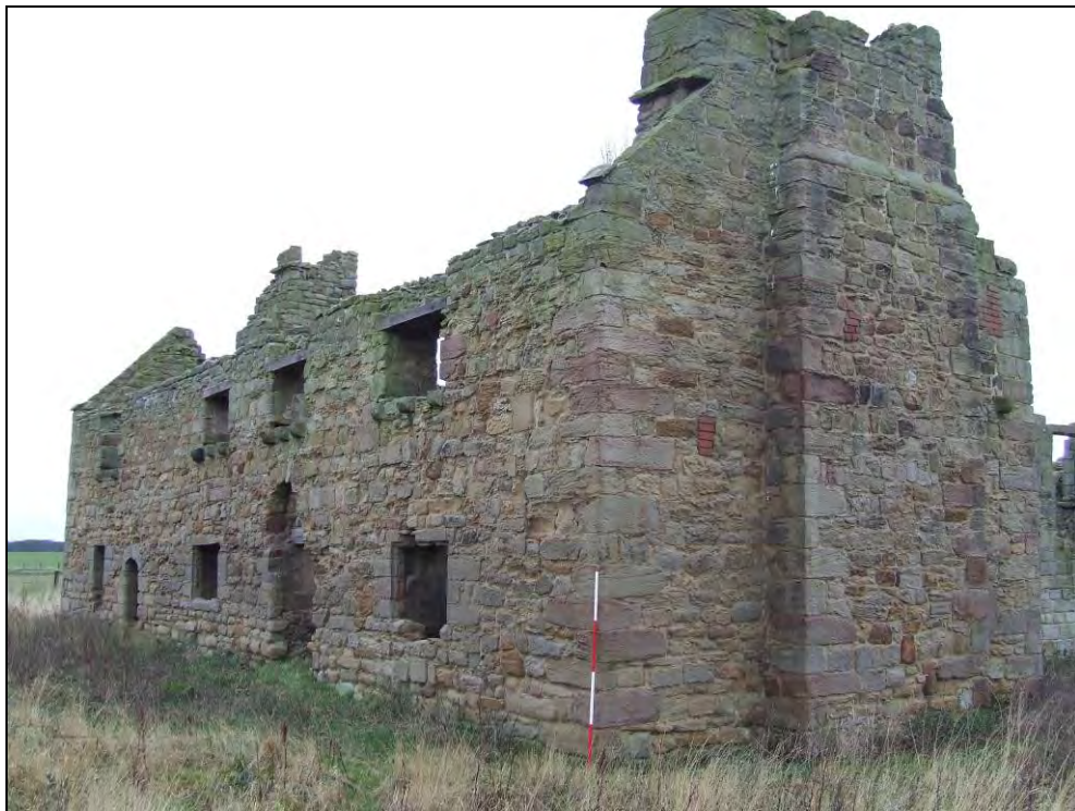
Fig 5.8.7 The later Dower house at Low Chibburn
