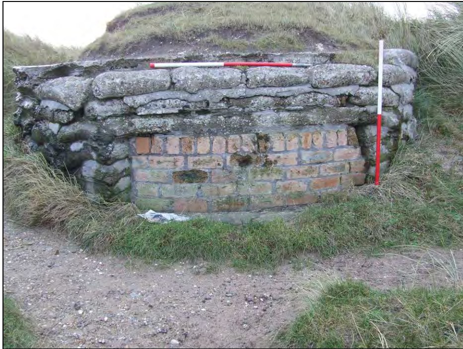
Fig 5.7.21 Circular pillbox (506) showing brick-blocked aperture.
