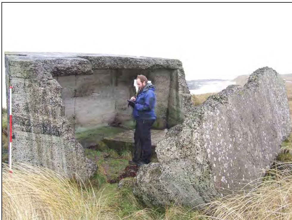
Fig 5.16. 21. Destroyed pillbox (672) in the dunes between Seahouses and Bamburgh.
