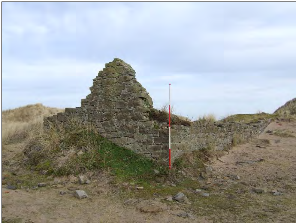
Fig 5.14.17 Partially upstanding gable end of Longhouse (409)
