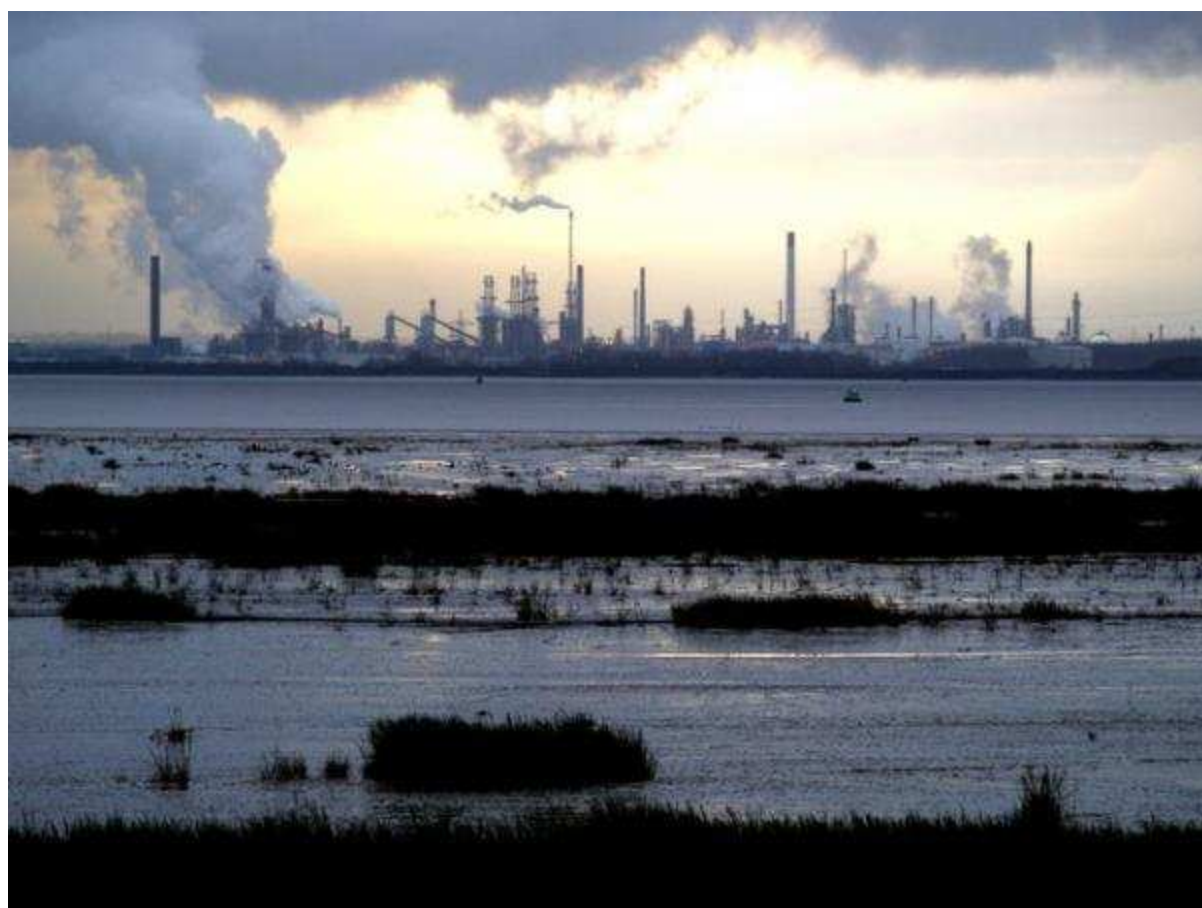
Figure 34. Oil refinery at Killingholme close to Paull Holme.
