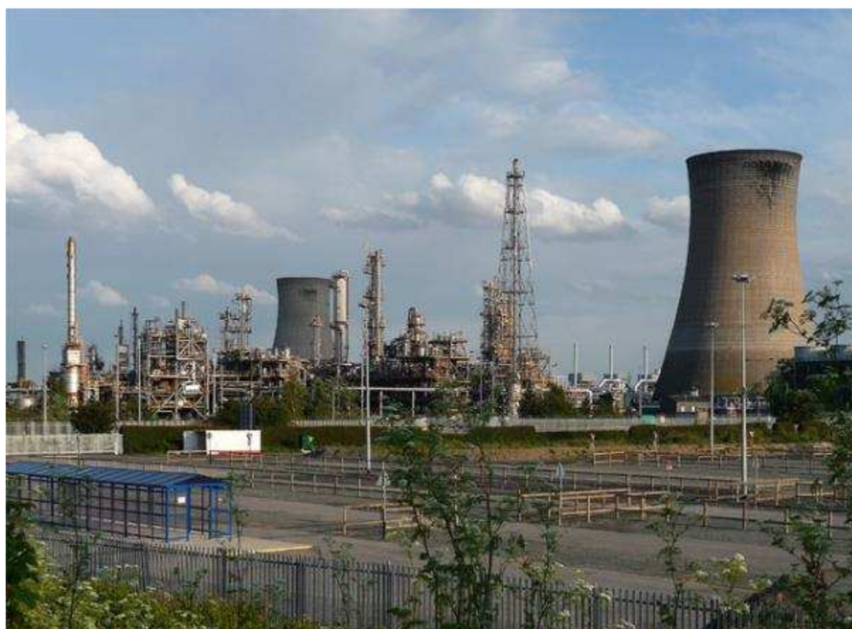
Figure 35. Salt End salt production works, east of Hull.
