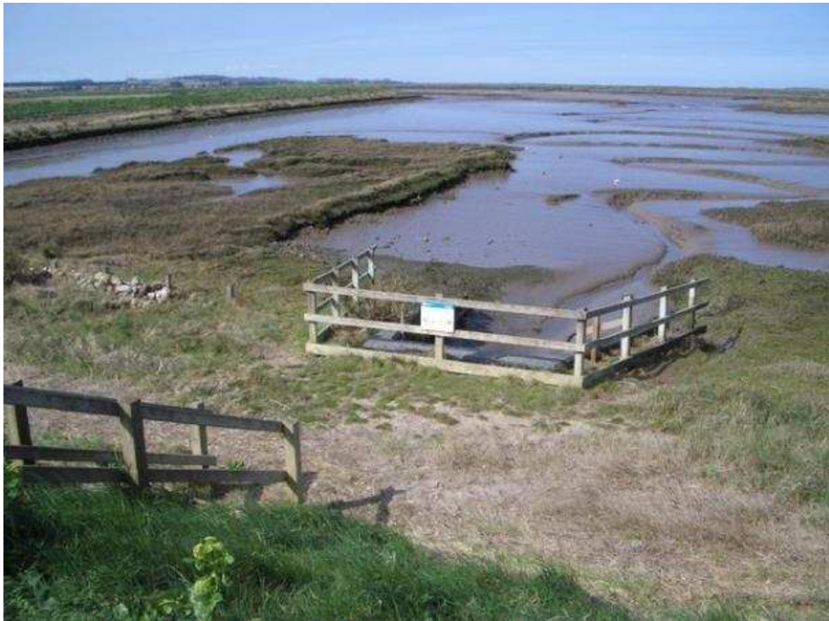
Figure 4. Sluice outlet and mud flats close to Brancaster.
