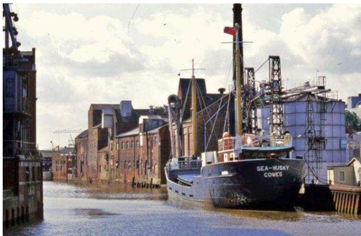
Figure 45. Kingston-upon-Hull docks, south of Scott Street Bridge.
