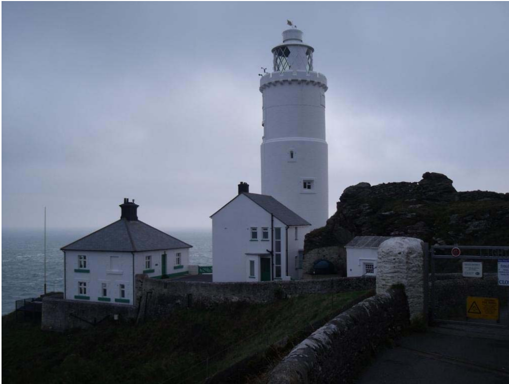
Fig 8 Start Point lighthouse. (Photograph; Cornwall Council.)
