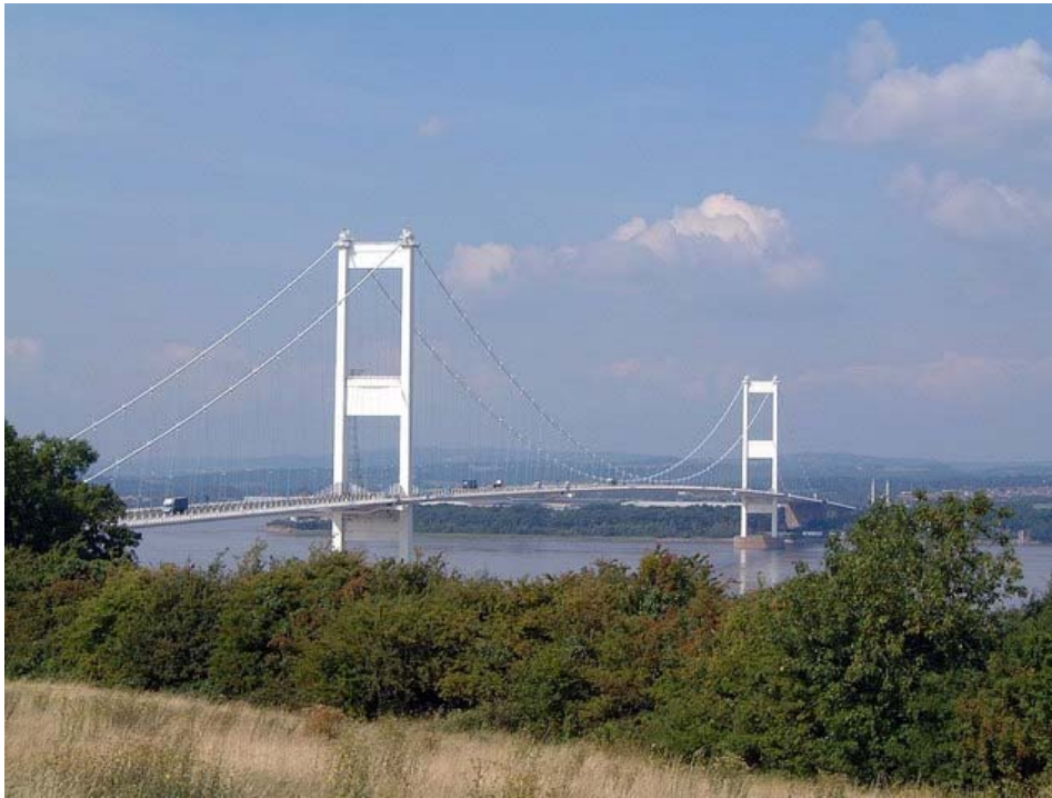
Fig 27 The old Severn Bridge viewed from Aust (©Copyright Barrie Jenkins and licensed for reuse under this Creative Commons Licence )
