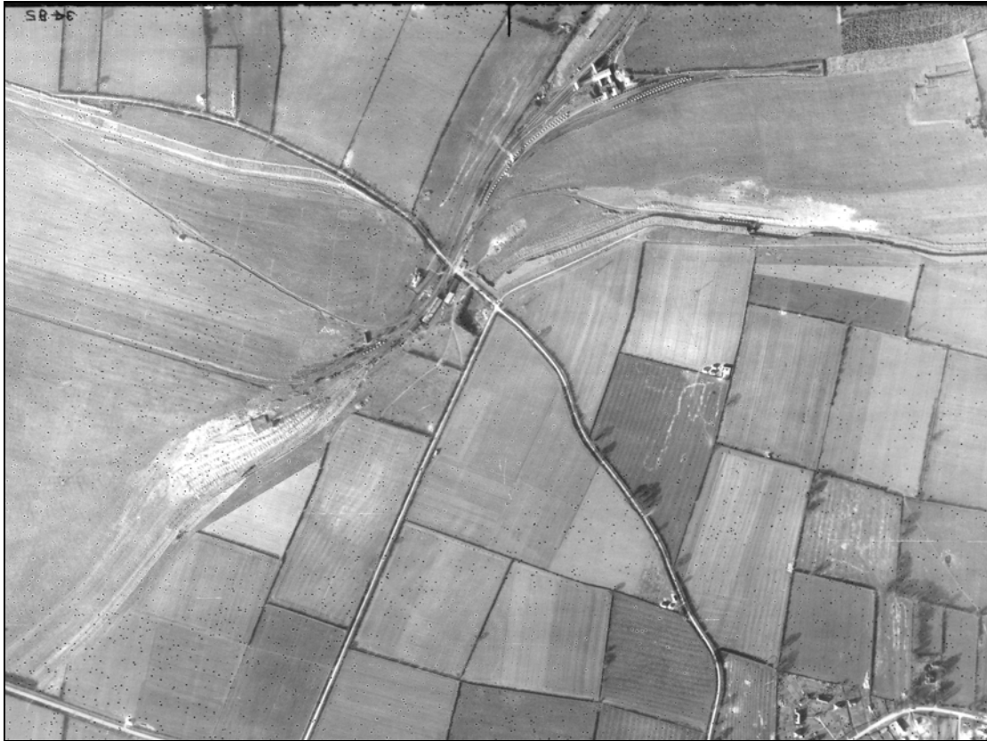
Figure 3.1: A part of the extensive ironstone quarrying at Wroxton, Oxfordshire. The quarrying extends in a fan shape to both sides of the crossroads in the centre of the image. The pale stone and linear spoil heaps show the active edge of the quarrying. The smooth ground lacking in field boundaries or ridge and furrow indicates reinstated topsoil. An extract from NMR RAF/106G/UK/1345 7200 01-APR-1946. English Heritage (EHA) RAF Photography
