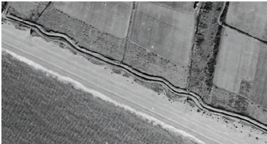
Figure 81. Anti-invasion defences at The Old Coastguards, Burton Road. A series of pits lie to the landward side of the anti-tank ditch and are possibly an earlier phase of the anti-tank defences (MDO25823). Photograph: RAF CPE/UK/2431 Frame 3284, 22nd January 1948. English Heritage (NMR) RAF Photography.
