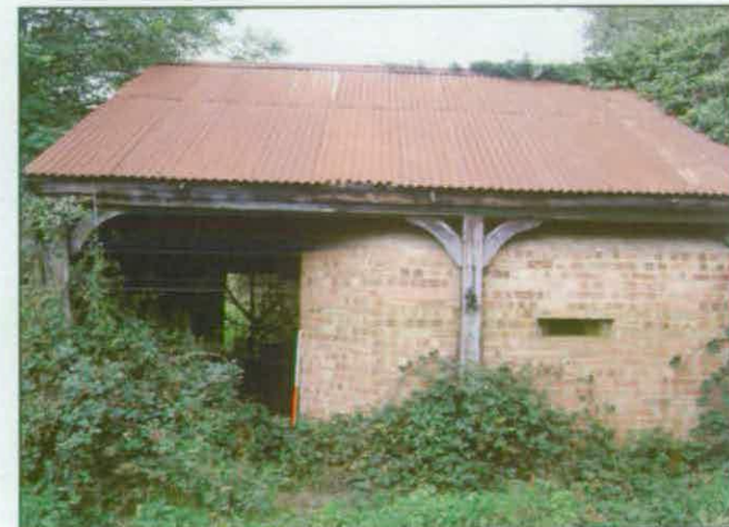
Plate 30: Pill box (01) constructed within cart shed adjacent to Tilty Mill, from south-east
