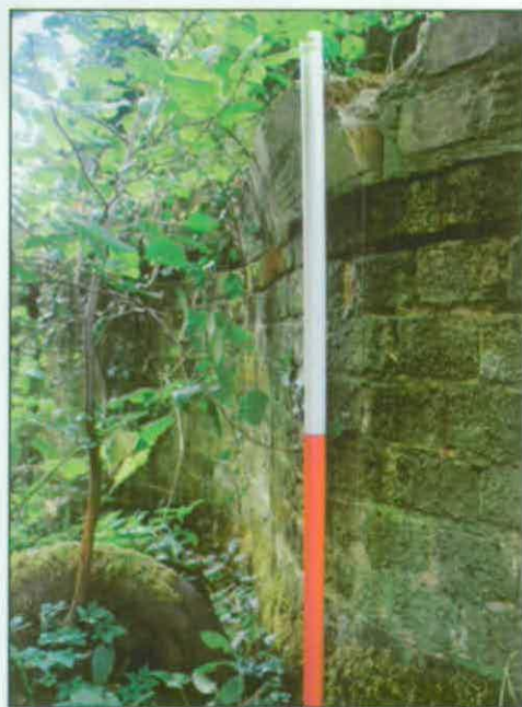
Plate 15: Inner curving profile of sluice gate (02d), from south-east
