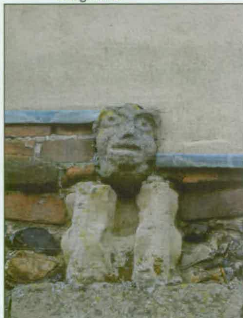
Plate 29b: Detail of stone in wall at Park Farm, Thaxted
