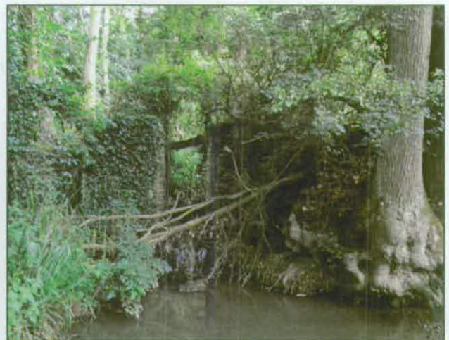
Plate 14: Sluice gate and bypass channel (02d), from north-west
