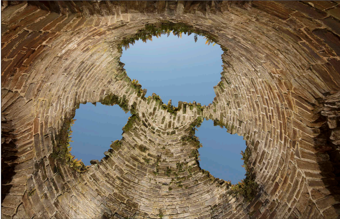
Fig. 12 The stone roof of the bath room on the south, built to resemble a ruin (© Historic England, Patricia Payne DP232121)
