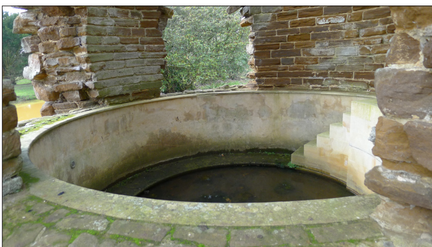
Fig. 16 The bath in the south room of the Bath House looking south-west, and showing the two stages of the tank (© Historic England, Jonathan Kewley)
