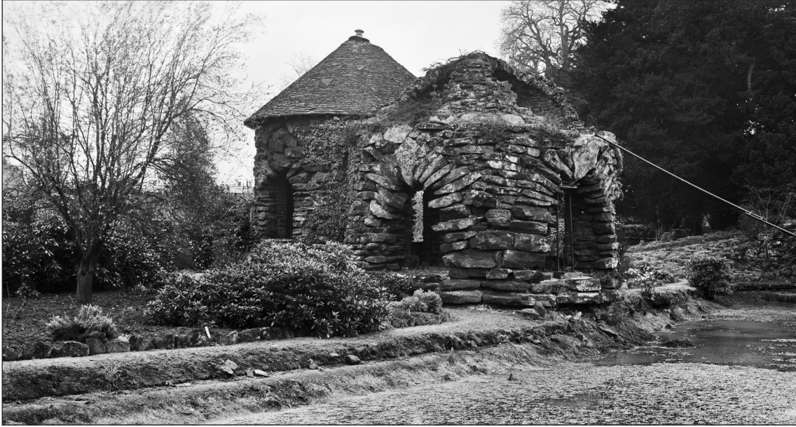
Fig. 53 The Bath House from the south-west in April 1954, showing how it had been undermined by the Bath House Water (p_a03147_001 Historic England Archive)
