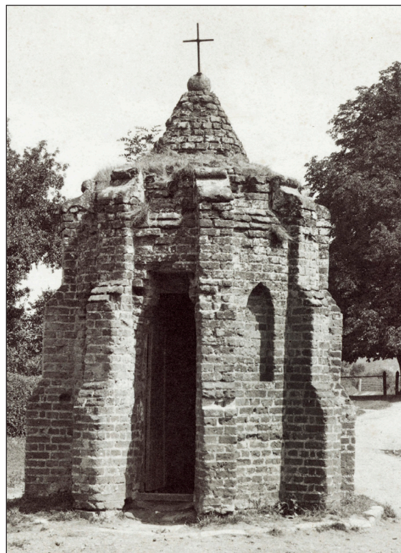
Fig. 40 (right) The Pump House, Rushbrooke, Suffolk, attributed to Thomas Wright (photographed between 1880 and 1917; OP27927 Historic England Archive)
