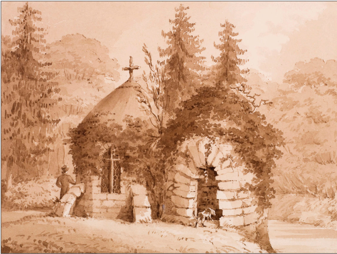
Fig. 45 The Bath House at Wrest, c. 1831 (detail from a watercolour attributed to Earl de Grey; DP110042 ©Historic England Archive)
