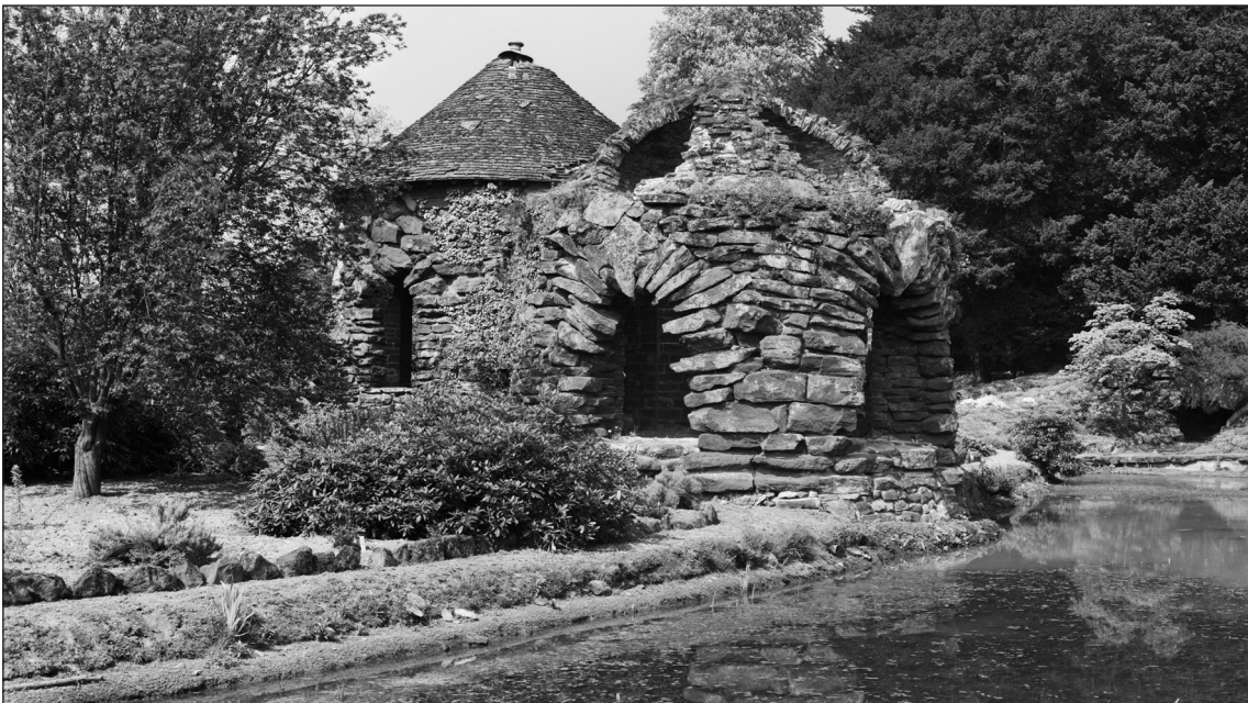
Fig. 54 The same view a month later, after underpinning (p_a03177_003 Historic England Archive)
