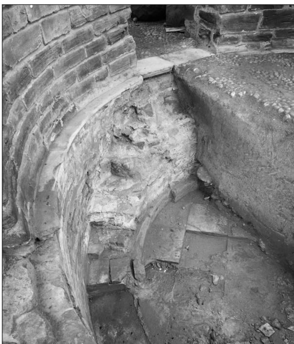
Fig. 52 The southern room of the Bath House in 1963, showing the pebble-topped earth filling (presumably dating from 1834) partly dug out to reveal the bath (p_a06331_003 Historic England Archive)
