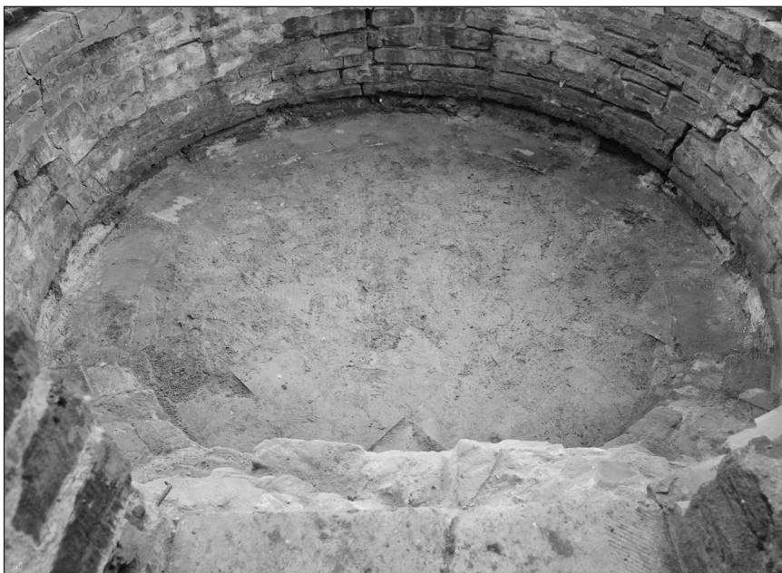
Fig. 59 The bath at Wrest in January 1968 after excavation but before ‘restoration’ (p_ao7506_001 Historic England Archive)
