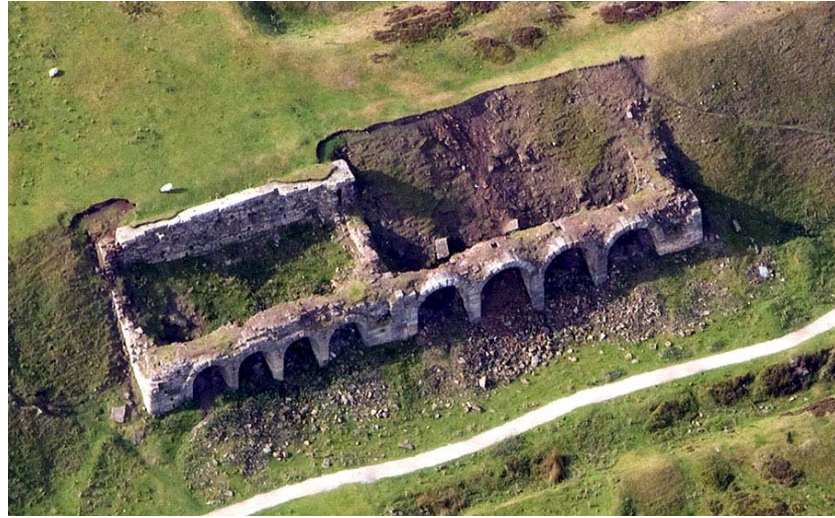
Figure 17. Calcining kilns at Top Bank in Rosedale (1300063) resulted in calcine dust which was reused after the closure of the mine
