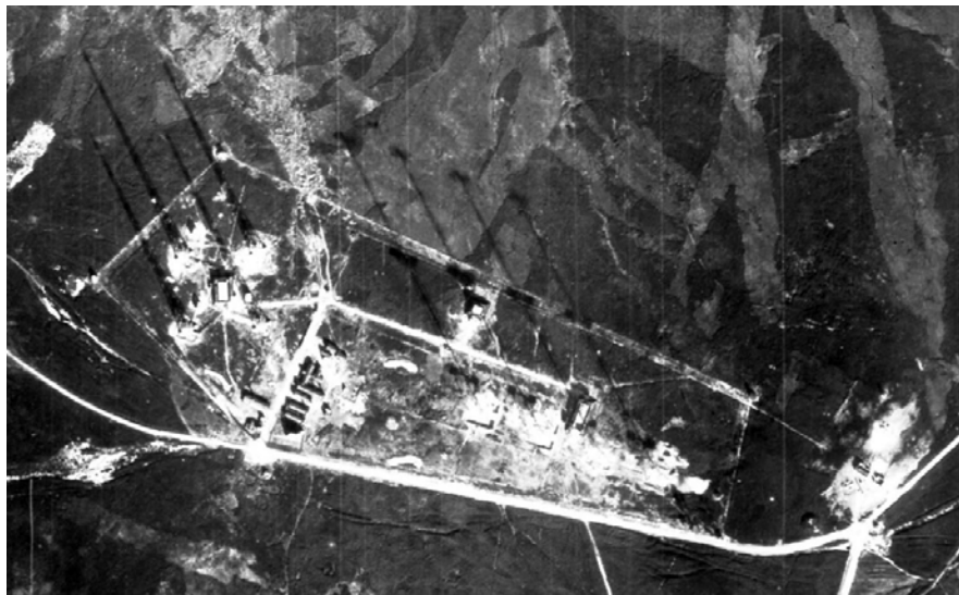
Figure 20. Danby Beacon radar station (1336422)
