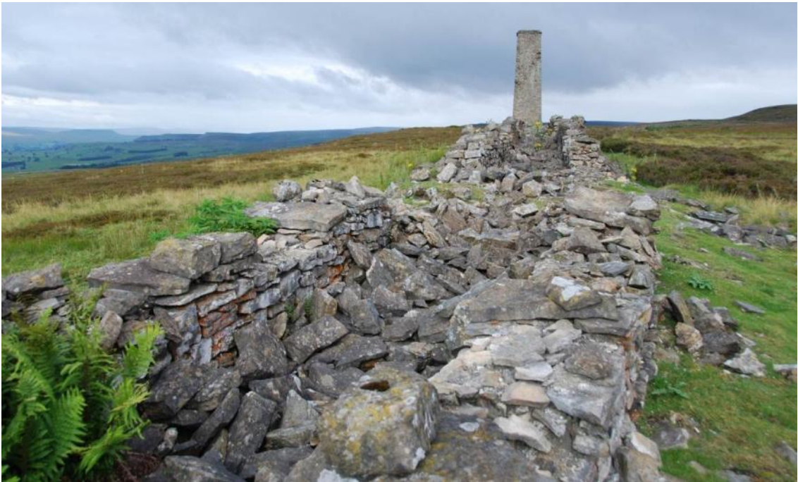
Figure 5.18: Cobscar Rake: Relict chimney and flue features associated with former lead mining activity on the ASMRP 14 limestone moors above Redmire Scar, in Wensleydale
