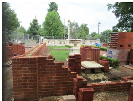
New structure being built in cemetery
