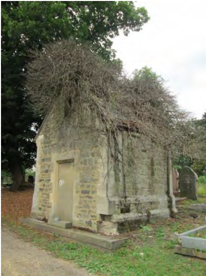
The only mausoleum (surviving), in poor condition
