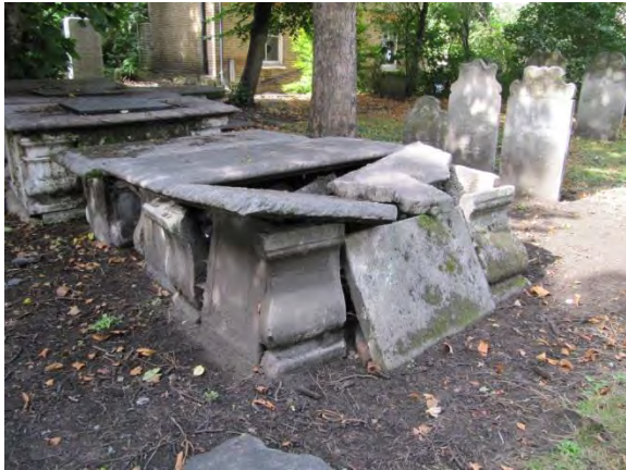
Damaged chest tombs; view left is the worst case, most have one or two collapsed panels
