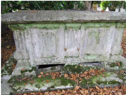
Loss of detail on reliefs from weathering
