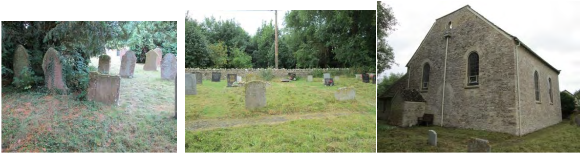
Left: C19th area of burials south of chapel. Centre: C20th/C21st area of burials west of chapel. Right: Rear (west) elevation and south elevation of chapel.
