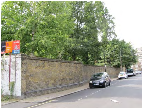
Exterior wall on Alderney Road (in good condition)
