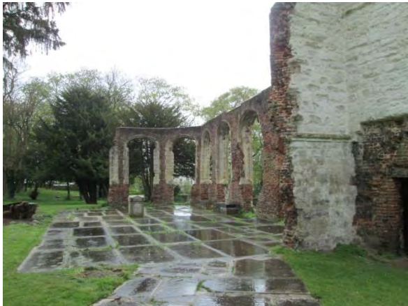
Fine C18th memorials with Christian symbolism cleared and re-used as paving, deteriorating in places
