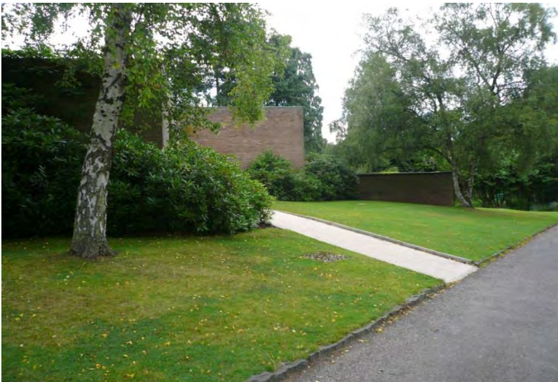
View towards the entrance building range
