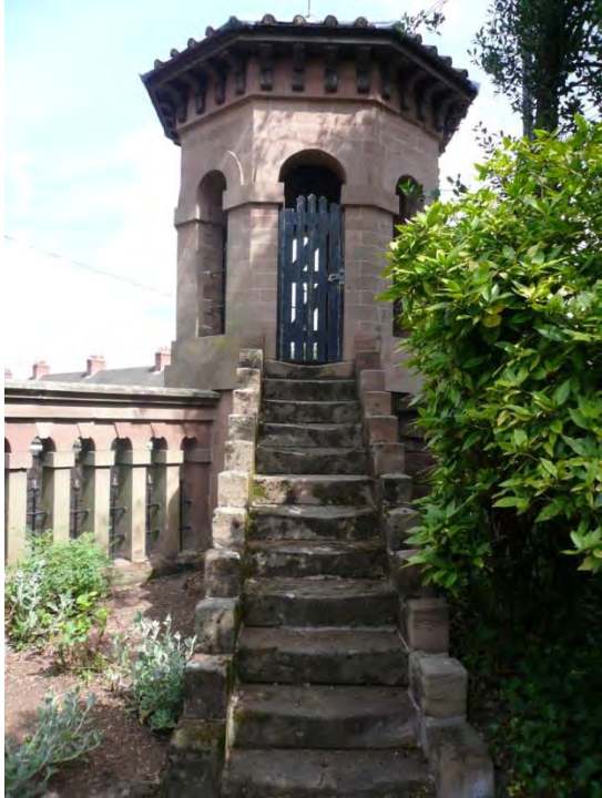
Gazebo near main entrance
