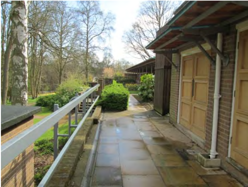
Rear of chapels and cremator on terrace overlooking woodland walks
