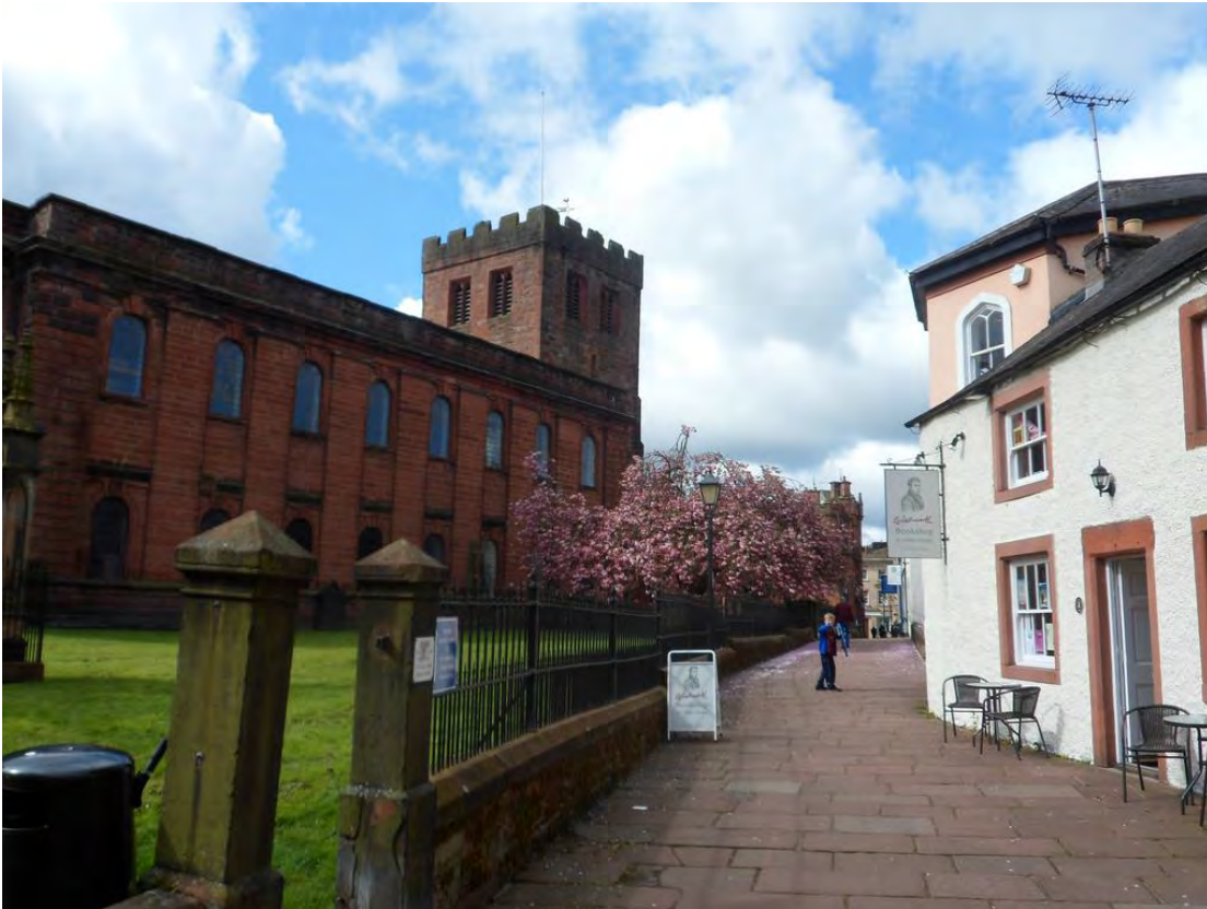
C19th century railings north side of the churchyard
