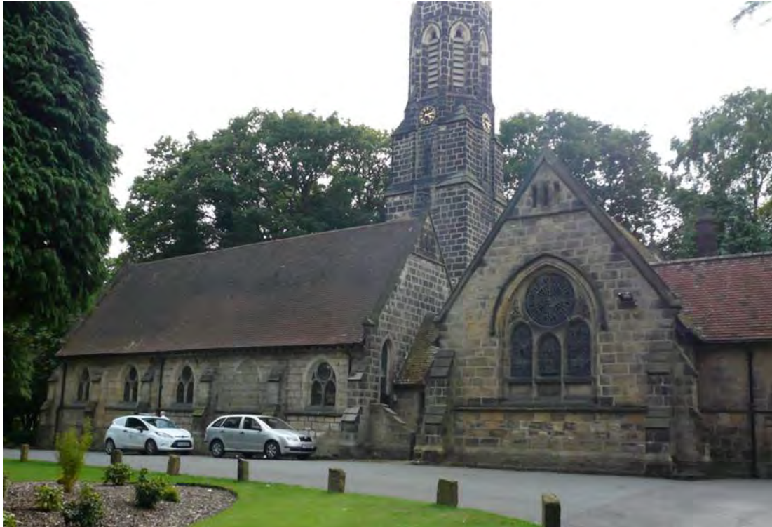
The chapel group and original crematorium chimney/tower
