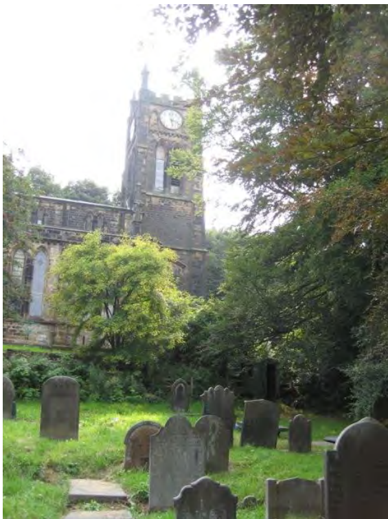
Area maintained by Calderdale Council, mown
