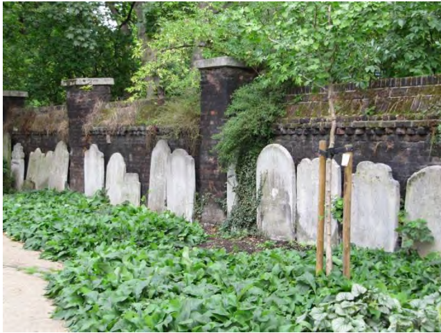
Perimeter wall and headstones, both in good condition
