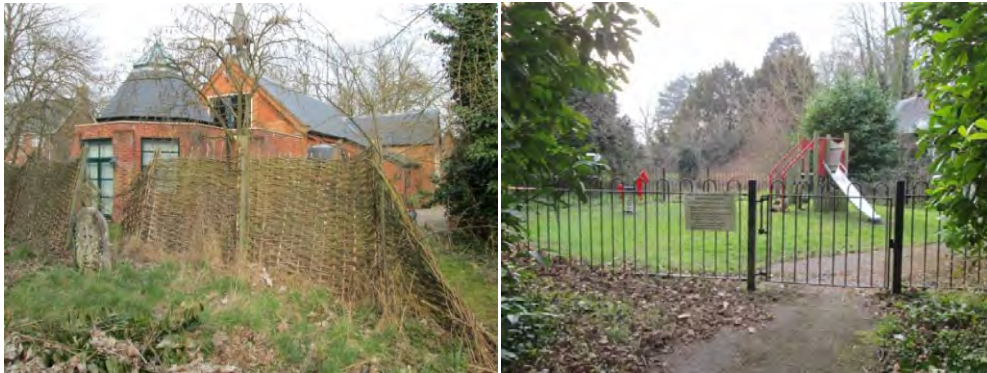
Left: rear of earlier chapel, boundary with burial ground. Right: Children's play area in burial ground entered via original burial ground gateway (right).
