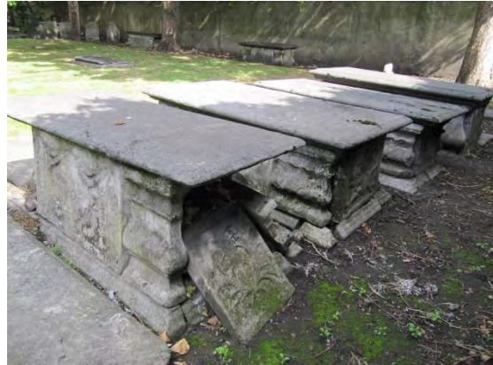
Damaged chest tombs; view left is the worst case, most have one or two collapsed panels
