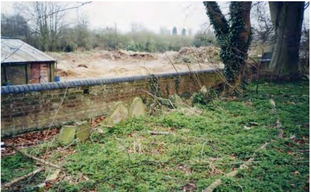
East boundary with cleared monuments next to former gas works (2000)
