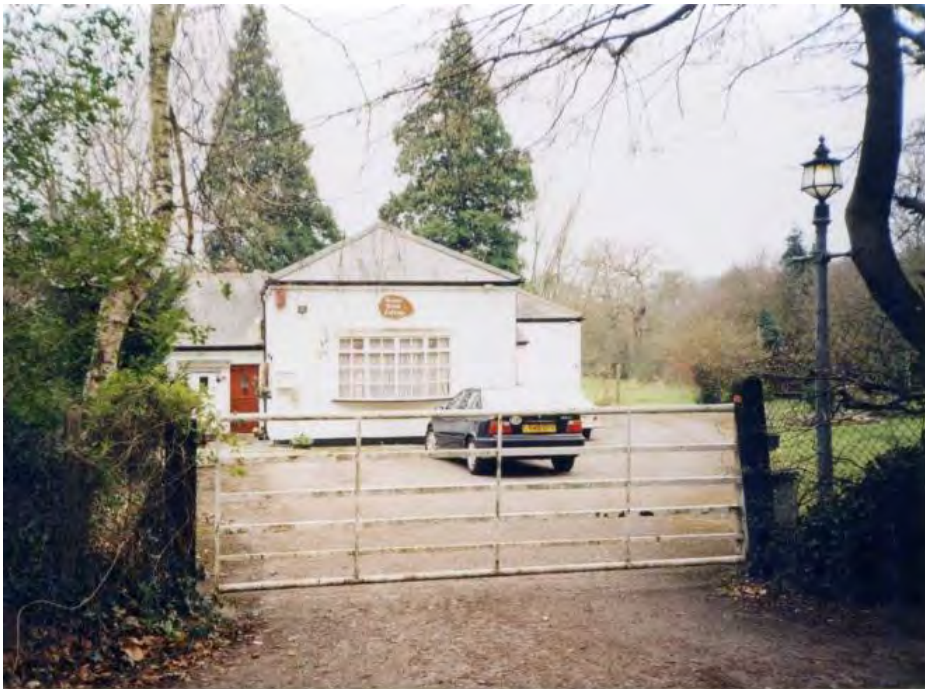
Former mortuary chapel seen from lane to north (2000) before extension.
