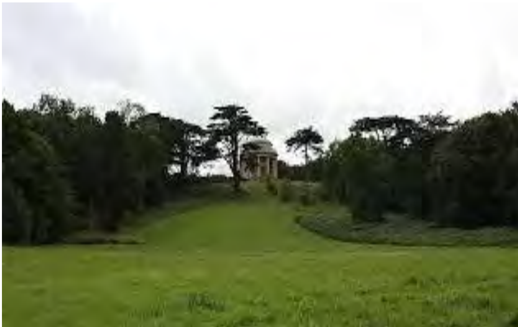
Setting from the north showing Cedar trees immediately around the building
