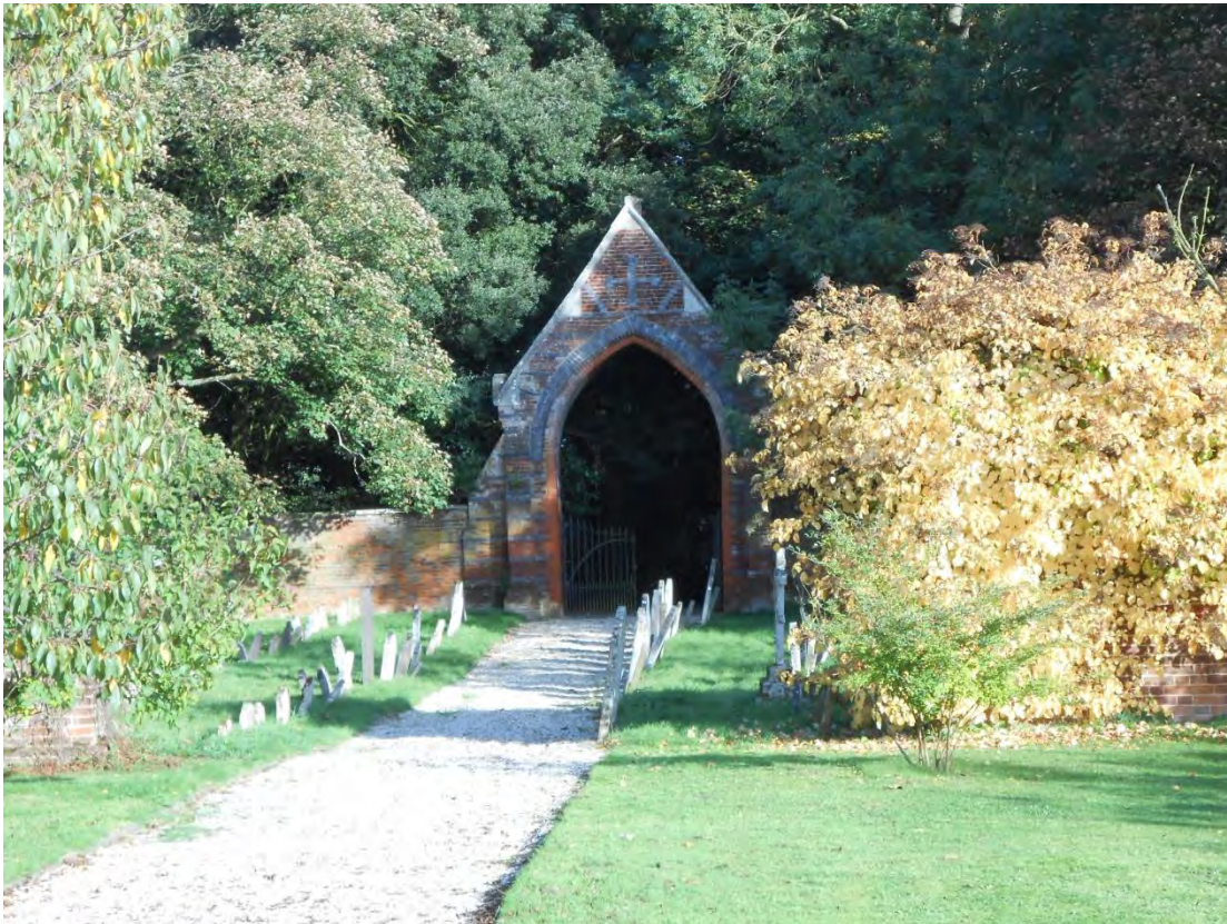
Interior of old section viewed from the newer extension. Access through boundary wall.
