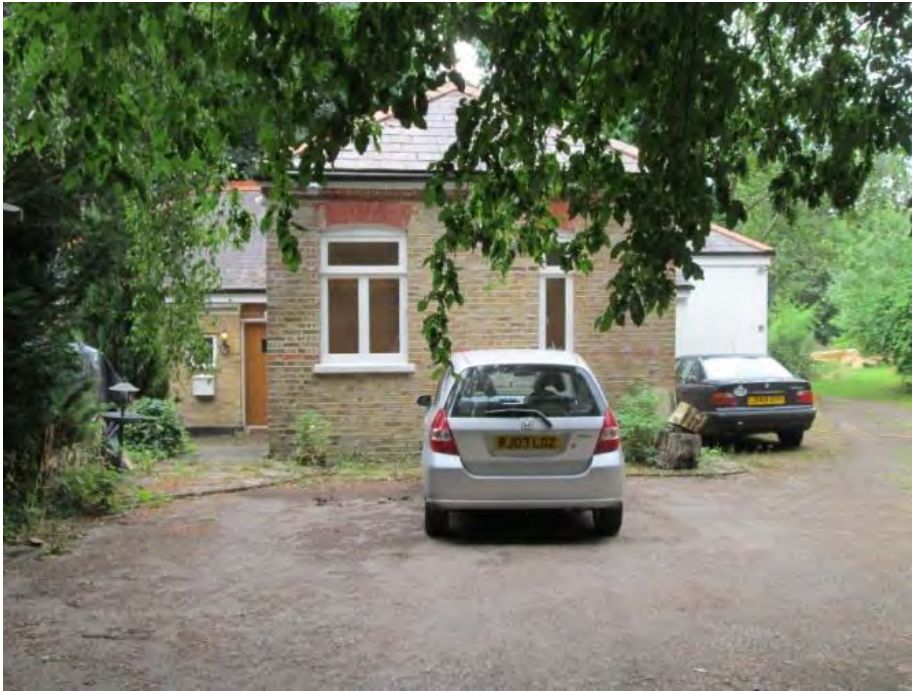
Former mortuary chapel seen from lane to north.
