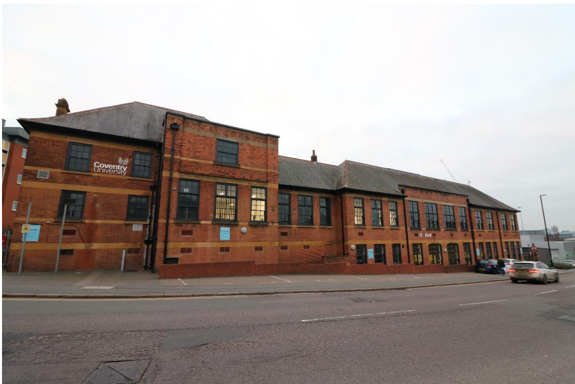
Fig 37: Cheylesmore Council School, Mile Lane. Photograph by authors
