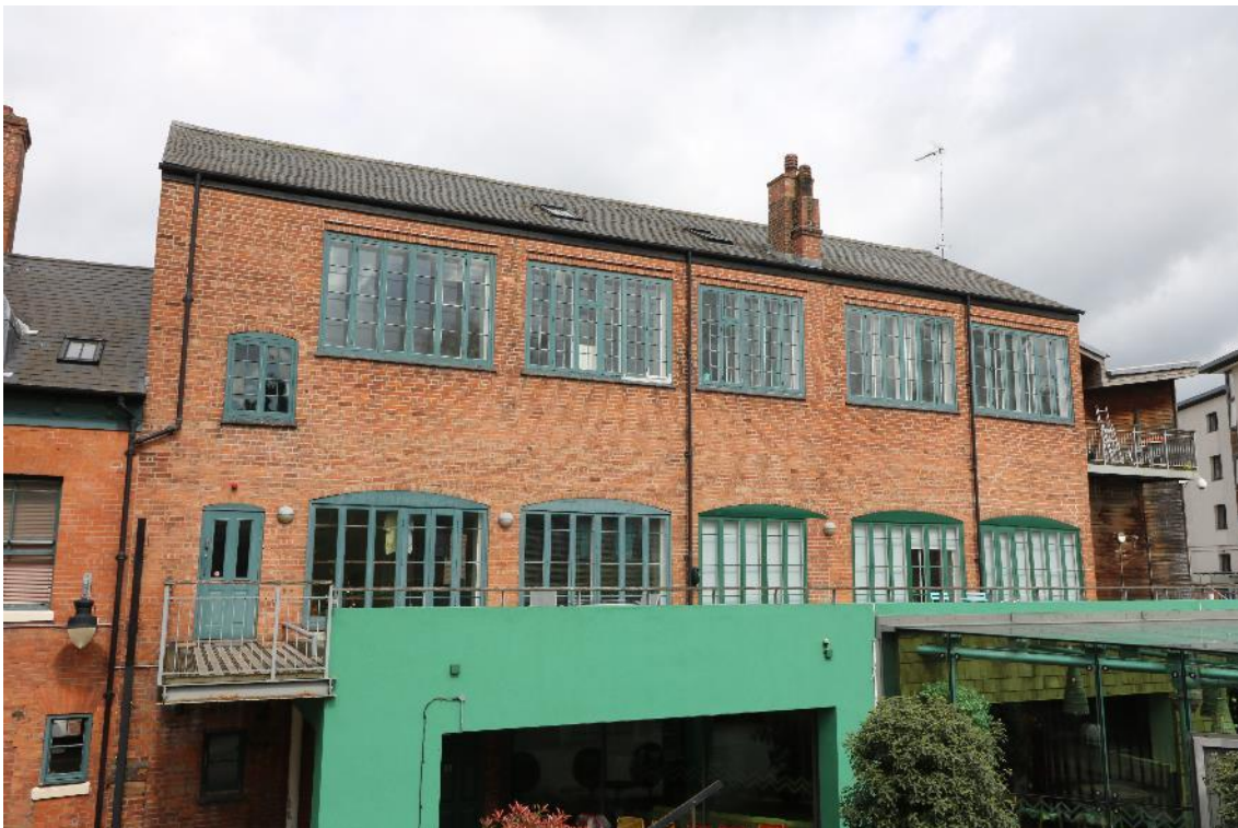
Fig 29: Former ribbon factory at 1-6 New Buildings. Photograph by authors
