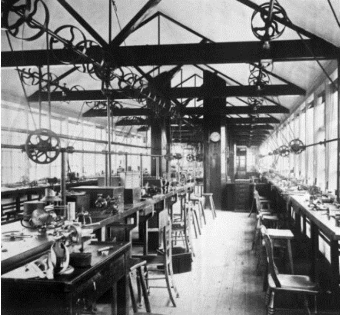
Fig 7: Rotherham's Watch Factory within a 'top-shop', 1890. Historic England (BL09921)
