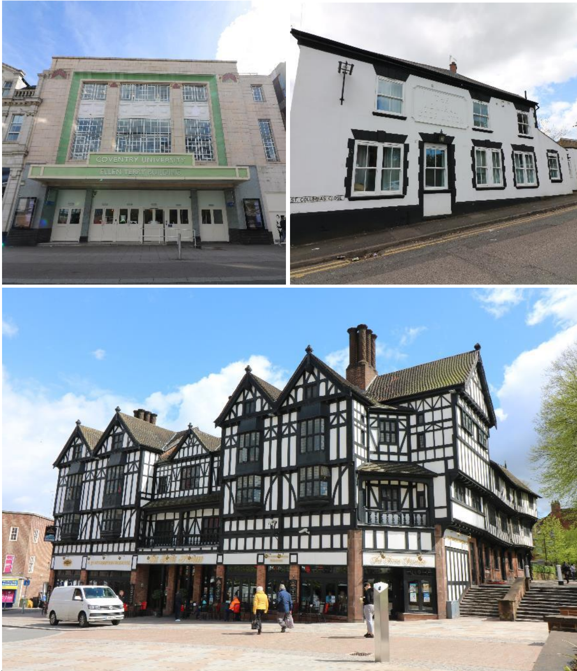
Fig 32: Ellen Terry Building, Jordan Well (top left); The Admiral Codrington, St Columba's Close (top right); The Flying Standard (bottom). Photographs by authors
