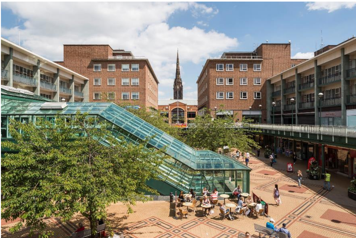
Fig 78: The Beaux-Arts inspired axial layout of the commercial precinct creates a number of distinctive views. Most striking is the view of the spire of St Michael's Cathedral, onto which the Upper Precinct was intentionally orientated by its architects (bottom). Later, the later 'terminating blocks' were also aligned to the axis, for instance Mercia House sited to the west and visible when looking down the precincts' east/west route between Broadgate and Lower Precinct (top). Historic England (DPI64313; DPI64623)
