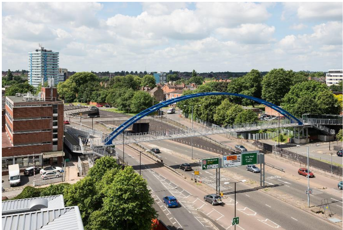
Fig 79: The city centre with its 'concrete collar'. Aerial view from the southeast (top). The 'Hill Cross' section of the ring road (bottom). Historic England (33181_013; DPI64733)
