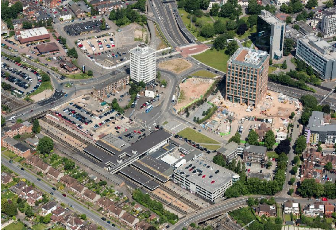
Fig 85: Aerial view of Coventry Station from the southeast. Historic England (33181_021).
