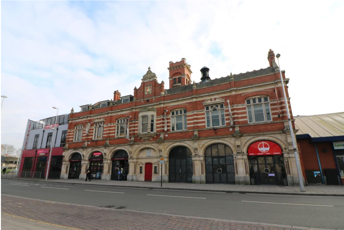
Fig 36: The Old Fire Station, Hales Street. Photograph by authors
