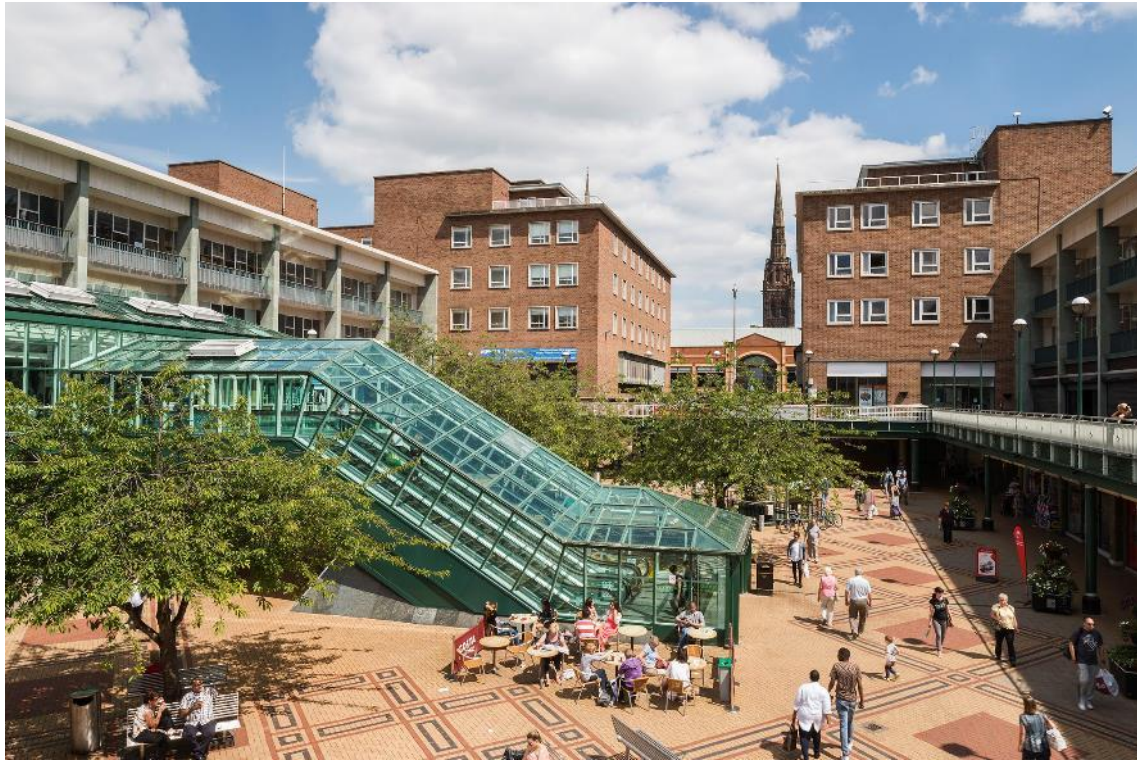
Fig 40: The Upper Precinct, looking east from the southwest corner prior to 2018-19 redevelopment. Historic England (DPI64624)
