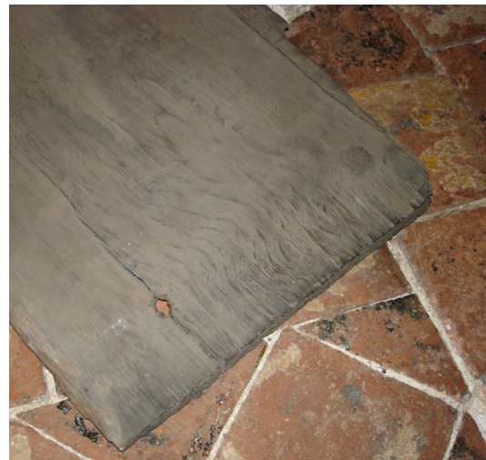
Figure 18: Scratched assembly marks and nail heads to shelf or canopy boards, Pyx Chamber (D Miles)
