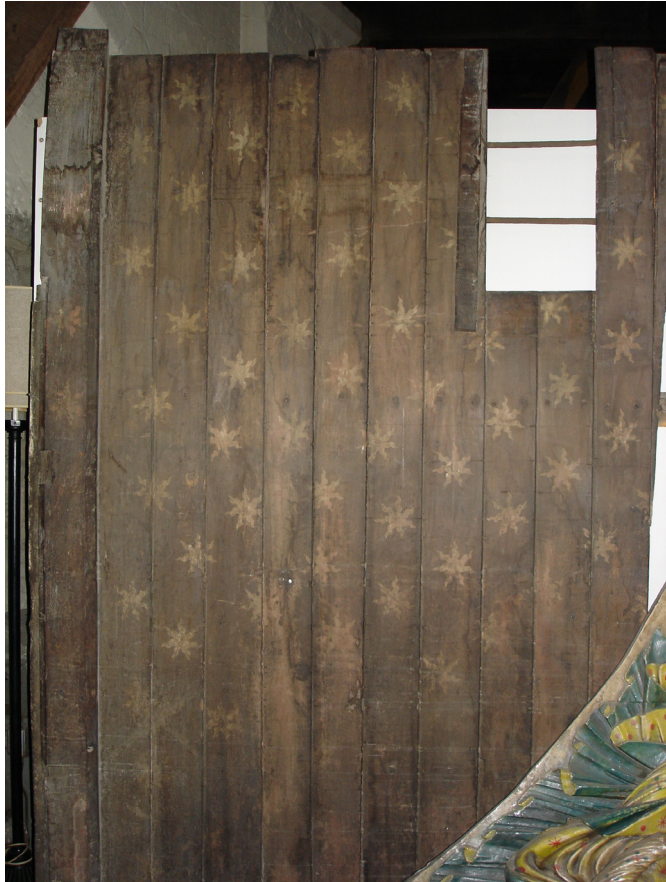
Figure 43: Wall panel from Muniment Room, now in Lapidarium (photographer)
