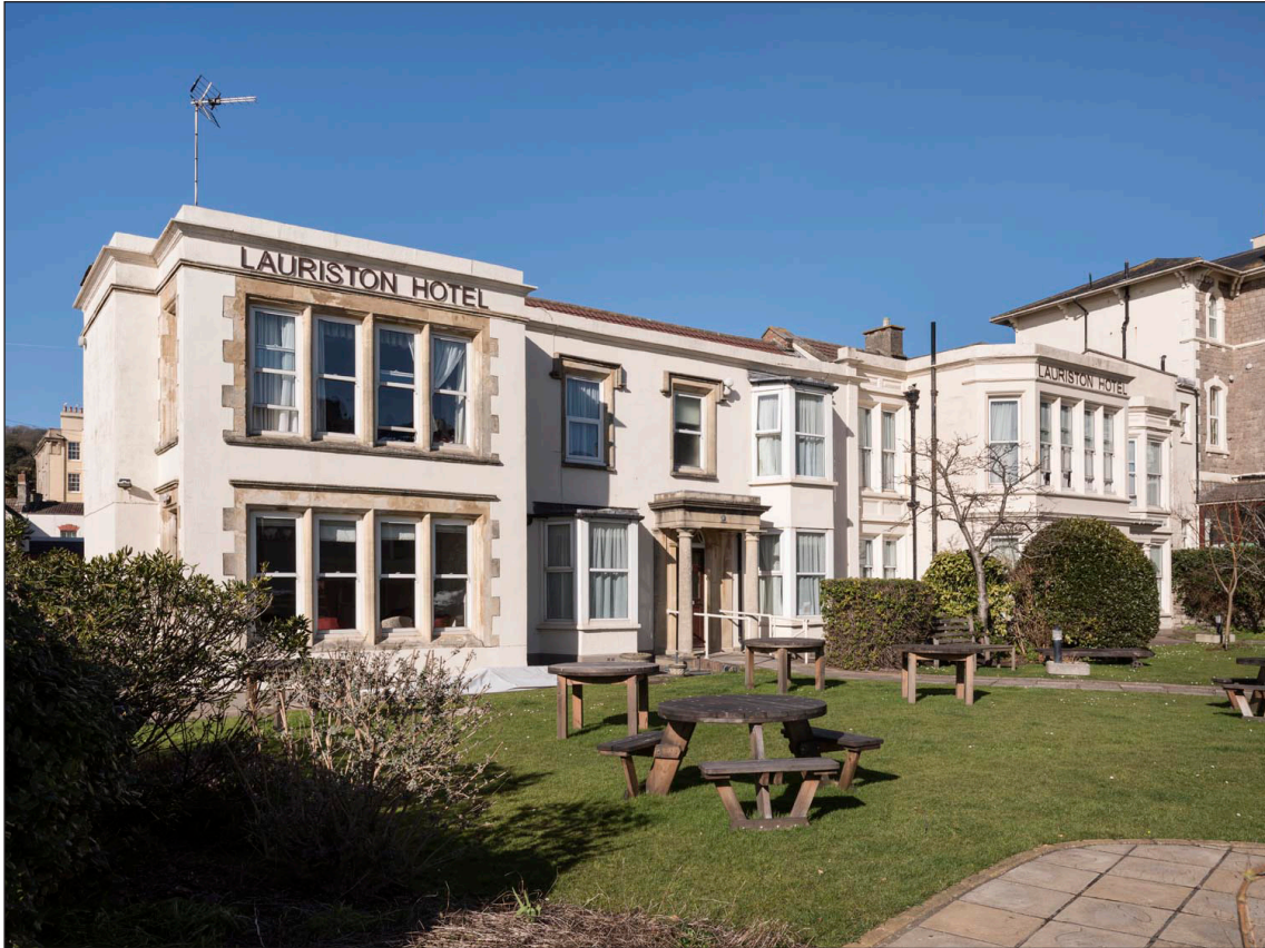
Figure 14: 1-2 Beachfield Villas are now part of the Lauriston Hotel, which was created through their amalgamation with the adjacent pair of Lauriston Villas. (DP218412)
