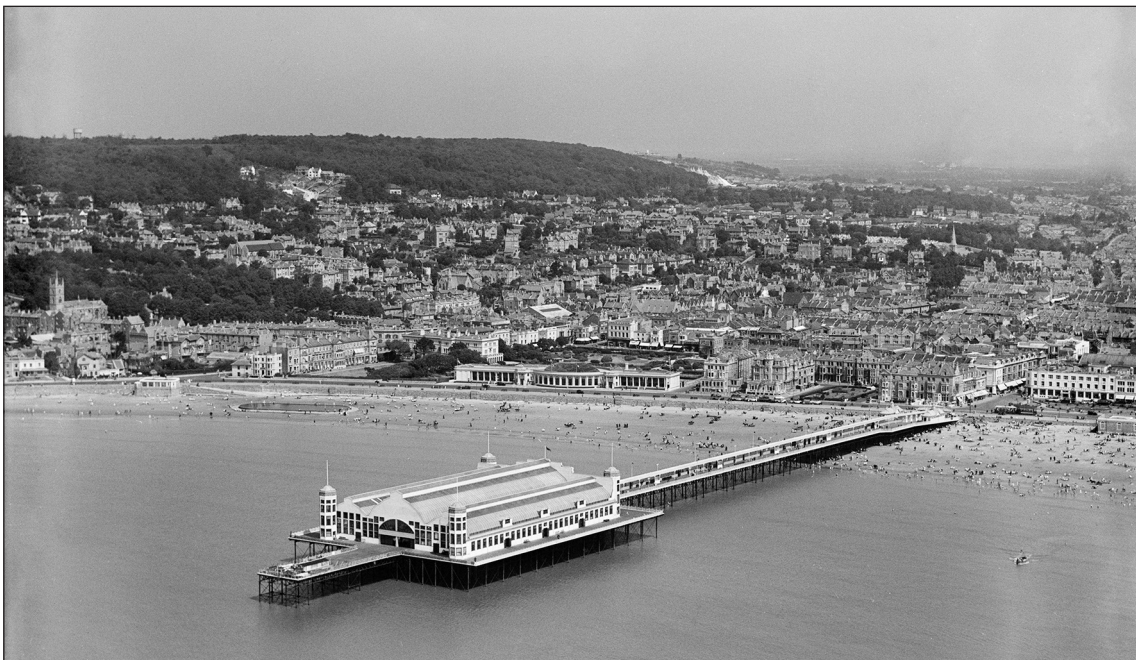
Figure 81: A 1935 Aerofilms photo of the Grand Pier once the pavilion had been rebuilt. (EPW048451)
