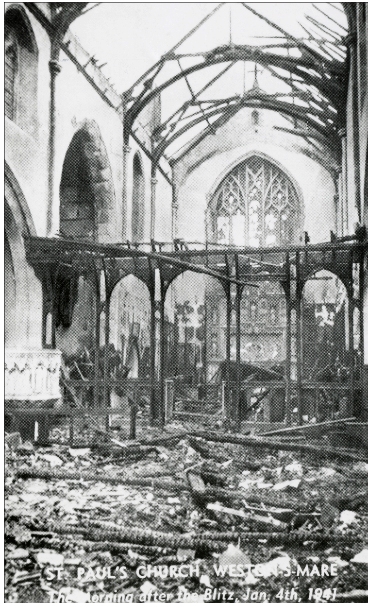
Figure 100: This photograph shows St Paul's Church after it had been hit during an air raid on 4 January 1941. (North Somerset Library Service)
