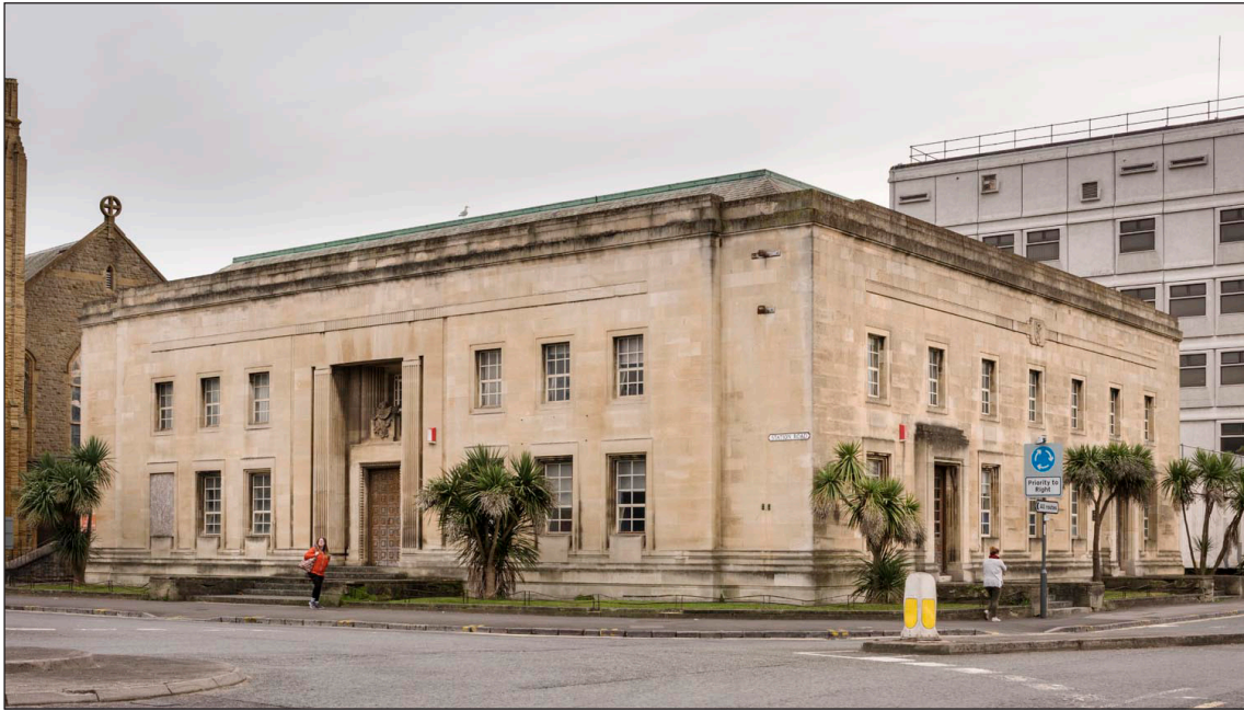
Figure 110: The 1934 Magistrates' Court will be retained and adapted to provide new homes in the centre of Weston, but the 1970 Police Station behind has been demolished to make way for housing. (DP218306)
