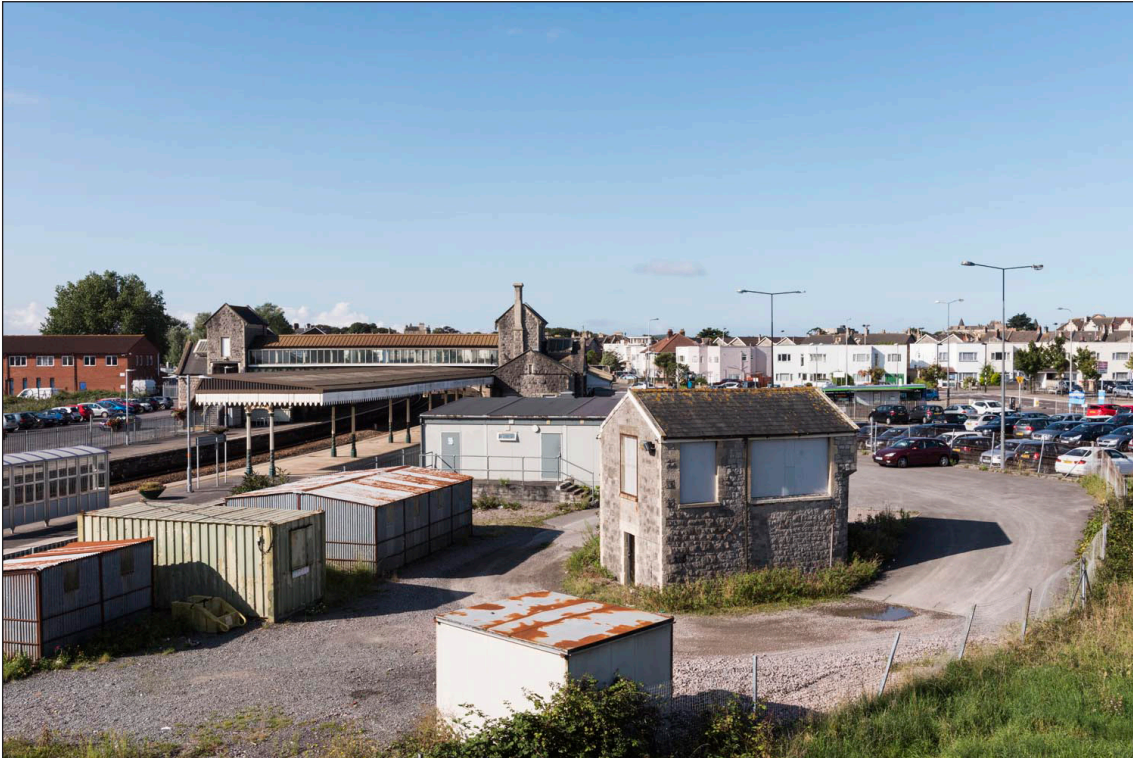
Figure 17: Coinciding with the new station, a new signal box for the branch line was constructed, though it now stands, unused, beside the current station. It is said to be the oldest surviving signal box on the British rail system. (DP218288)
