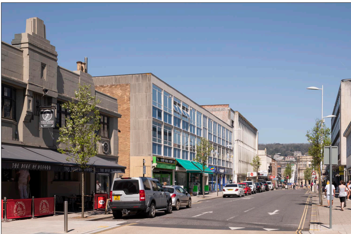
Figure 103: Union Street was widened during the 1950s when it became simply an extension of the High Street. The last surviving small houses on its east side were removed and new office buildings, shops and a new Friends Meeting House was created. (DP218536)
