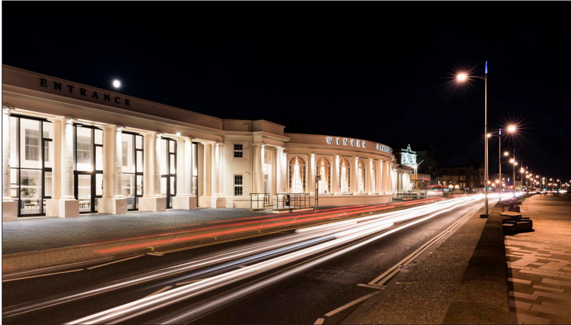
Figure 88: Designed by TH Mawson with the Borough Engineer Harold Brown, the Winter Gardens pavilion provided the town with a larger ballroom and it became home to HC Burgess's Orchestra. This modern, long time exposure image has the lights of cars streaking along the seafront road in front of it. (DP218335)
