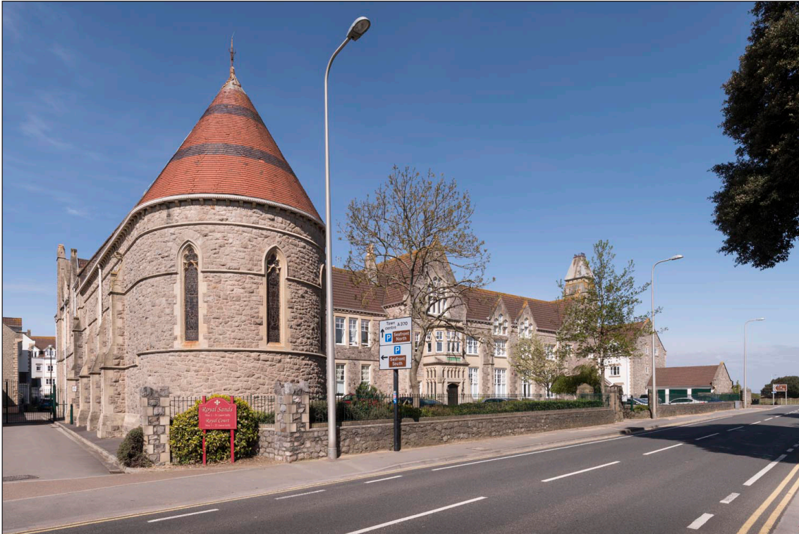
Figure 64: Around £14,000 was spent on the original Sanatorium, which would ultimately treat 100 patients. It was designed by Hans Price. Today the building has been converted into private apartments under the name of Royal Sands. (DP218567)
