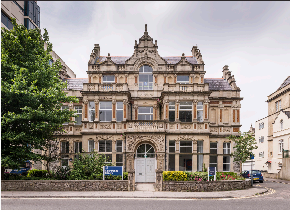
Figure 28: The high costs of carvings and other decorations meant that the fine street elevation of the School of Science and Art could only be added seven years after the main building had been completed. (DP218737)
