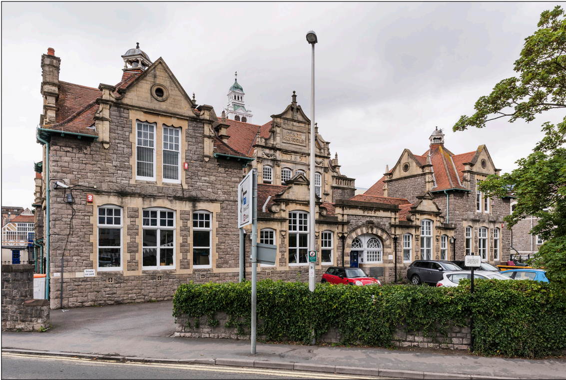
Figure 55: The Board School in Walliscote Road with its dramatic roofscape is one of Hans Price's best-known buildings and one of his most elaborately decorated. (DP218258)
