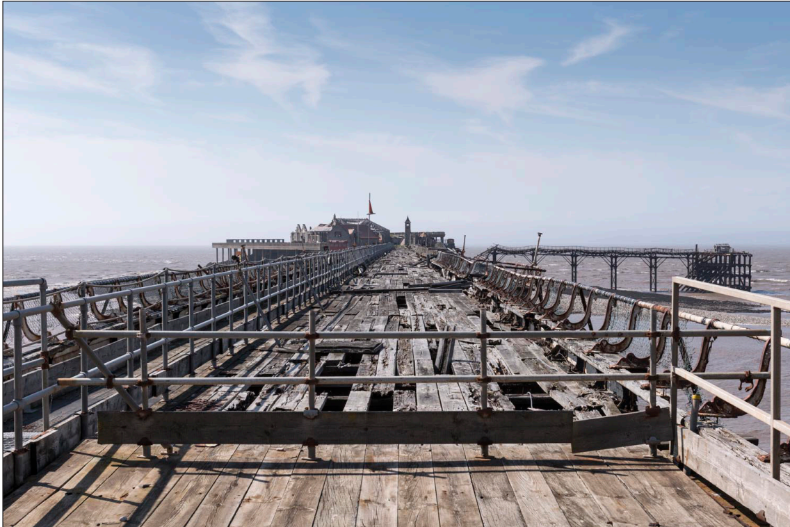
Figure 114: Birnbeck Pier looking towards the island (DP218733)
