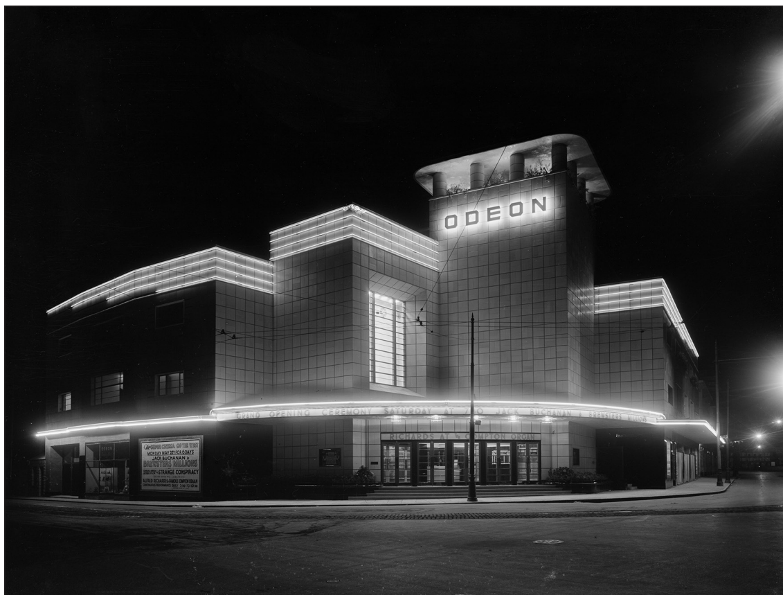
Figure 93: Howitt was responsible for designing four other Odeon cinemas: Warley, near Birmingham (1934); Clacton (1936, demolished); Bridgwater (1936); and Bristol (1938). All of his Odeon cinemas featured a square tower with a projecting flat slab roof supported by squat, cylindrical columns. (BB87/02801)
