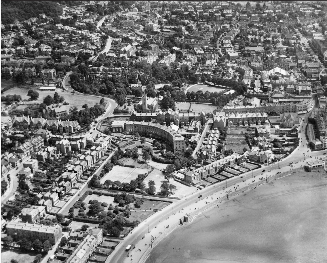
Figure 22: This Aerofilms photograph of 1930, taken from the east, shows Royal Crescent, with Oriel Terrace behind. Both were built in 1847 to a design by James Wilson of Bath for the solicitor Henry Davies (EPW033277)
