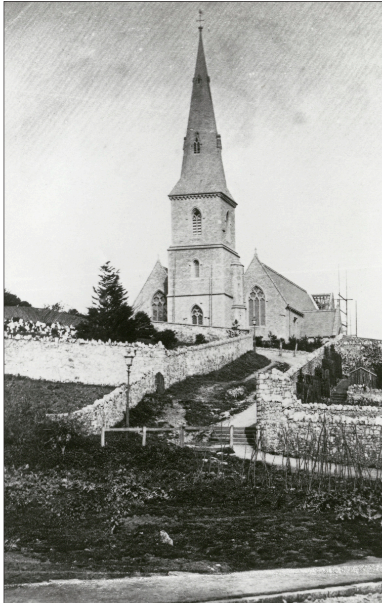
Figure 42: Christ Church of 1854-5 was one of the first buildings in the new district of Montpelier. This photograph was taken in around 1877, when the chancel extension by Price & Grosholz was under construction, with scaffolding visible at the right-hand side of the photograph. (North Somerset Library Service)
