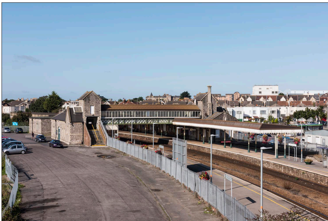
Figure 19: Weston's current railway station is actually relatively small, with only two platforms flanking the twin tracks. (DP218284)
