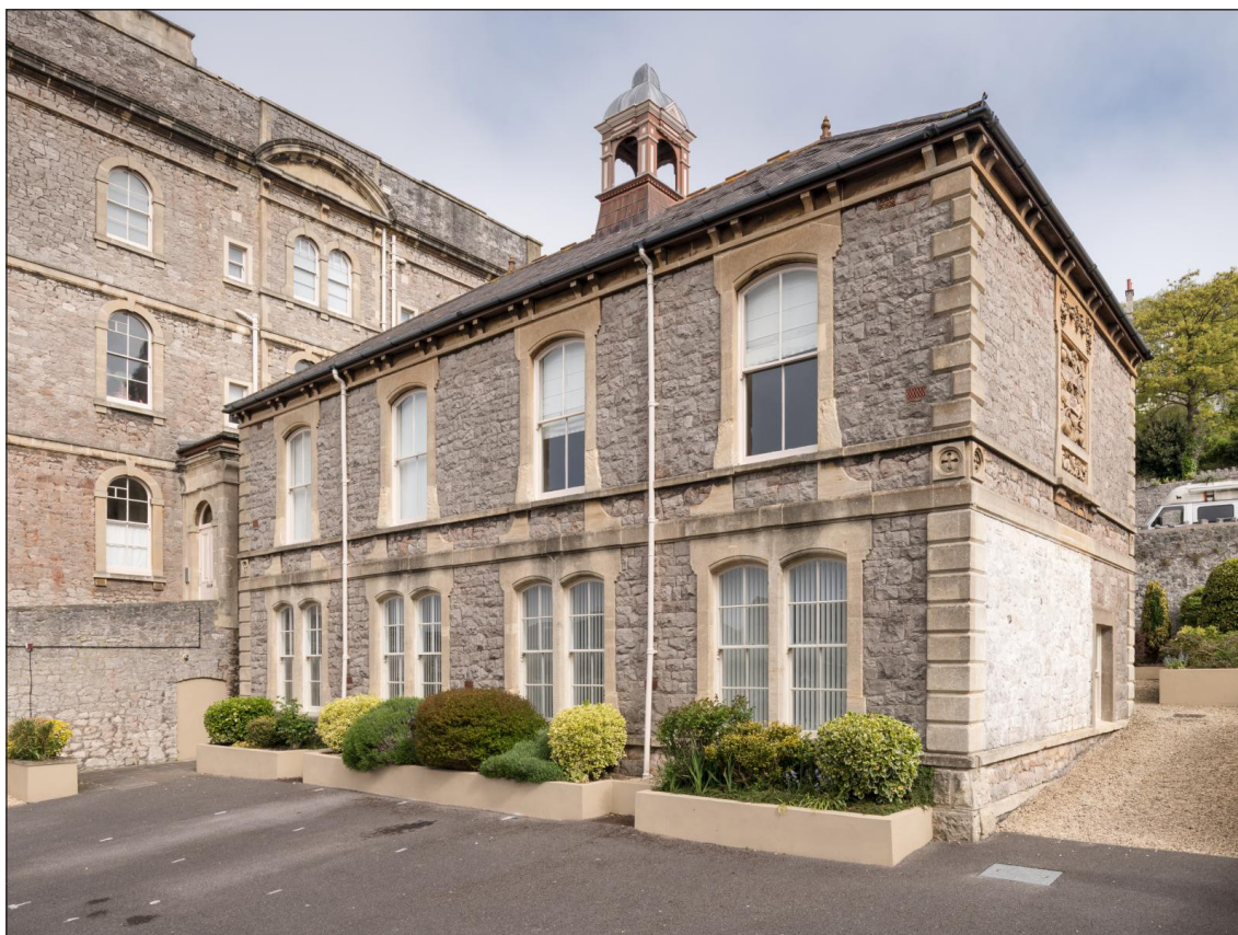
Figure 57: The extension to St Peter's Preparatory School in Atlantic Terrace East by Price & Wooler. (DP218643)
