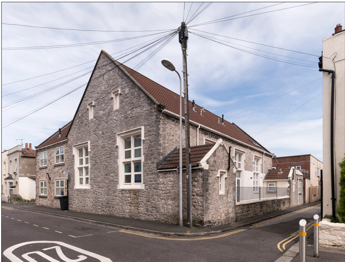
Figure 54: After its opening in 1855, the British School was described by the Taunton Courier and Western Advertiser as a 'handsome, lofty, and well-ventilated building'. (DP218581)
