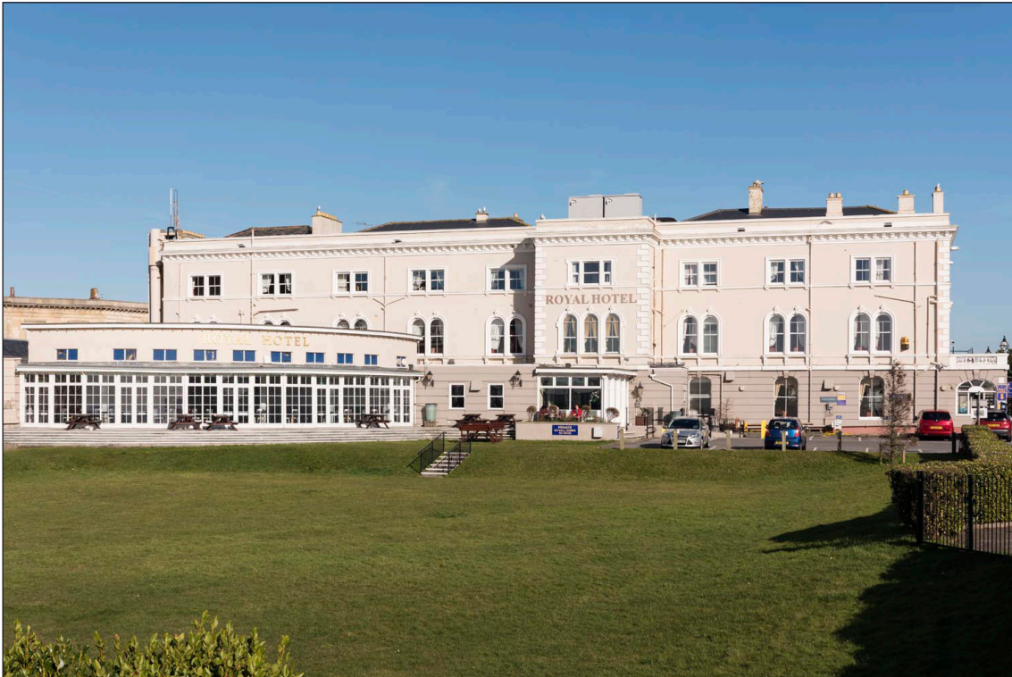
Figure 7: Early maps show the Royal Hotel to have been a much smaller building, which matches the southern three bays of the hotel (right-hand side). The end of the original building appears to have been where the almost central block breaks forward. (DP218422)
