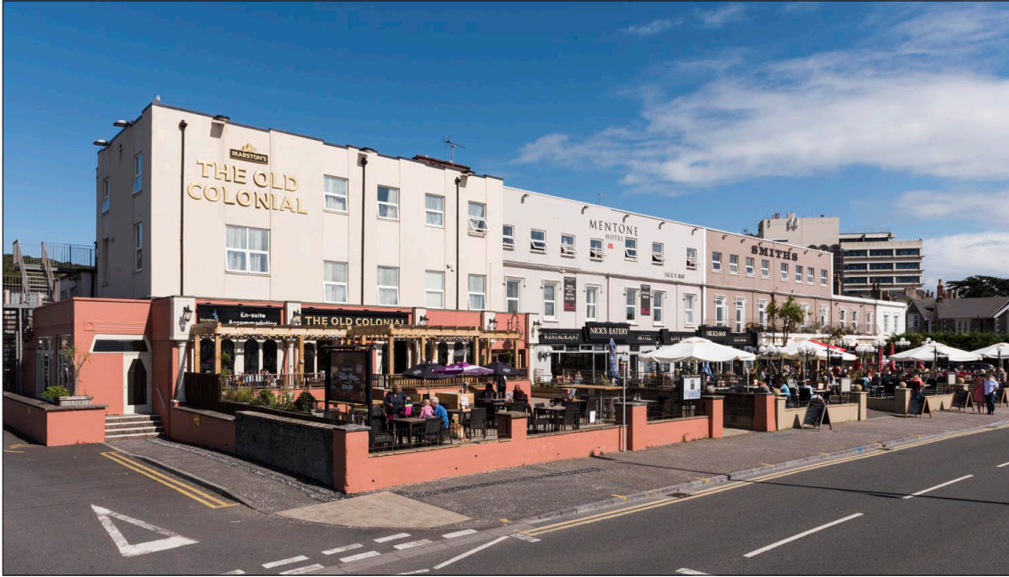
Figure 15: Victoria Buildings was the first terrace built on the seafront. Although it was originally constructed for wealthy residents, its houses were soon being used as lodgings for affluent holidaymakers. This photograph shows that most of the terrace has been raised by one storey. (DP218275)
