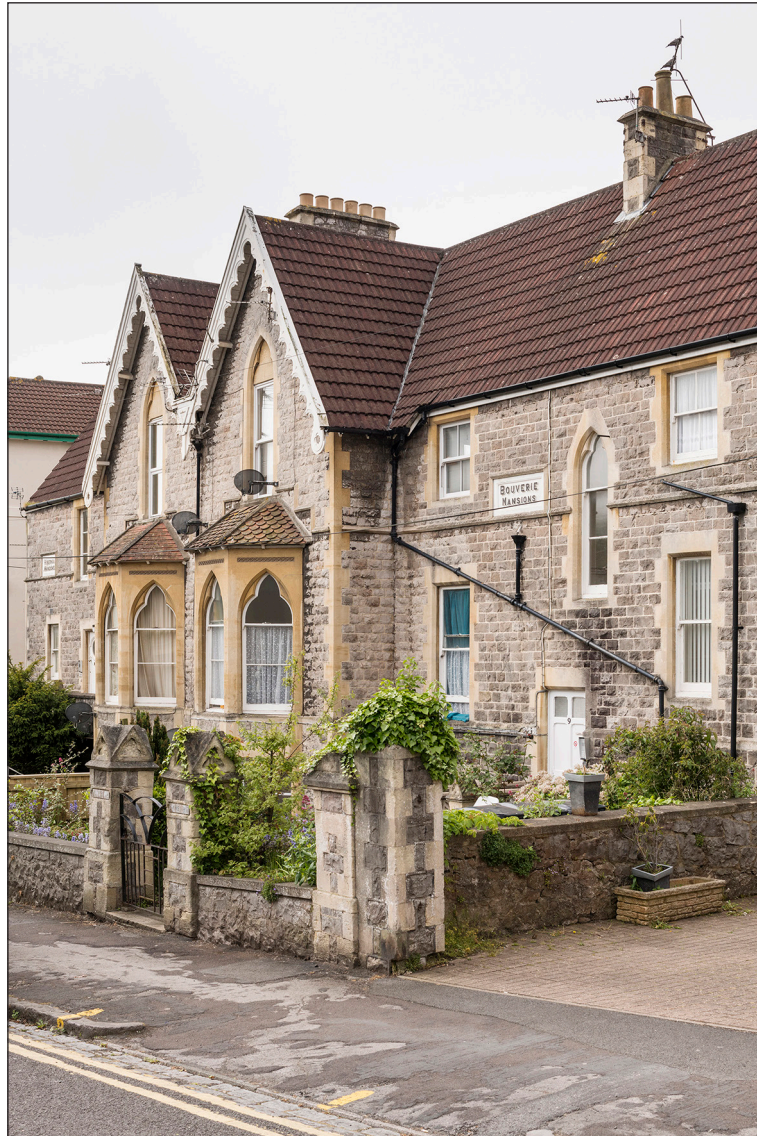
Figure 96: This pair in Victoria Quadrant was among many Victorian houses acquired by Henry Butt and converted into flats during the interwar period. It is now known as Bouverie Mansions (right-hand side) and Hibernia Mansions (left-hand side). (DP218645)
