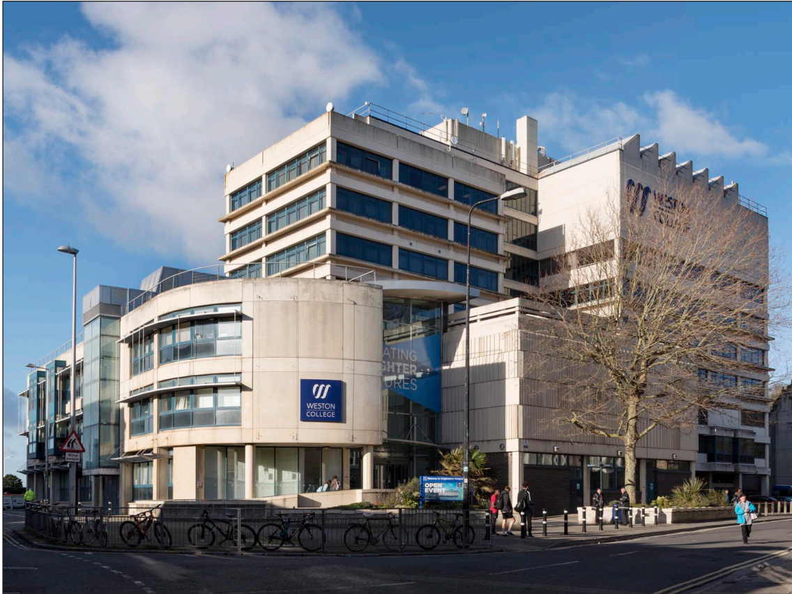
Figure 105: The eight-storey Weston College was designed by Bernard Adams, the County Architect; it was enlarged and updated in 1997-8 by Stride Treglown. (DP218342)
