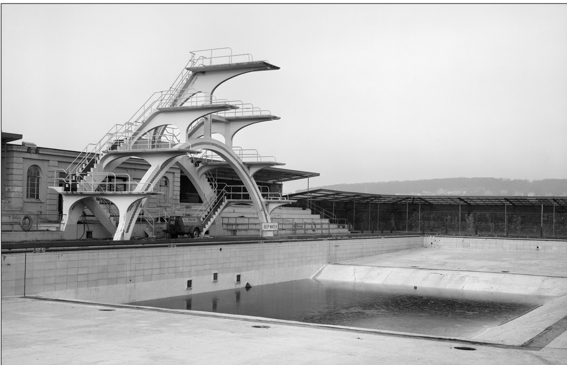
Figure 91: The structure consisted of two parallel reinforced concrete arches, 26ft (8m) high, faced with a band of coloured tiles from which seven boards at 3m, 5m, 7m and 10m were cantilevered. These were reached by steps from the rear. This photograph was taken to mark its completion in 1937. (BB81/08493)
