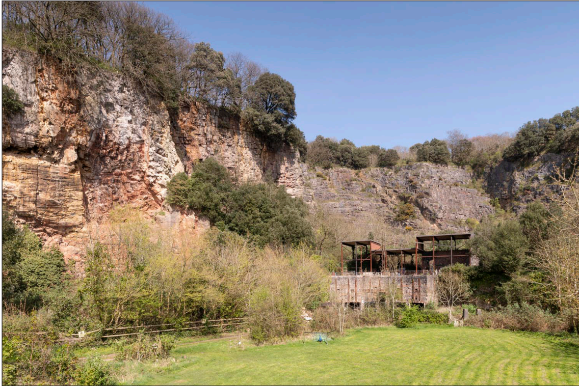
Figure 69: The Town Quarry and another at Milton were the main sources of local stone used in Weston's housing boom from the mid-19th century onwards, along with stone imported from around Bath for dressings and fine detailing. (DP218544)
