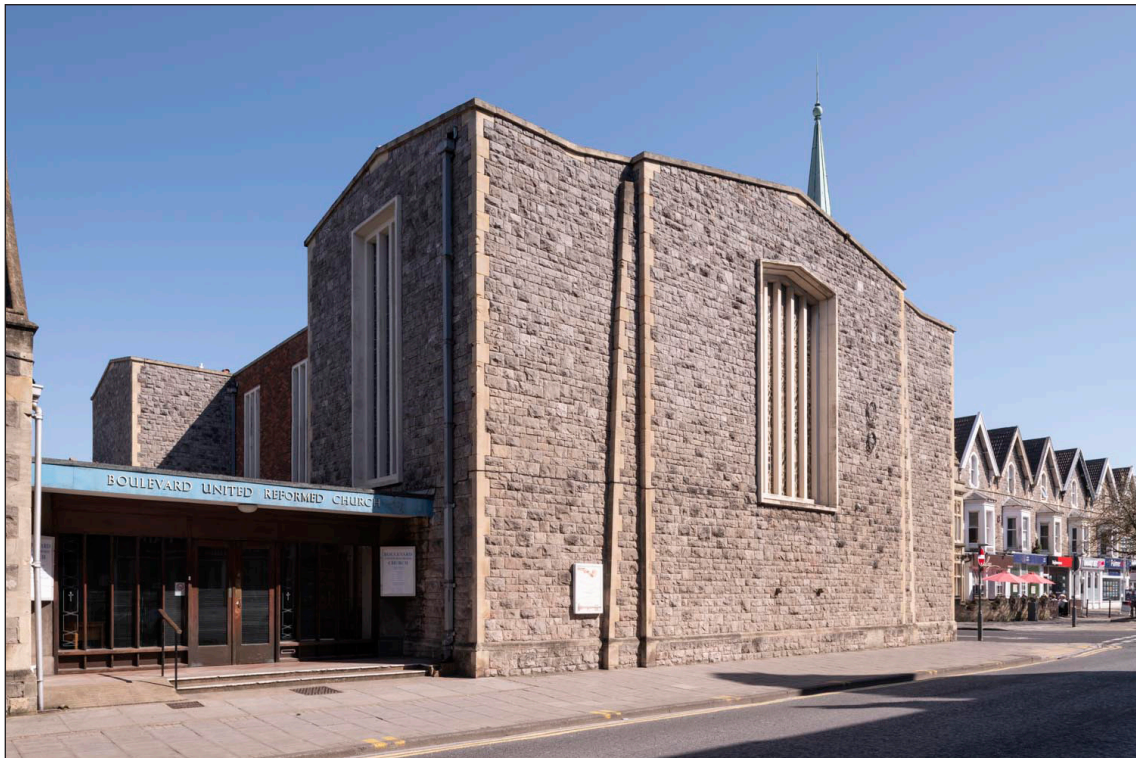
Figure 102: The Boulevard Congregational Chapel (now the Boulevard United Reform Church) was rebuilt and reopened in 1959 to designs by Gordon W Jackson & Partners. The adjacent church hall was rebuilt in 1953, another victim of the highly damaging air raid of 28-29 June 1942. (DP218516)
