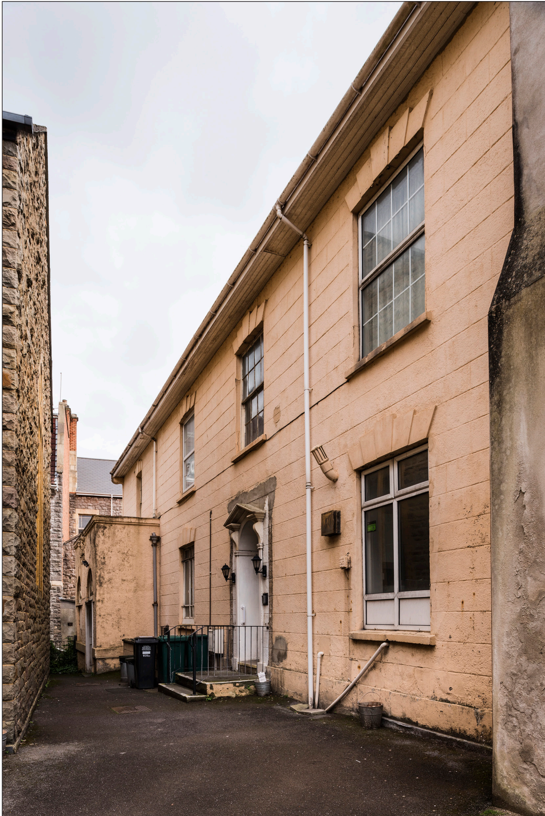
Figure 8: Originally three-bays wide and symmetrical, a fourth bay in a similar style was added to the east of Parsley's Whitecross House between 1903 and 1931, by which time the building was being used as a Sunday School. (DP218260)
