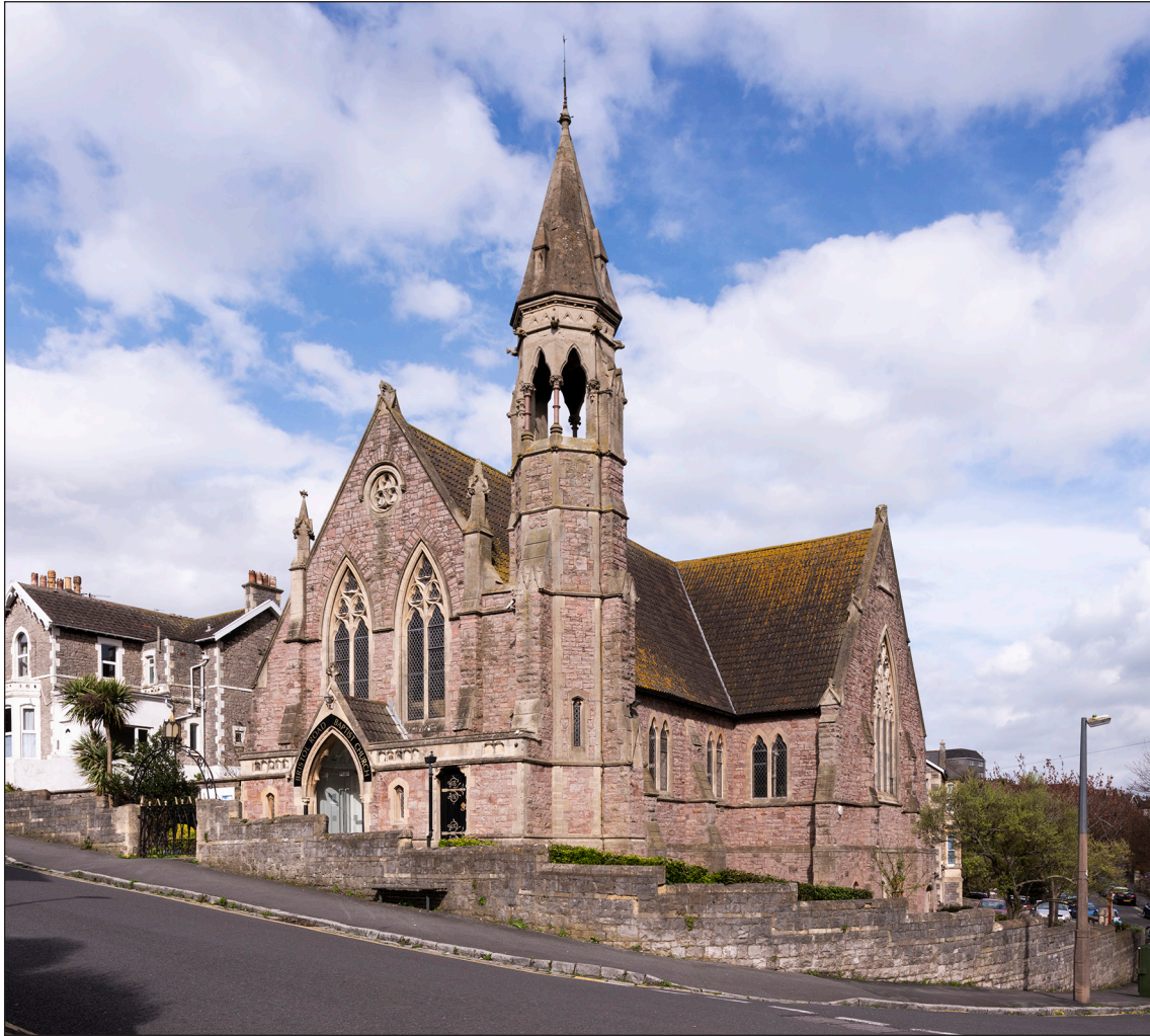
Figure 51: The Baptist Chapel in Bristol Road Lower was built in 1865-5 to a design by Hans Price. (DP218508)
