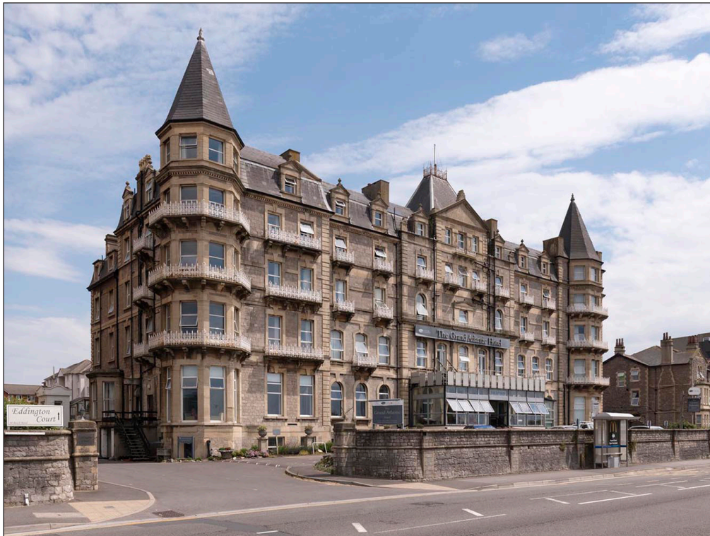
Figure 84: Examination of the Grand Atlantic's facade reveals that the original elevation of the College survives, but the building has been extended on either side by wings with polygonal, corner turrets. It has also been raised to four storeys, with an attic throughout. (DP218759)
