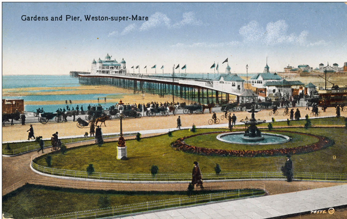
Figure 79: The Grand Pier's original pavilion was destroyed by fire in 1930 and its replacement also succumbed to fire in 2008. This early 20th century postcard also shows the seafront tram, a number of horse-drawn carriages and some early motor cars. (PC08229)
