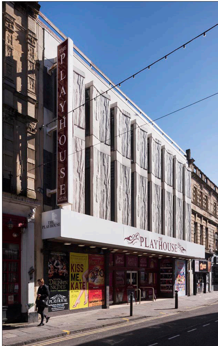
Figure 104: The new Playhouse, which opened in 1969, was designed by WS Hattrell & Partners and has a brutalist facade with boxed-out panels of textured glass fibre, sculpted by William Mitchell. (DP218395)
