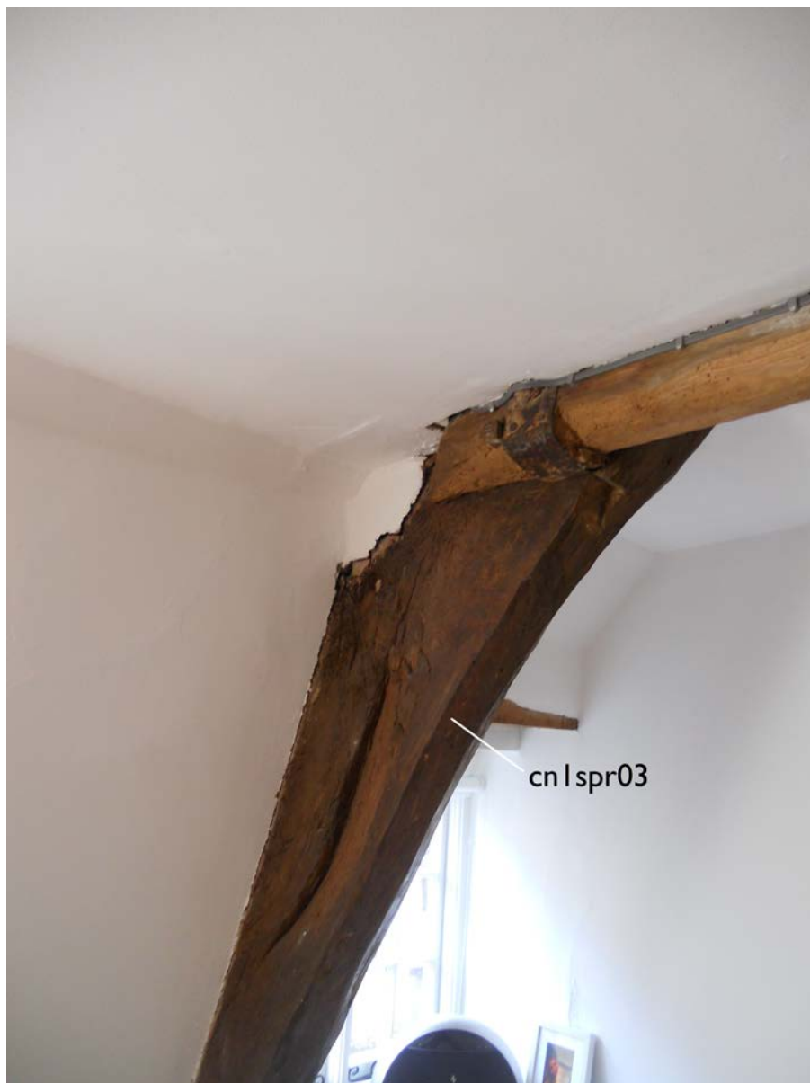
Figure 6: Photograph showing the west principal rafter of the south truss sampled for dendrochronology (photograph Martin Bridge)
