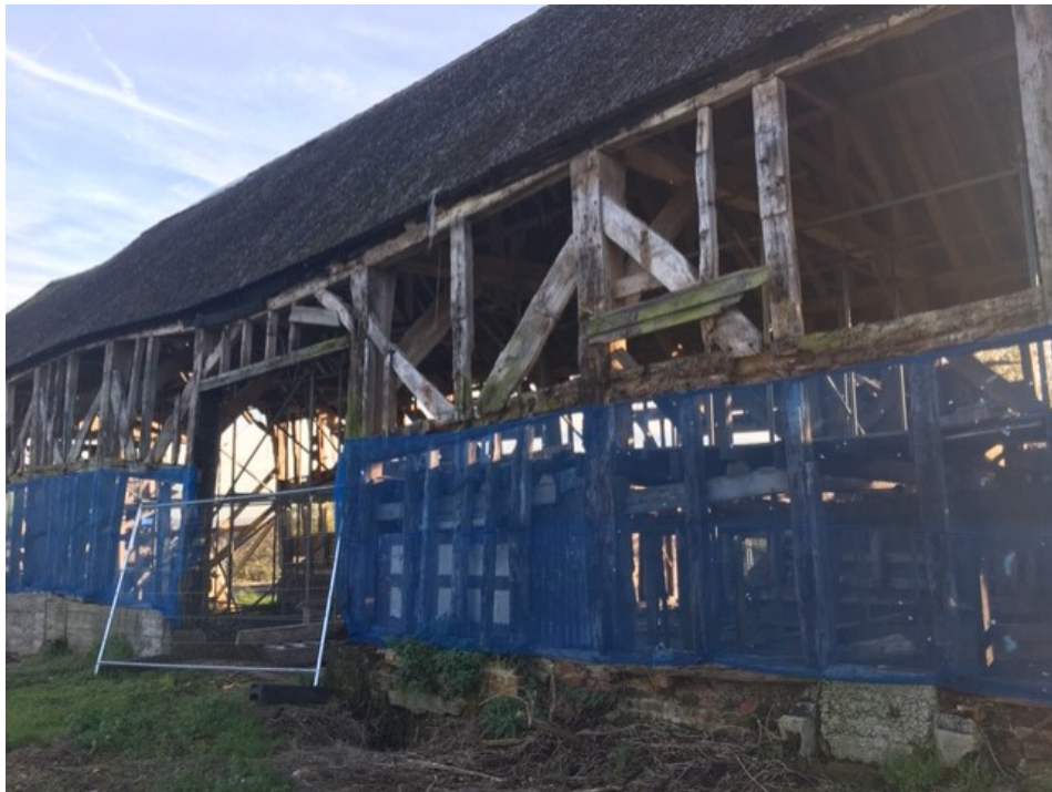
Figure 4: North wall of the barn with its unusual bracing, photograph taken from the north-east (photograph Alison Arnold)
