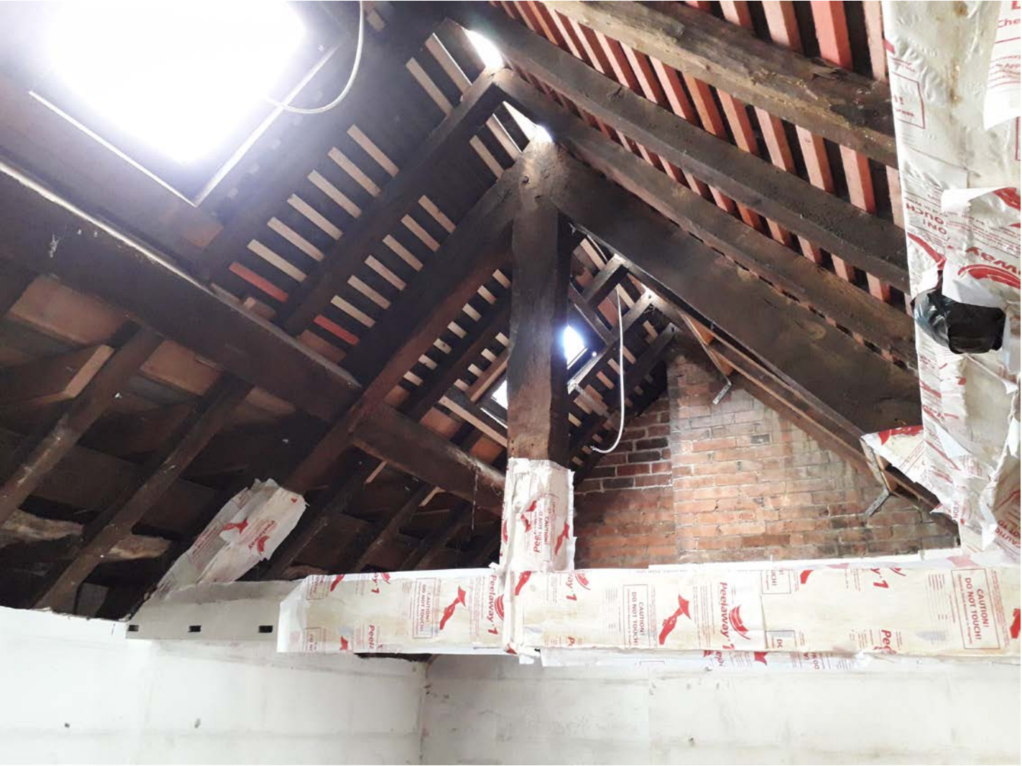
Figure 2: North side, truss 4, photograph taken from the south (Alison Arnold)
