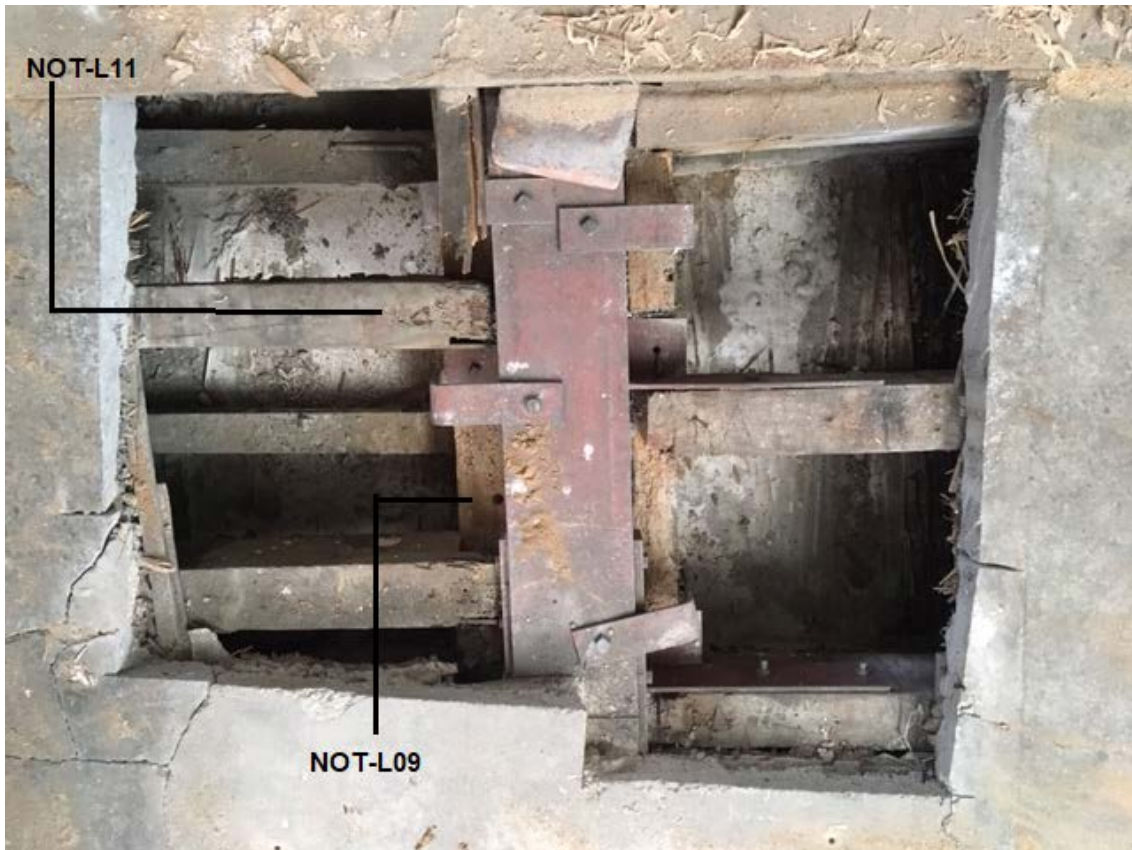
Figure 4: Photograph of some of the exposed floor frame on the north side, showing the location of samples NOT-L09 and NOT-L11, photograph taken from the north (Alison Arnold)
