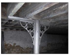
Figure 53: The centrally located iron column in R003 (© Historic England, photograph: Alastair Coey Architects, 2019)
