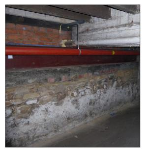
Figure 68: The north side of the blocked up opening between R001 and 002 with steel I-beam inserted above original wall (© Historic England, photograph: Alastair Coey Architects, 2019)
