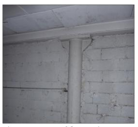
Figure 124: One of the cast-iron columns in the south wall of R118 carrying a steel beam (© Historic England, photograph: Alastair Coey Architects, 2019)
