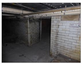
Figure 87: Opening leading into R003 showing glazed brick walling and sections of timber staging (© Historic England, photograph: Alastair Coey Architects, 2019)
