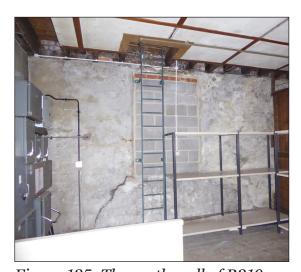
Figure 125: The south wall of R210 showing the blocked window, steel ladder and electrical distribution boards to left (© Historic England, photograph: Alastair Coey Architects, 2019)
