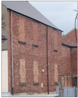
Figure 118: The south wall elevation of Block E showing blocked windows (© Historic England, photograph: Alastair Coey Architects, 2019)
