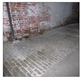
Figure 28: Floor covering of wooden blockers in R141 (© Historic England, photograph: Alastair Coey Architects, 2019)
