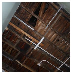
Figure 151: The exposed timber structure of the ceiling of R323 forming a floor in the next stage of the water tower above (© Historic England, photograph: Alastair Coey Architects, 2019)
