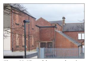
Figure 82: View of the west elevation of the 1892-94 building showing the windows of the 'Waiting Room' (centre) and blocked south windows of the 'Manager's Office' (to their left). Both rooms now form part of R208 (© Historic England, photograph: Alastair Coey Architects, 2019)
