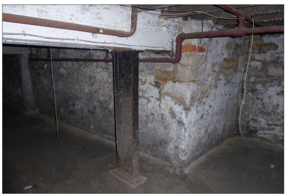
Figure 70: Steel stanchion carrying the north end of the east beam in the ceiling of R001 (© Historic England, photograph: Alastair Coey Architects, 2019)
