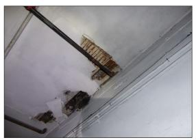
Figure 93: The original lath and plaster ceiling in the 'gateway' (R113) (© Historic England, photograph: Alastair Coey Architects, 2019)
