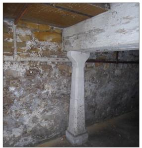
Figure 69: Timber post carrying the north end of the central beam in the ceiling of R001 (© Historic England, photograph: Alastair Coey Architects, 2019)
