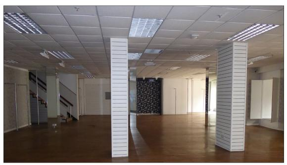
Figure 18: Columns with later facings at the division between the 1873 and 1882-83 blocks (© Historic England, photograph: Alastair Coey Architects, 2019)
