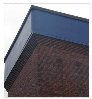
Figure 129: View of the water tower storage tank from the northwest showing the tank panels and corbel-course (© Historic England, photograph: Alastair Coey Architects, 2019)
