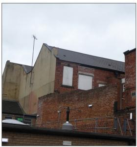
Figure 63: The rendered north end elevation of the 1882-83 building and part of the warehouse of Block F (© Historic England, photograph: Alastair Coeu Architects, 2019)
