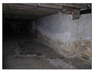
Figure 51: Limeswashed rubble construction in the north wall of R003 (© Historic England, photograph: Alastair Coey Architects, 2019)
