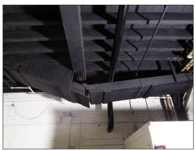
Figure 156: A timber chute in the ceiling of R119 (© Historic England, photograph: Alastair Coey Architects, 2019)
