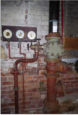
Figure 36: Pipework and dials associated with the Mather and Platt sprinkler systems (© Historic England, photograph: Alastair Coey Architects, 2019)
