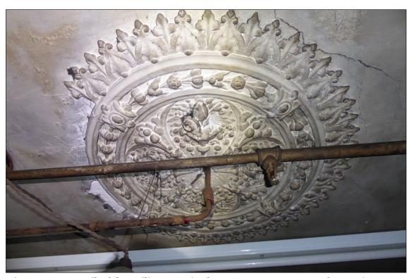
Figure 142: Detail of the ceiling rose in the west compartment of R132 (© Historic England, photograph: Alastair Coey Architects, 2019)
