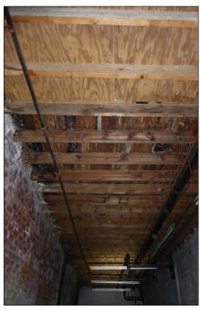
Figure 160: Timber ceiling joists and boards in R141-142 looking east (© Historic England, photograph: Alastair Coey Architects, 2019)
