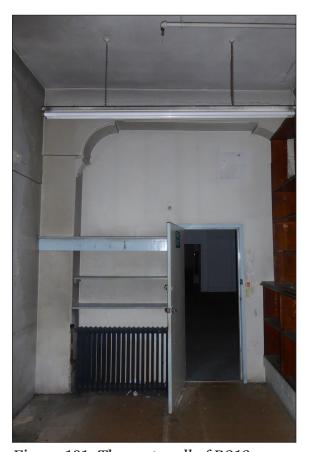
Figure 101: The east wall of R213 showing the shouldered-arch opening into R208 (© Historic England, photograph: Alastair Coey Architects, 2019)
