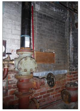
Figure 137: The east wall of R129 showing the blocked window to R132 and pipework relating to the 1908 Grinnell sprinkler system (© Historic England, photograph: Alastair Coey Architects, 2019)
