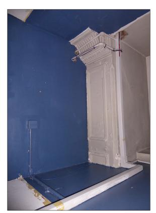
Figure 55: The remains of the panelled soffit in the reduced opening between R103 and R123 (© Historic England, photograph: Alastair Coey Architects, 2019)
