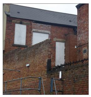
Figure 64: Blocked up second-floor window (left), opening onto former lift shaft (centre) and half-landing window (right) on the rear of the 1882-83 building (© Historic England, photograph: Alastair Coey Architects, 2019)
