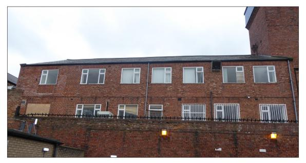
Figure 130: North elevation of the 1883 warehouse (Block F) with replacement casement windows (© Historic England, photograph: Alastair Coey Architects, 2019)
