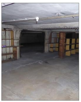
Figure 85: R004 looking north-west showing the two columns offset from the centreline (© Historic England, photograph: Alastair Coey Architects, 2019)
