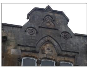
Figure 23: Detail of truncated central gable to 1892-94 section (© Historic England, photograph: Alastair Coey Architects, 2019)
