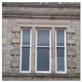
Figure 105: The central tripartite first-floor window on the 1894 building (Block D) (© Historic England, photograph: Alastair Coey Architects, 2019)
