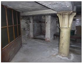
Figure 86: Detail of a column in R004 with timber staging behind (© Historic England, photograph: Alastair Coey Architects, 2019)
