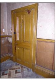
Figure 114: The door of R209 with bolection mouldings (© Historic England, photograph: Alastair Coey Architects, 2019)
