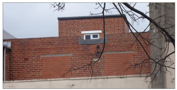
Figure 83: Blocked windows and parapet to the rear of R306 (© Historic England, photograph: Alastair Coey Architects, 2019)
