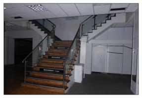
Figure 80: The modernised bifurcated staircase on the ground floor of R104 (© Historic England, photograph: Alastair Coey Architects, 2019)
