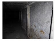
Figure 52: The inserted timber beam and posts on the south wall of R003 (© Historic England, photograph: Alastair Coey Architects, 2019)
