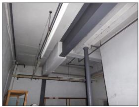
Figure 143: Interior of R133 looking south showing the column supporting the flitch beam and R131 partitioned off to the right (© Historic England, photograph: Alastair Coey Architects, 2019)
