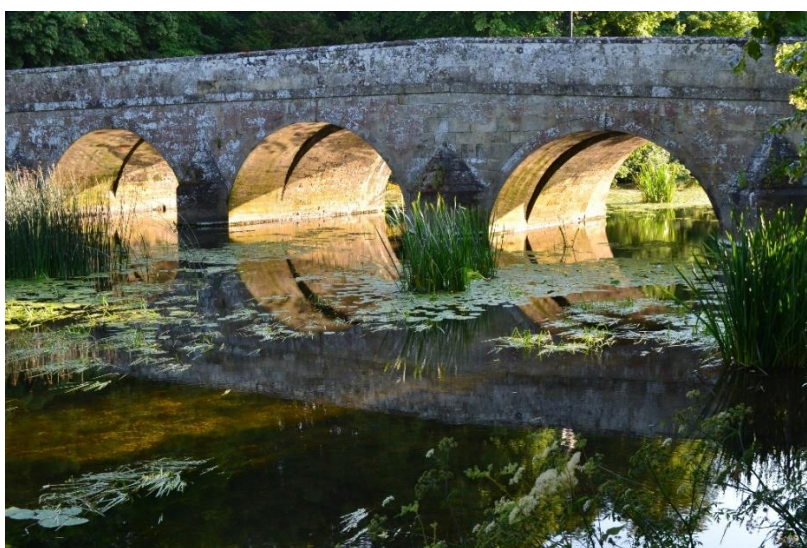
Figure 24 View of Blandford Bridge
