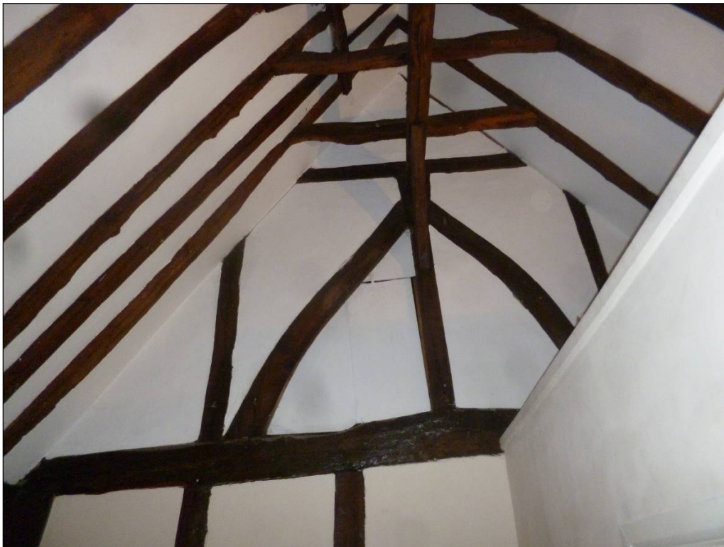
Figure 5: Truss III, photograph taken from the south (Robert Howard)
