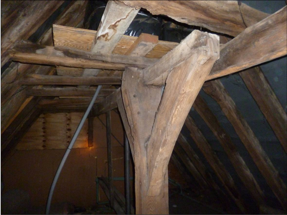
Figure 7: Truss IV, photograph taken from the north (Robert Howard)
