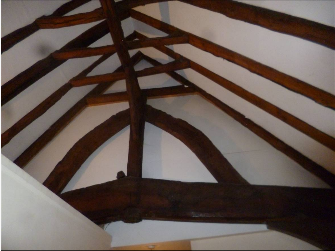
Figure 6: Truss III, photograph taken from the north (Robert Howard)
