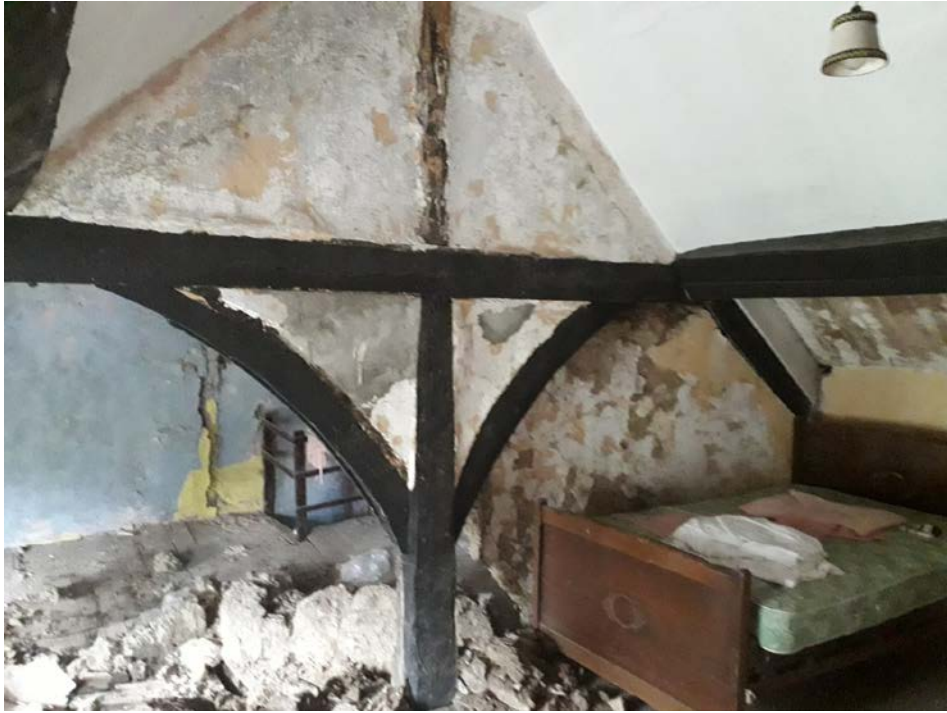
Figure 3: Truss 3, photograph taken from the east (Alison Arnold)
